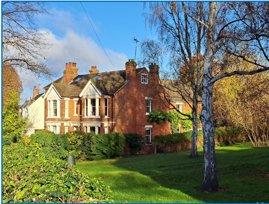
View of side elevation from junction of The Avenue and Chiltern Road
