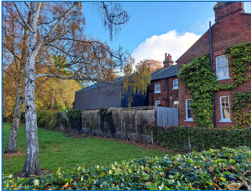
Two storey side / rear extension at 1 Chiltern Road
