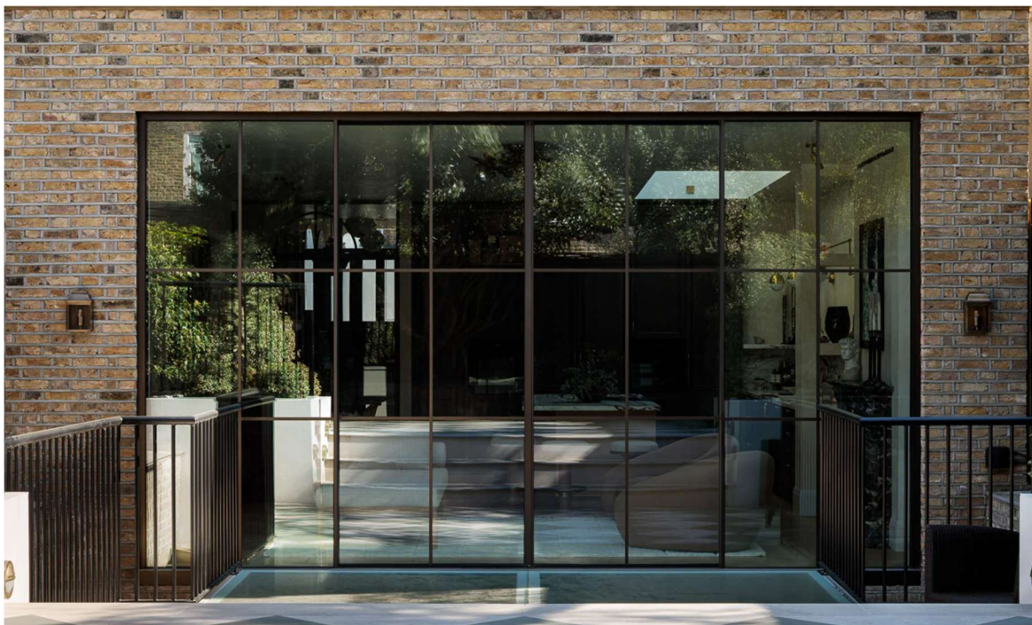
Figure 2 - Perla slimline metal glazing: example of a dark metal framed, multi-pane glazed opening within brickwork.
