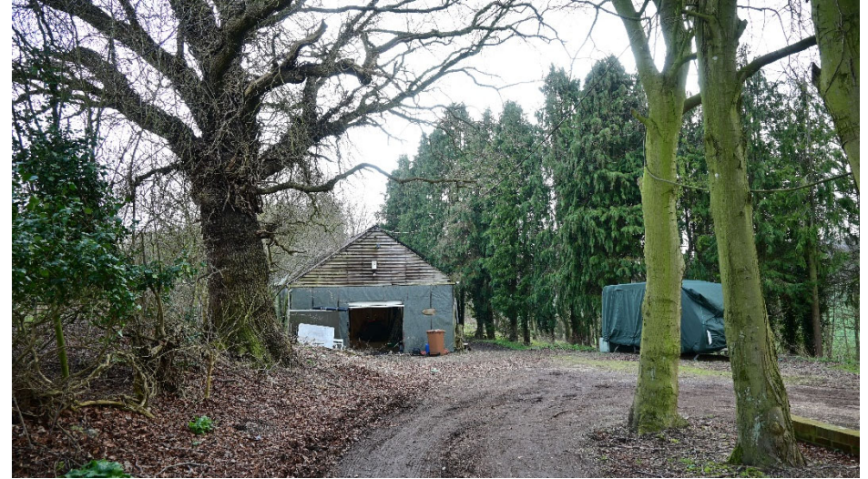
Figure vii - View of outbuilding from existing track.
