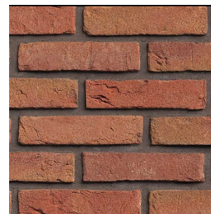
Red facing brickwork.
