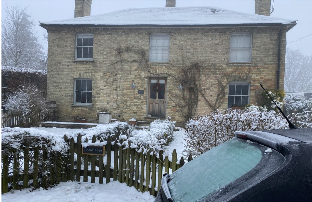
Figure 13: School House, matched yellow brick to Fordham's terrace though slightly earlier in date.
