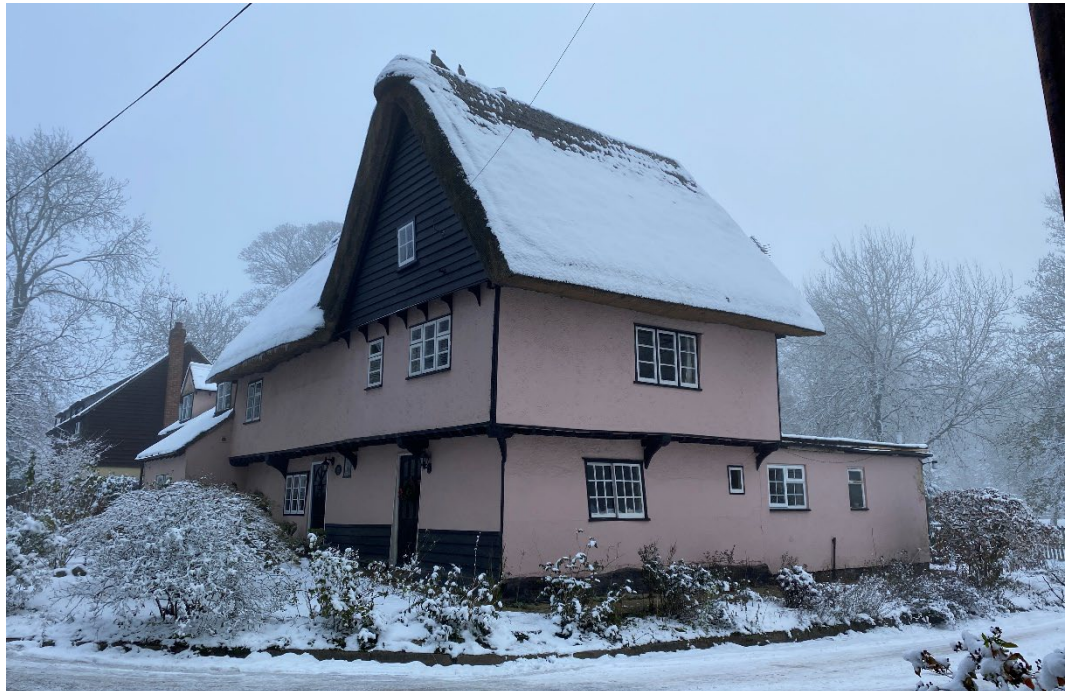
Figure 10: 16 th century Church Cottage with jetties to two elevations representing some of the vernacular architectural tradition within the conservation area.
