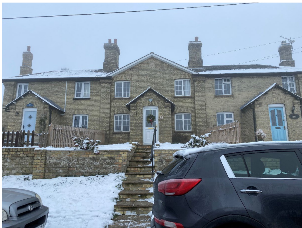
Figure 12: one of the blocks of Fordham's terrace, note elevated level, symmetrical arrangement around the central pediment and pilaster detailing.
