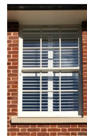
7 - TIMBER SLIDING SASH WINDOWS (STYLE AS INDICATED)
