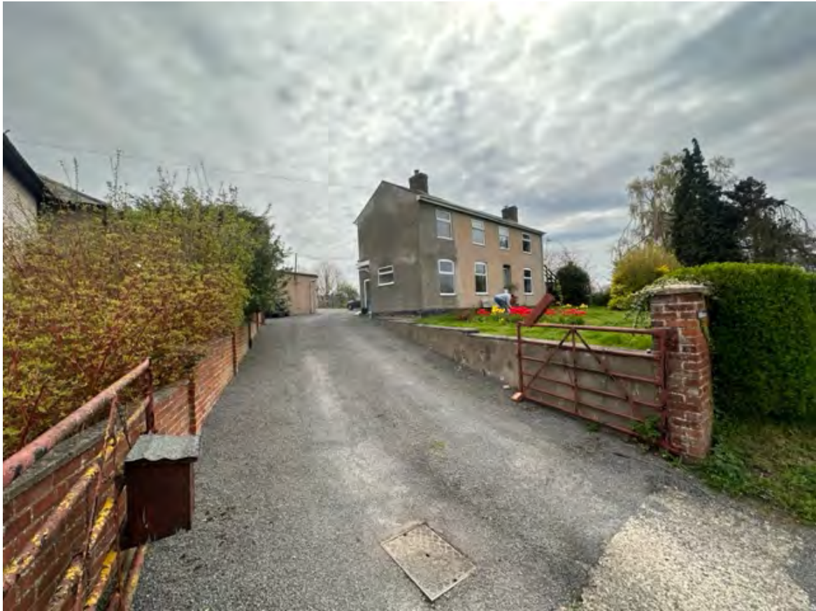
Plate 11: Looking South-east up access road to Hillcrest
