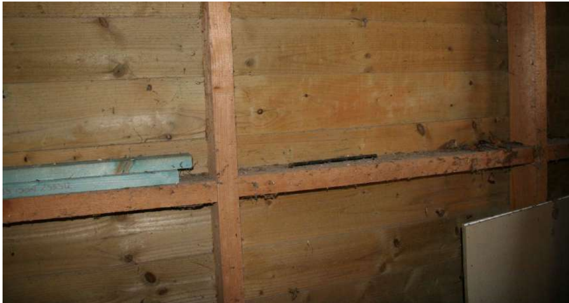
Detail of the partition wall in the NE Garage.
