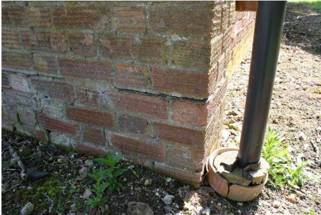
Detail of the textured brickwork and asphalt damp proof course on the NW corner.
