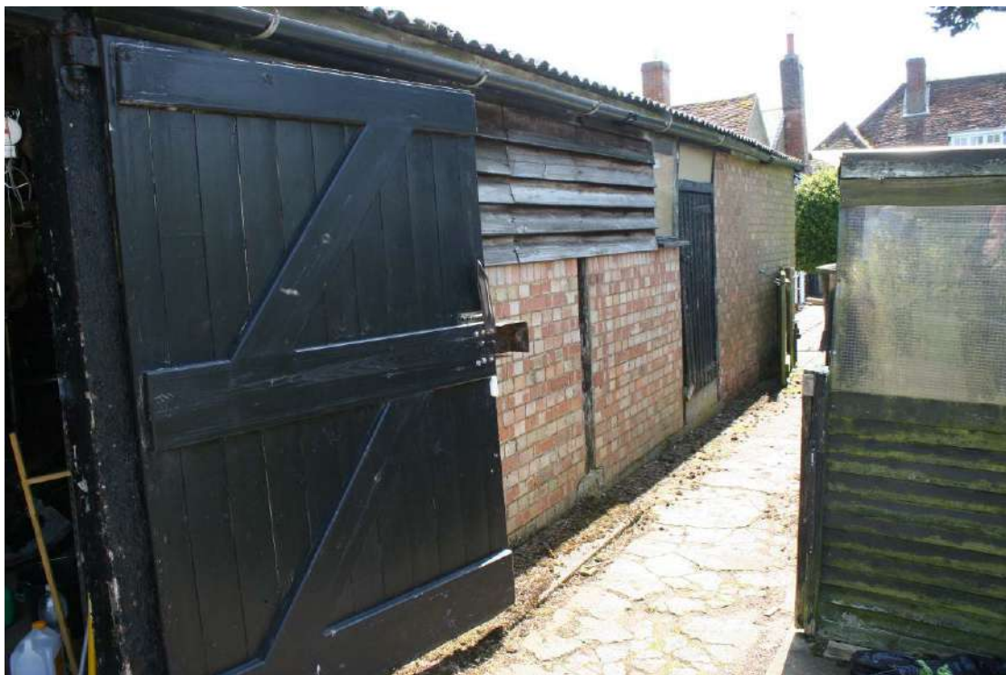
Detail of the door and brick panelled walls. Looking SE.
