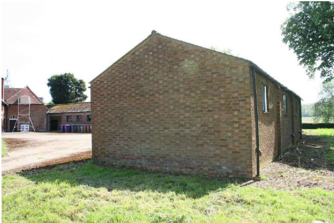
The NW and SW elevations.
