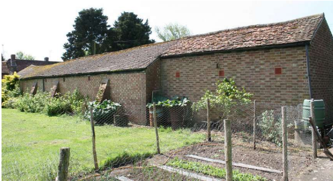
The NE elevation of the Workshop and Stables.
