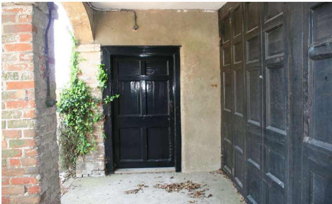
Georgian style six panel door to the East Room.
