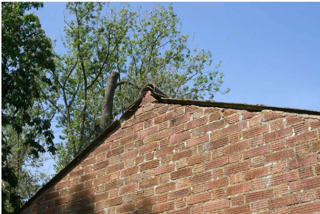
The roof is clad with corrugated cement board.
