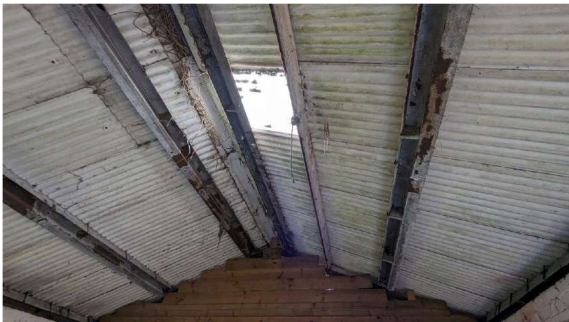
Detail of the steel beam purlins.
