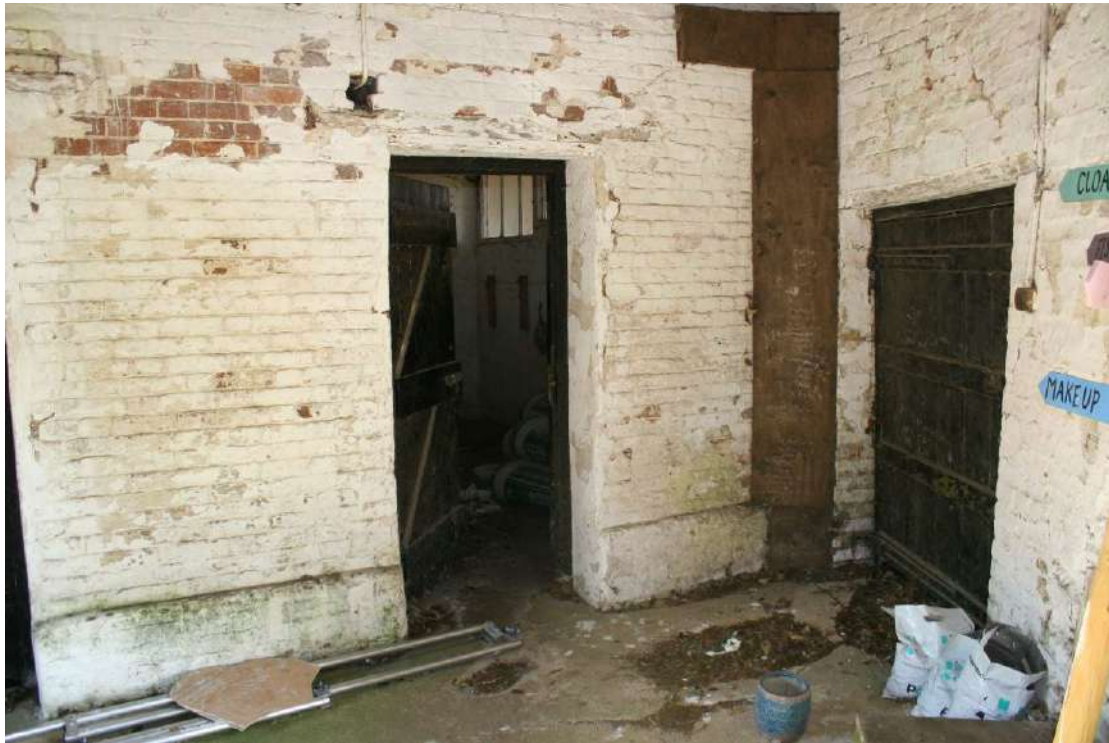
The entrance door to the Work Room.
