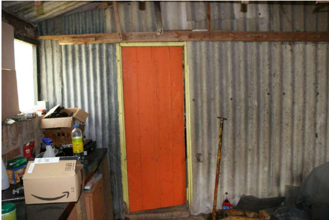
The NW end bay is divided off with a corrugated cement board wall.
