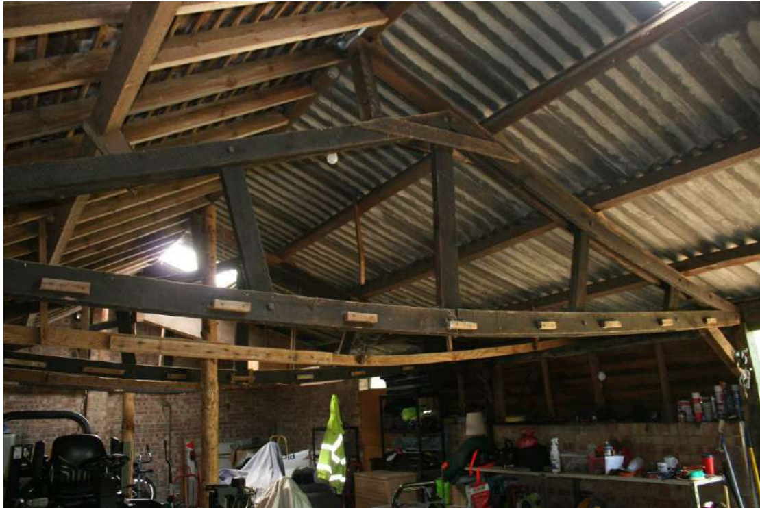
One of the composite trusses looking S.
