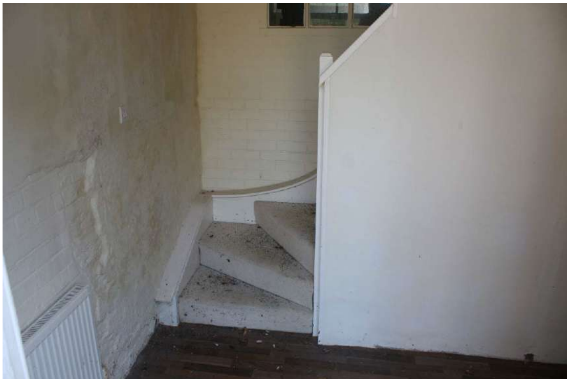
MC20th staircase up to the converted accommodation.
