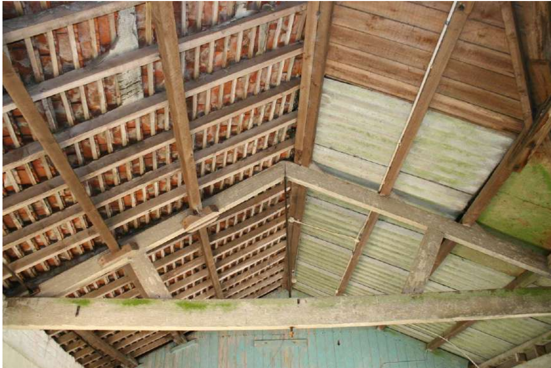
The roof over the carriage arch. Looking SW.
