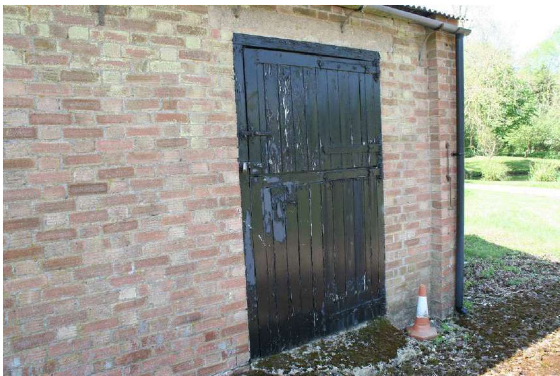
Detail of the split stable doors.
