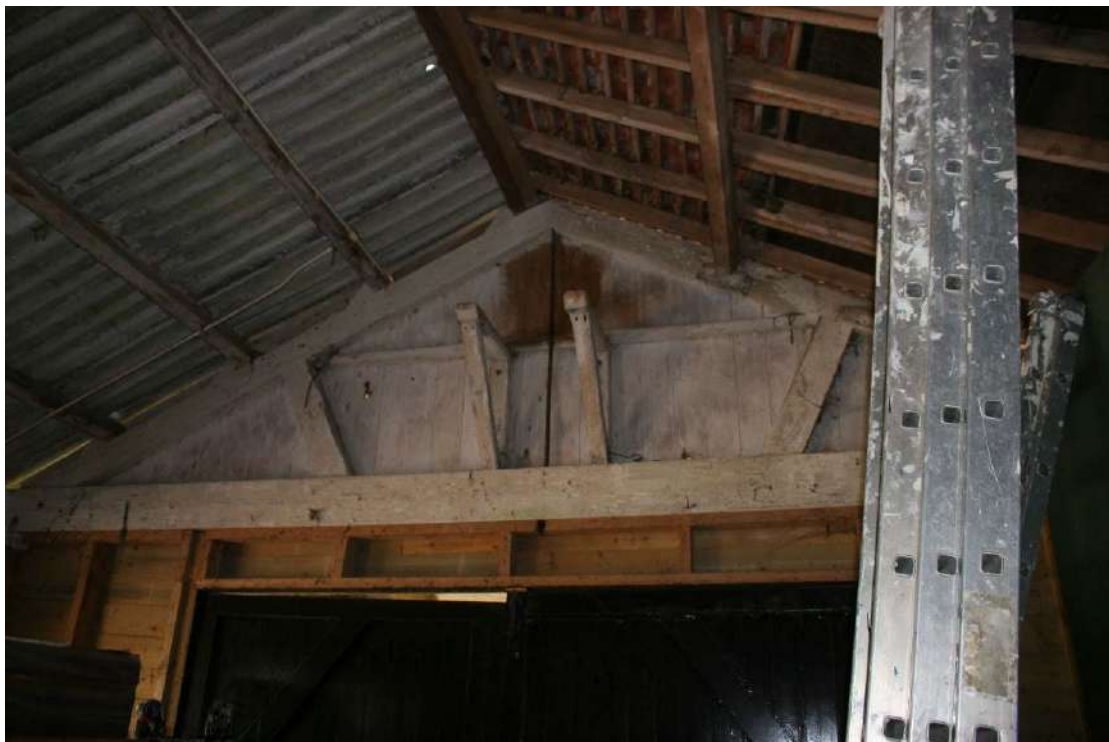
The frame above the garage doors and support for a small tank.
