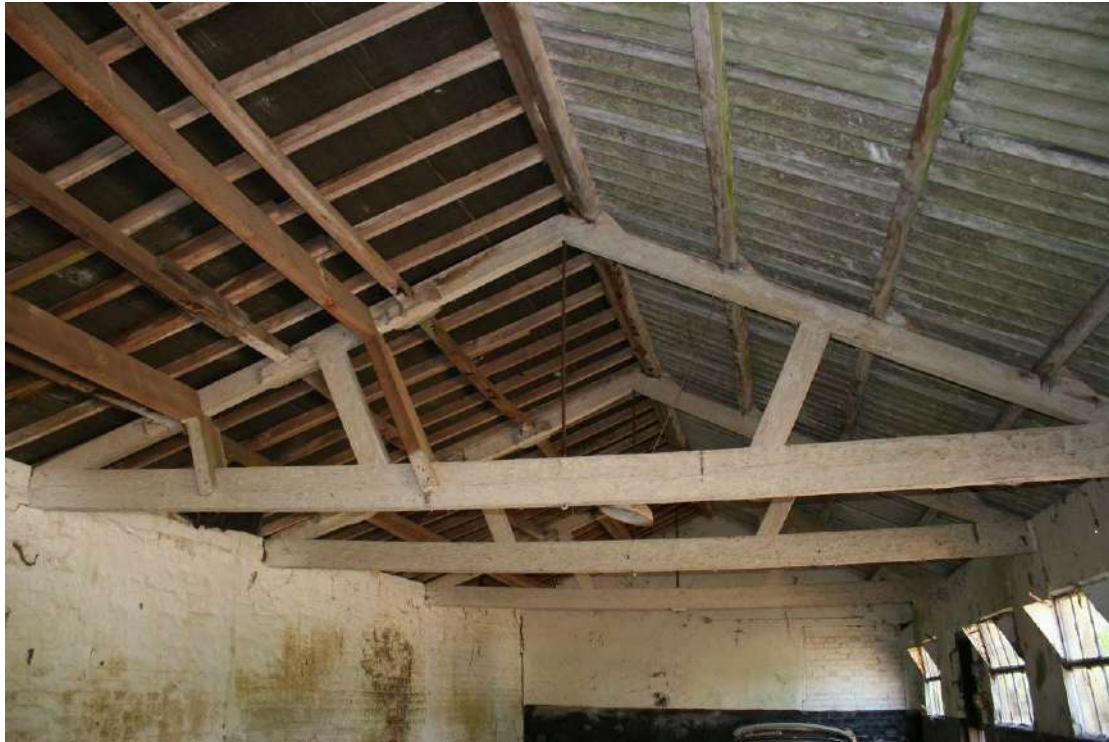
Detail of the roof structure looking SW.
