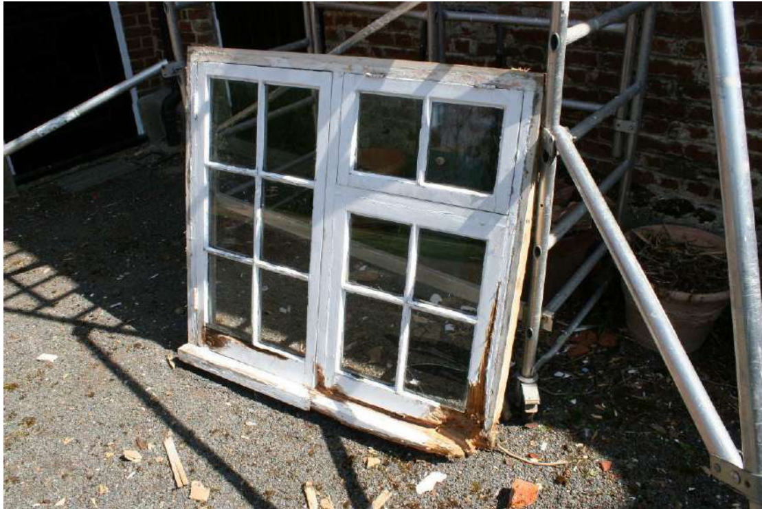
1930's casement window under restoration.
