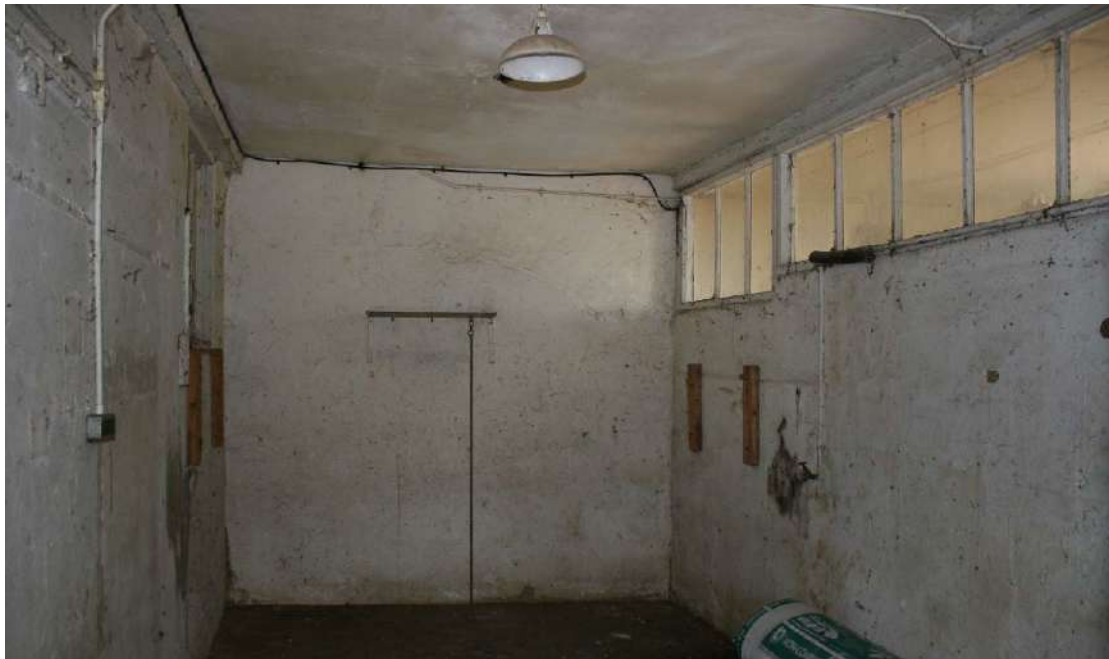
Looking N in the Work Room.
