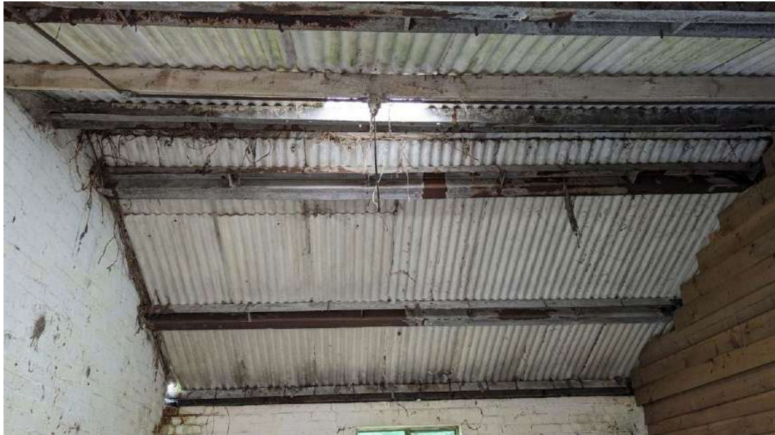
Looking W in the roof of the southernmost bay.
