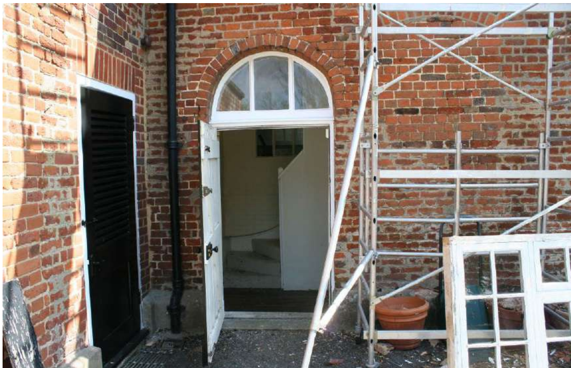
Detail of the blocked western window and inserted doorways.
