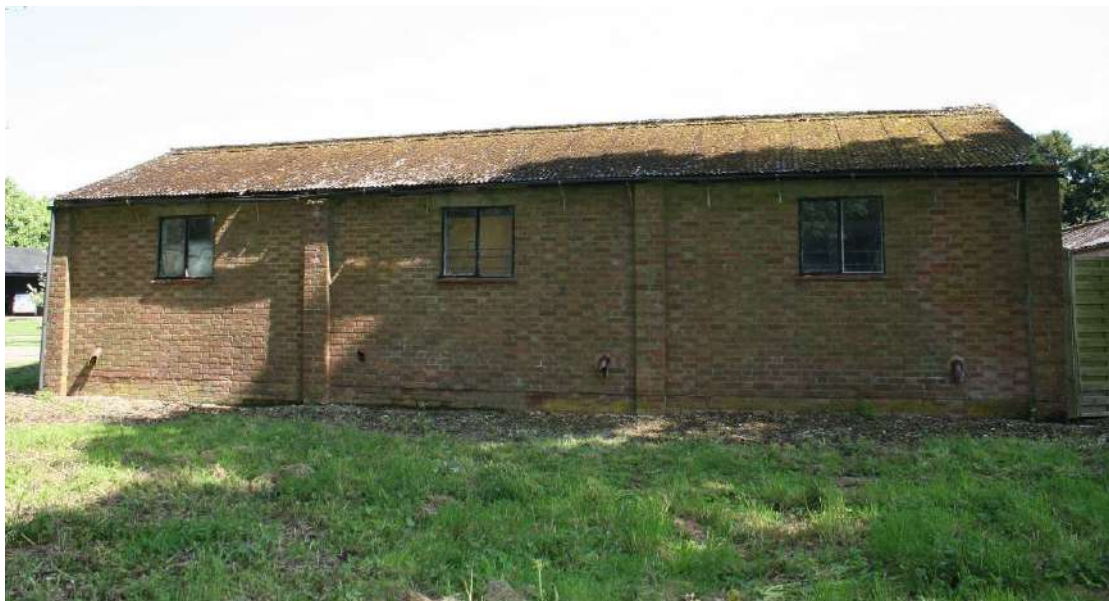
The SW elevation of the Standalone Garage.
