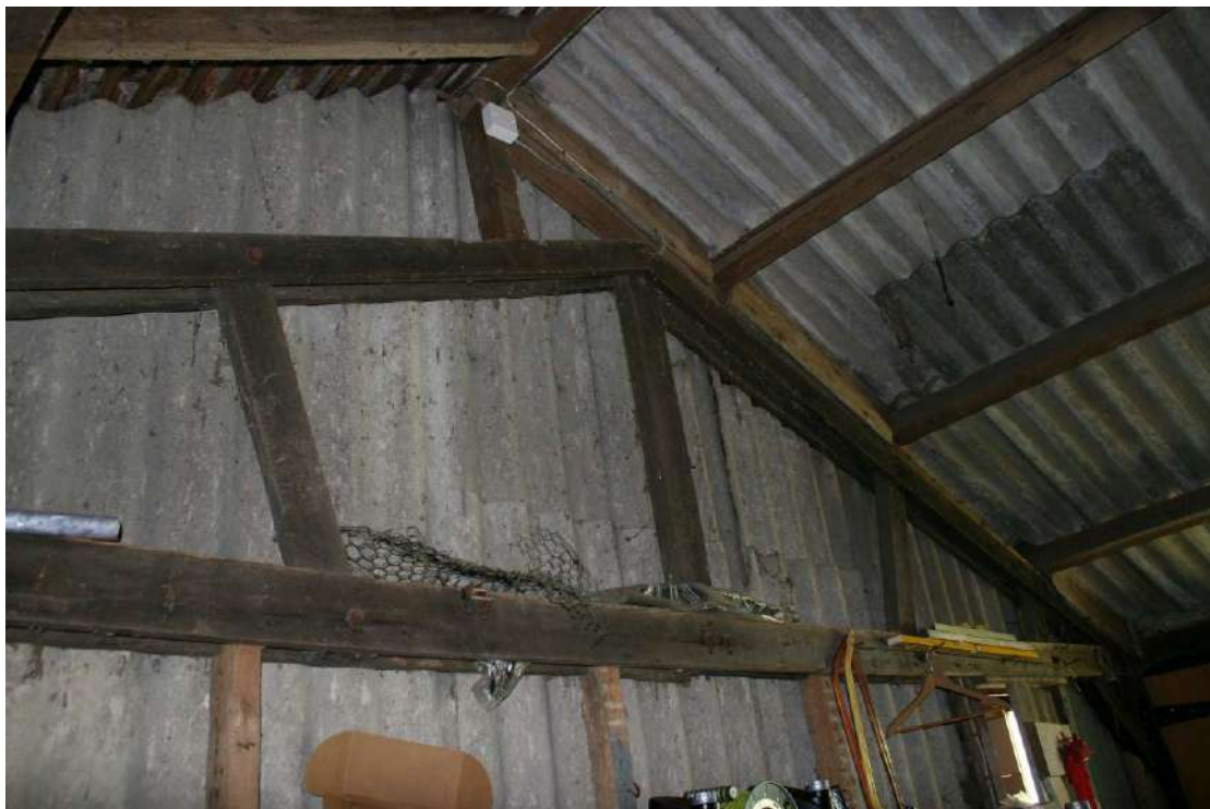
The roof truss and added structure inside the NW end bay. Looking SW.
