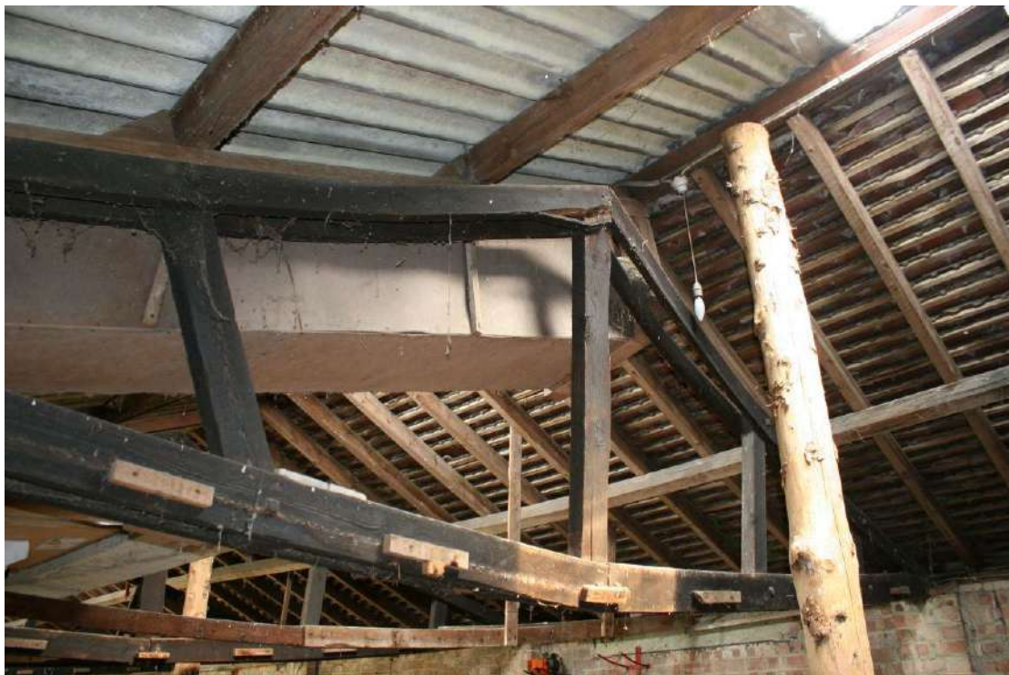
The SW side of the roof has a corrugated cement board roof covering.
