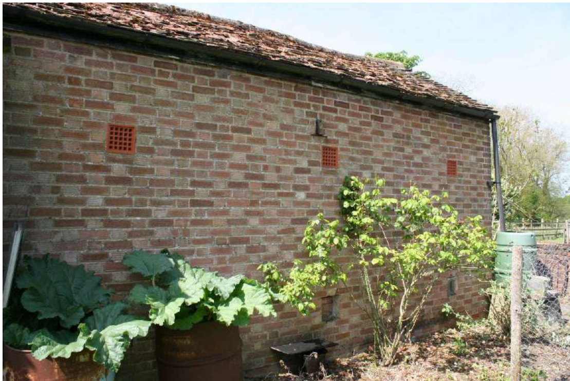
The NE elevations of the Stables.
