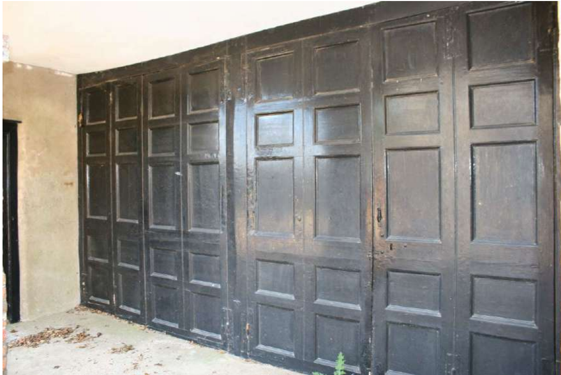
Georgian style coach house doors now used as car garages.
