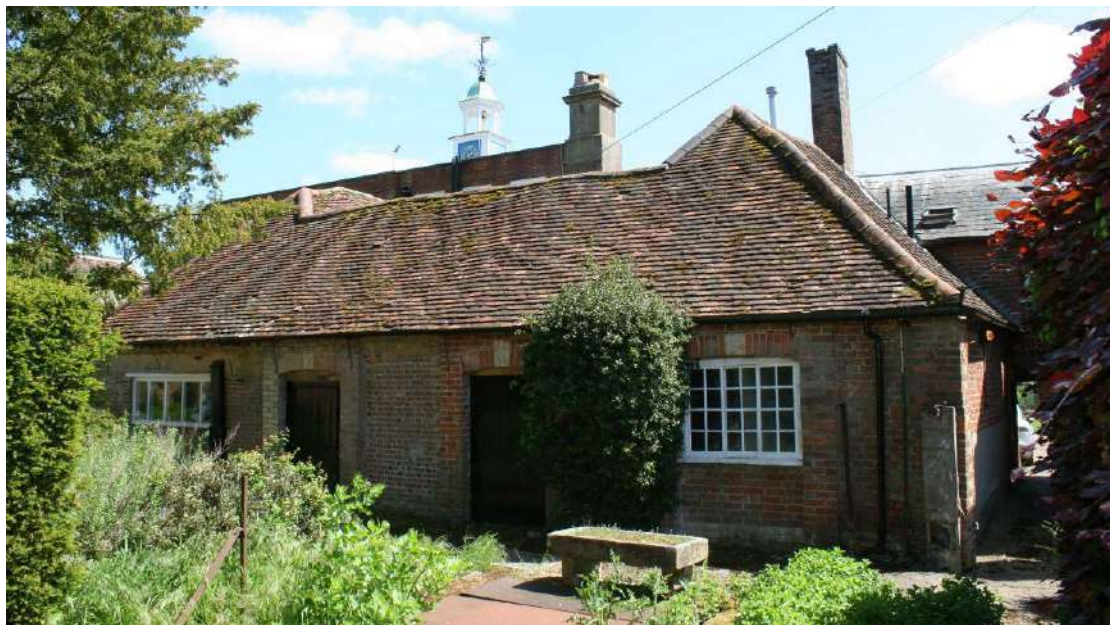
North elevation of the Kitchen.
