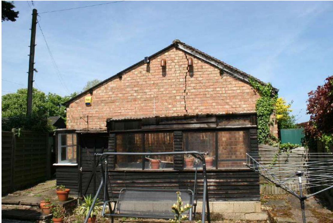
The SE elevation of the Workshop.
