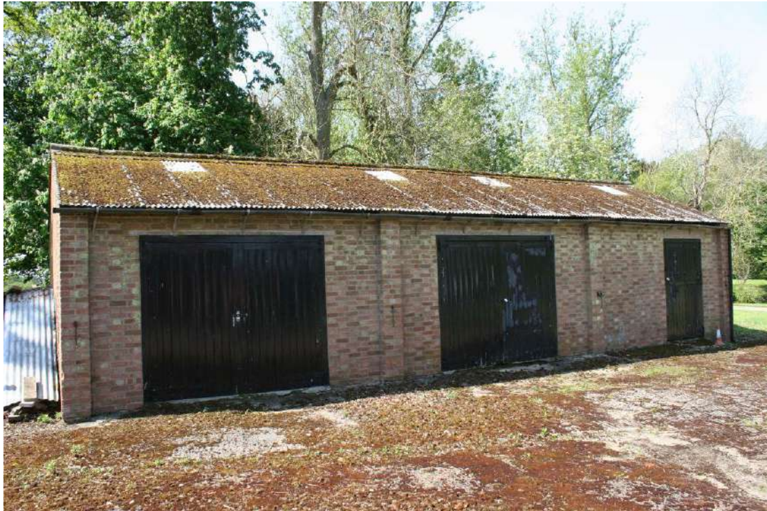
The NE elevation is the working side of the building.
