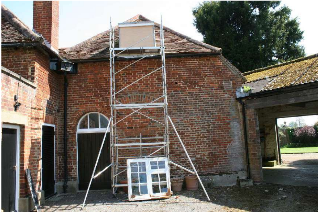
The western elevation of the Coach House.
