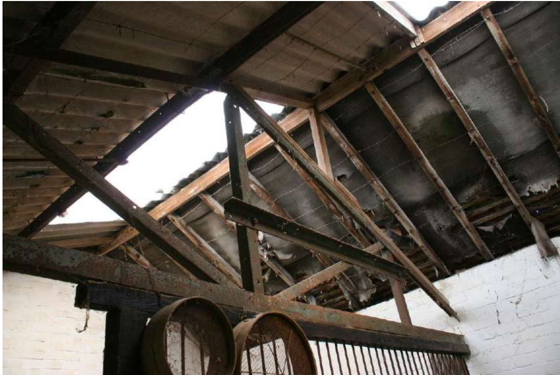
Reused steel roof truss. Looking N.
