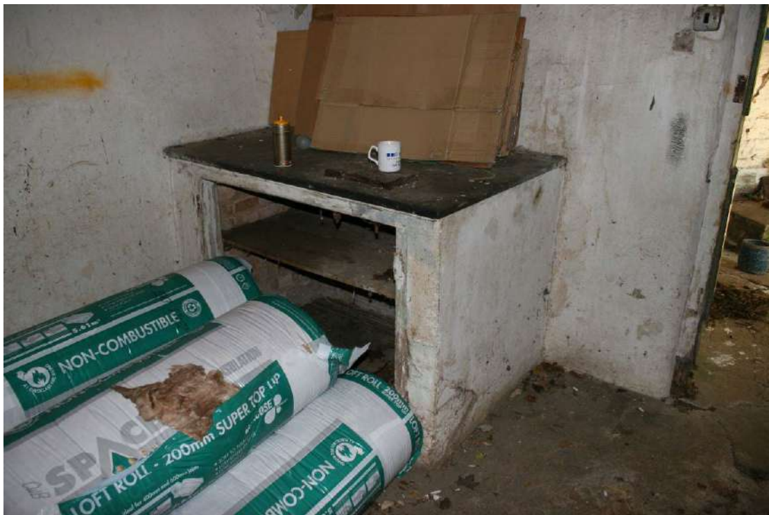
Brick built cabinet with wooden shelves and slate top.
