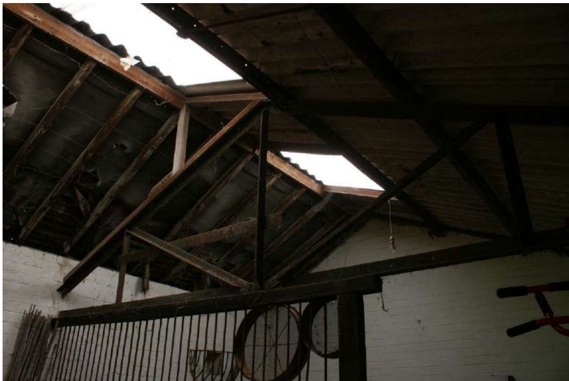
Reused steel roof truss. Looking S.
