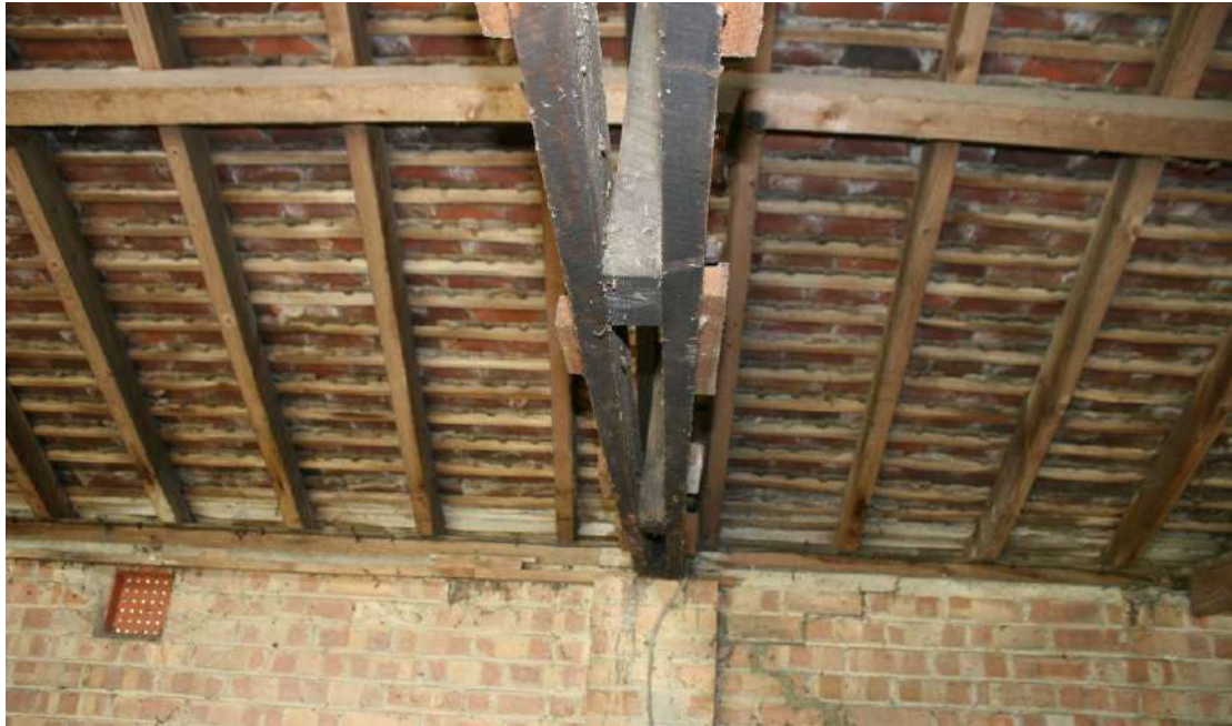
Detail of one of the composite trusses and the NE side of the roof with nibbed tiles.
