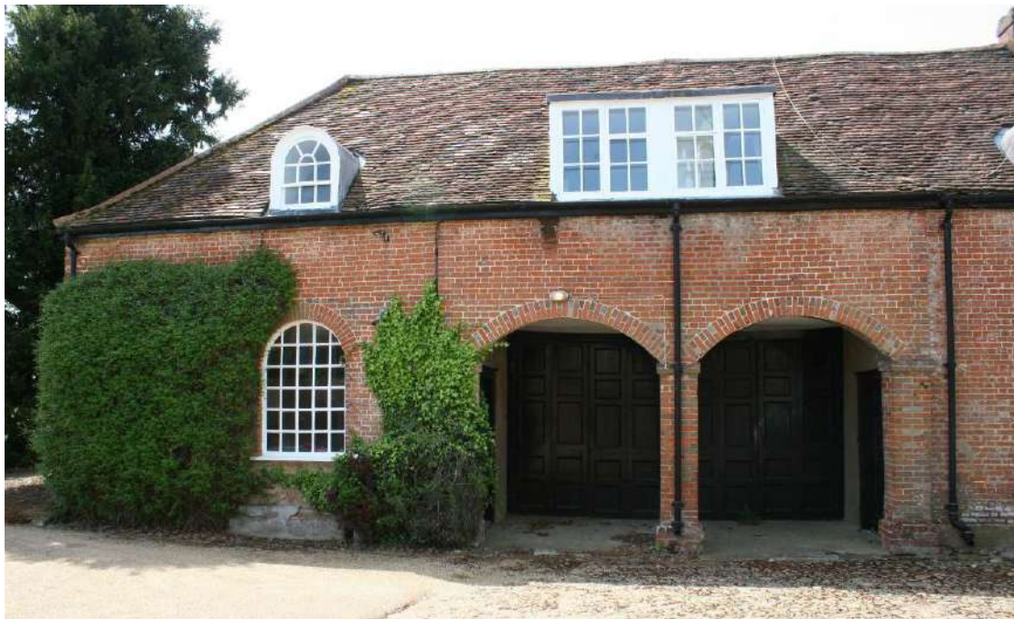
The Coach House east elevation.
