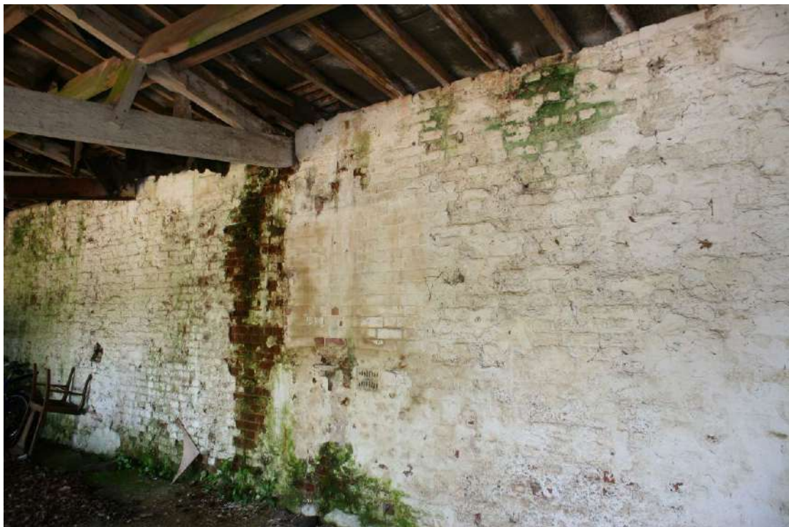
Bricked up window in the SE wall.
