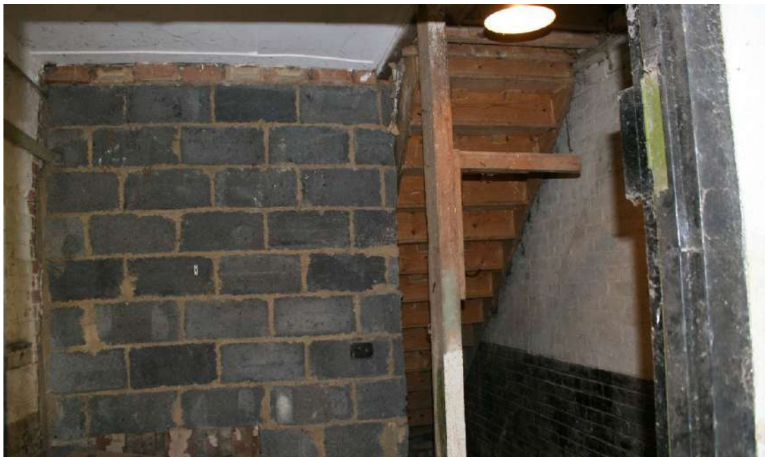
Looking N in the Storeroom.
