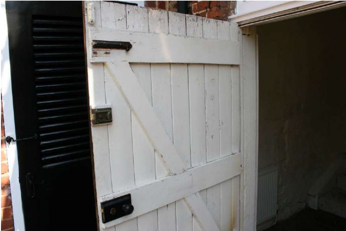
MC20th door into the stairwell for the Coach House.
