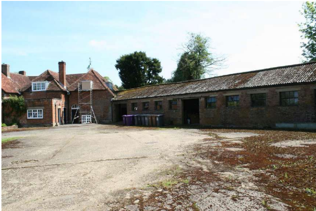
The NW elevation of the Long Garages in relation to the Coach House. Looking E.
