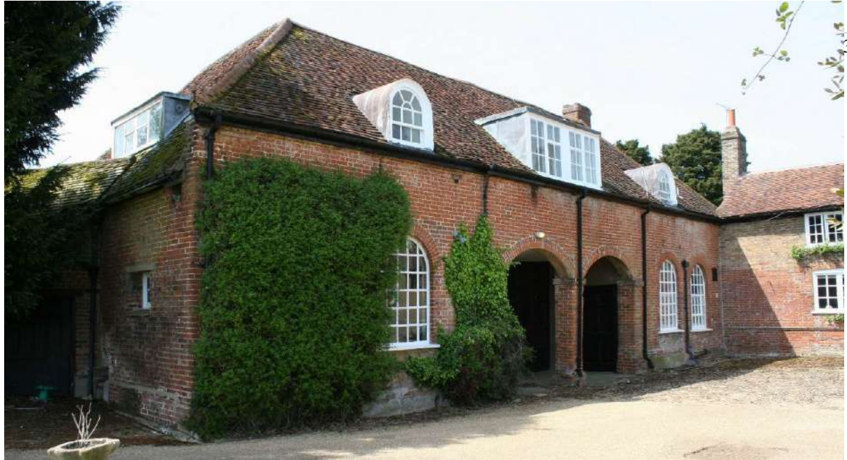
BJHC. 08 05 2024. The east elevation of the Coach House.
