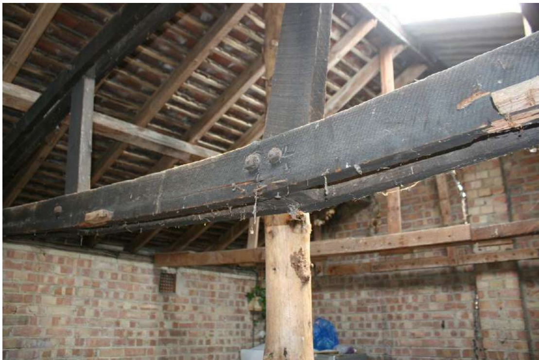
Detail of the bolted construction of the trusses.
