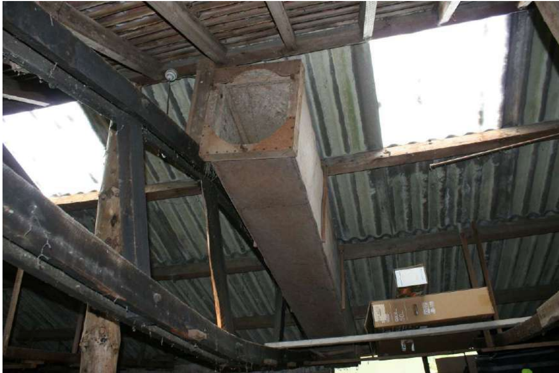
There is a timber duct fitted in the roof.
