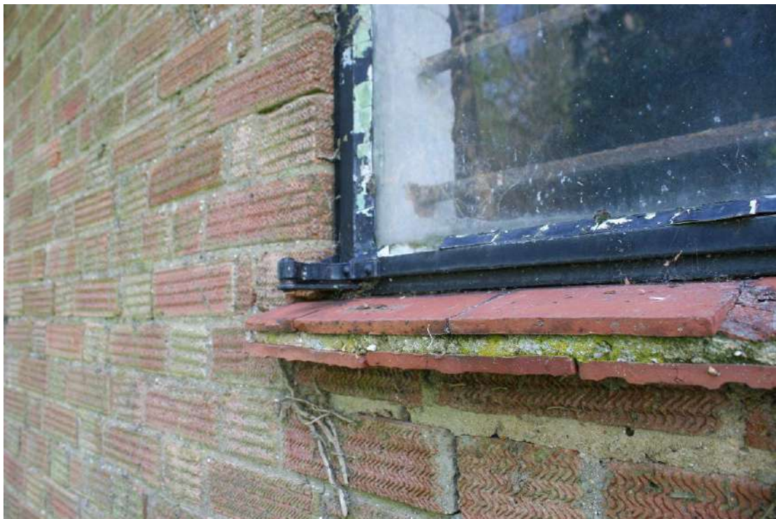
Detail of the brickwork, windowsill and Crittall style windows.
