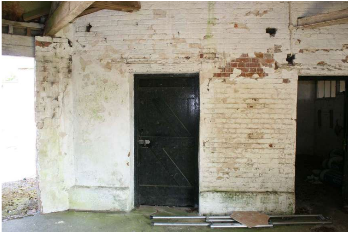
Door into the Storeroom. Note it is hung backwards.
