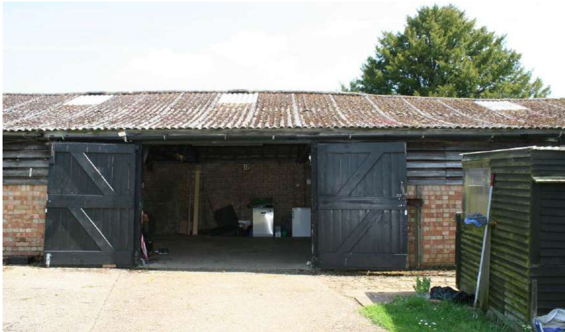
The garage doors in the SW elevation.
