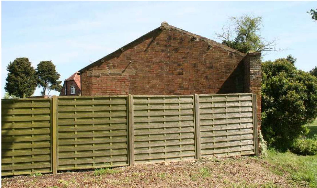
The SW elevation has a blocked doorway for an internal passageway.
