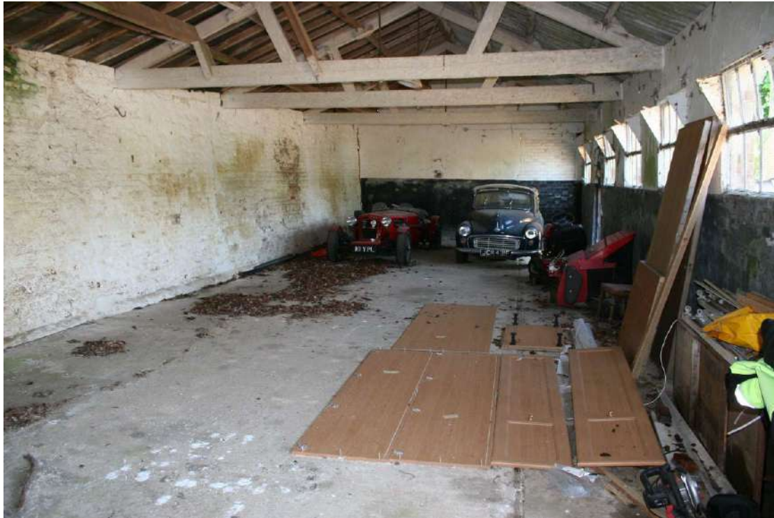
Looking SW in the Long Garage.
