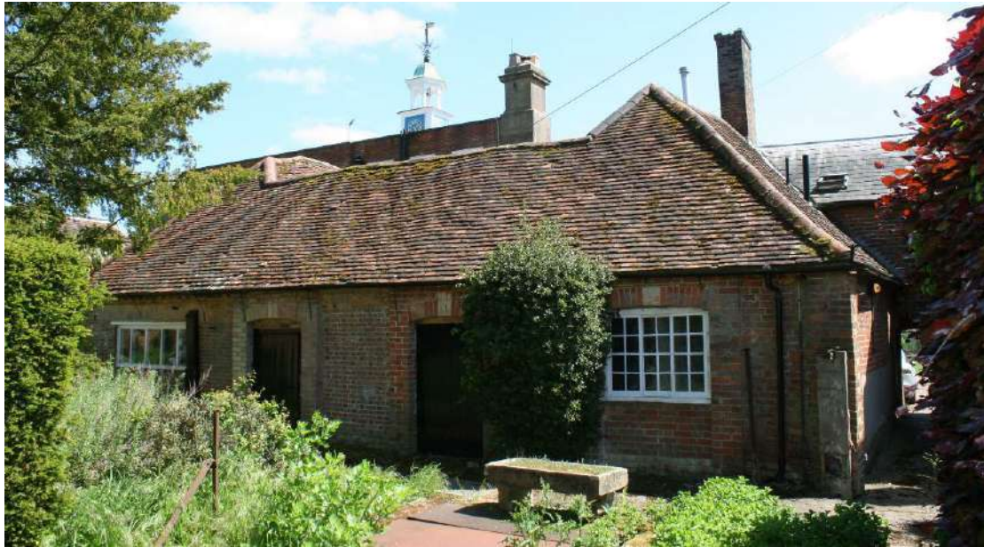
The north elevation of the Kitchen in context with the House.
