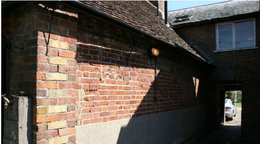
The western elevation looking SE.
