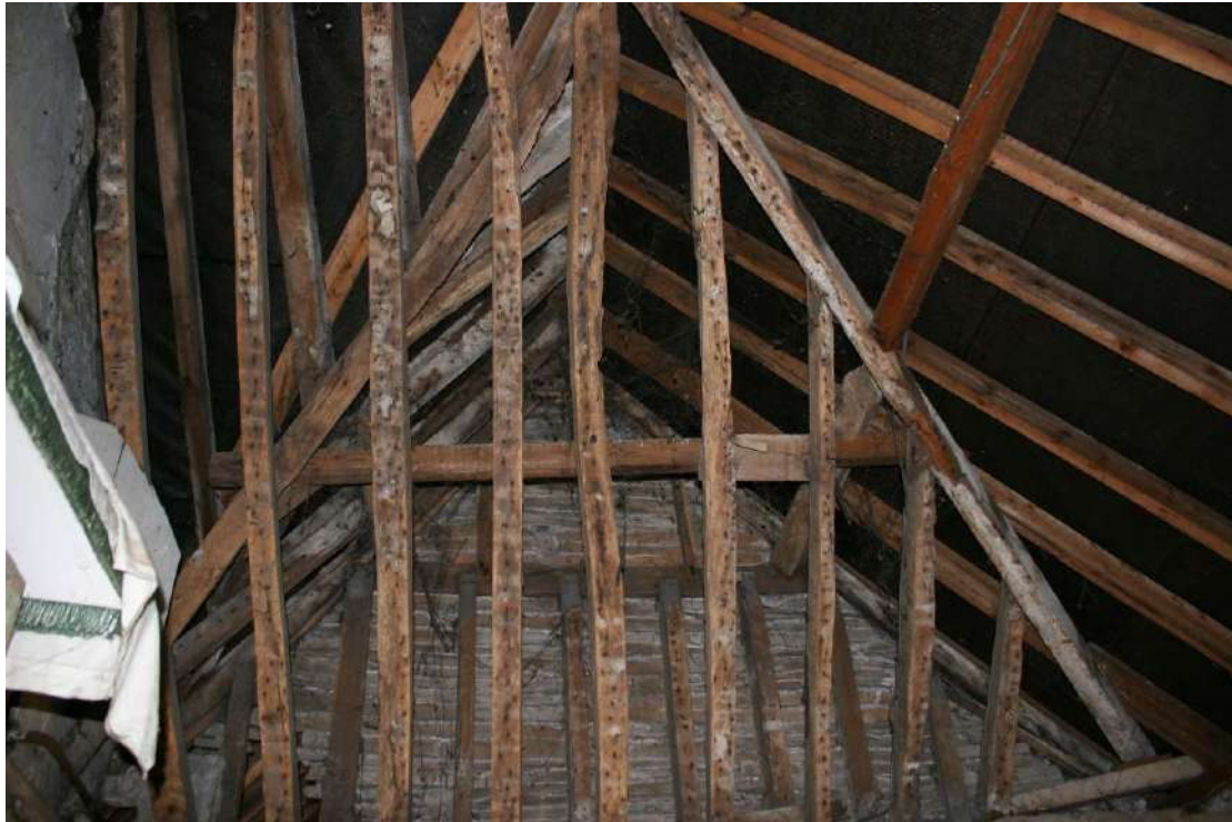
Looking E in the Store at the older rafters.
