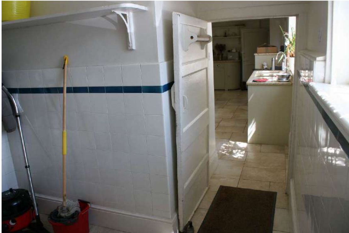
The doorway into the Kitchen has a four panel Art Deco door. Looking E.
