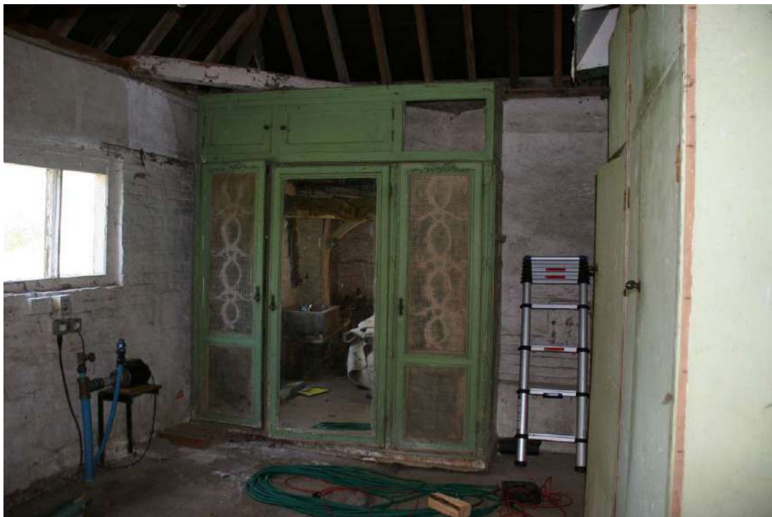
Looking W inside the Store.
