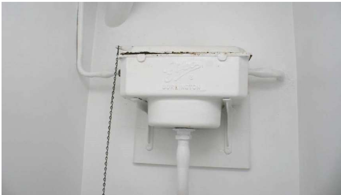
The original 1939 cast iron cistern.
