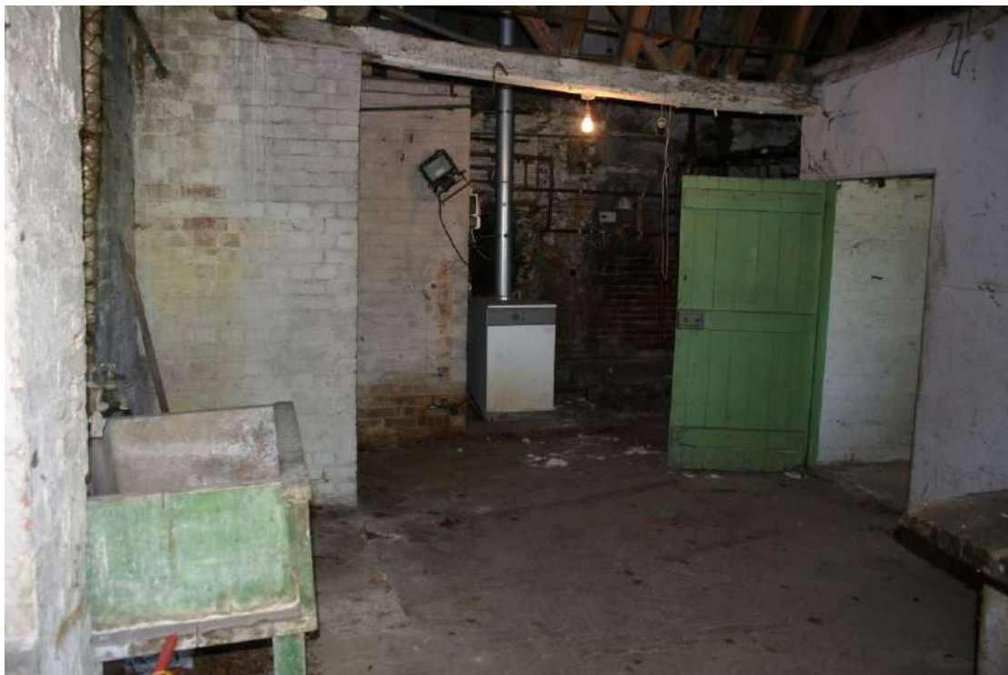
Looking S in the Boiler Room.
