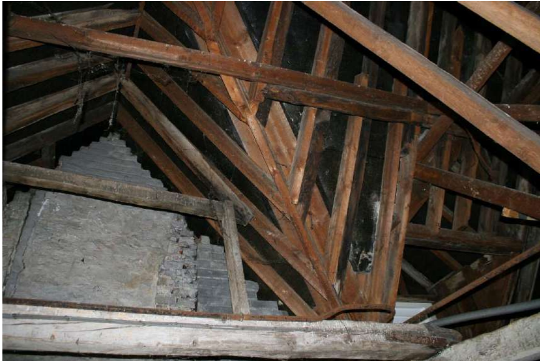
The roof over the wooden sink.
