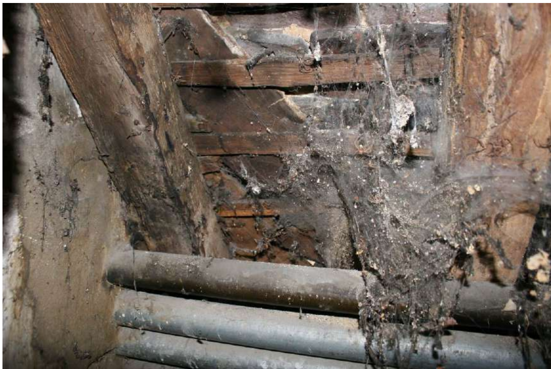
A section of 1939 original roof tiling with narrow laths.
