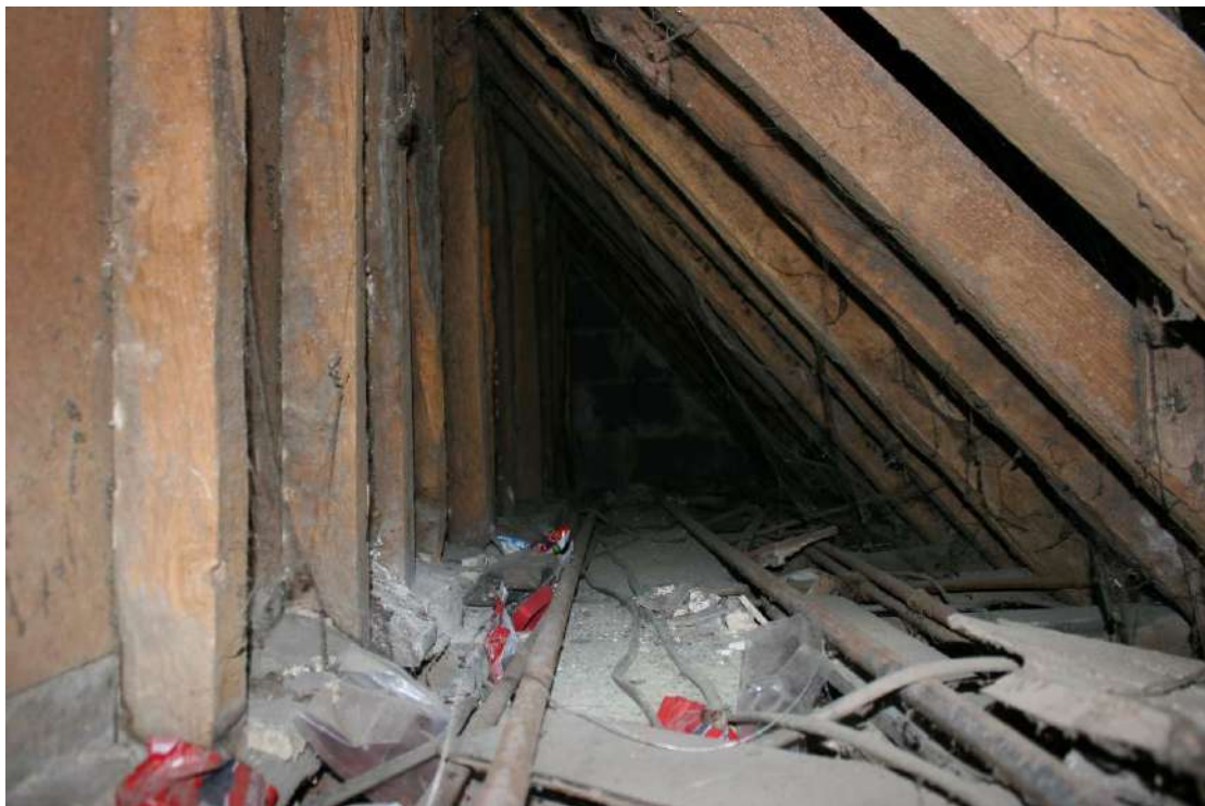
Looking S along the ceiling over the Store corridor.
