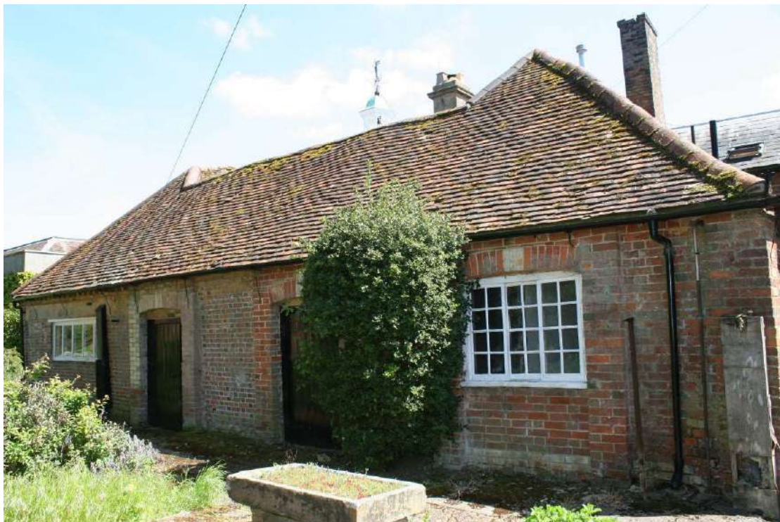
The north elevation of the Kitchen with MC20th doors and windows.
