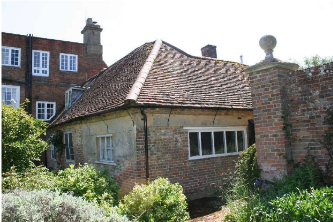
The north and east elevations of the Kitchen range.
