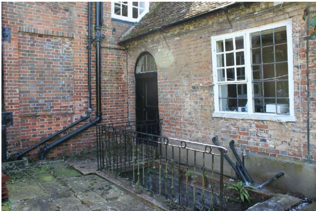
External entrance to the Cellar and doorway to the servant's corridor.
