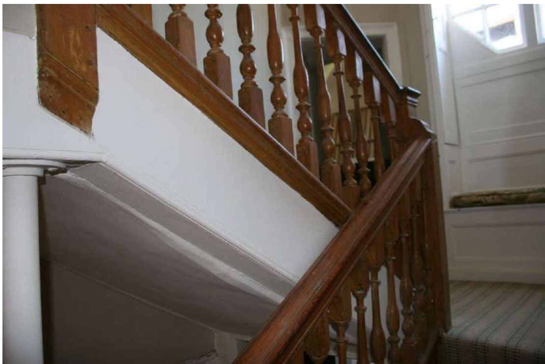
The staircase at the half-landing.
