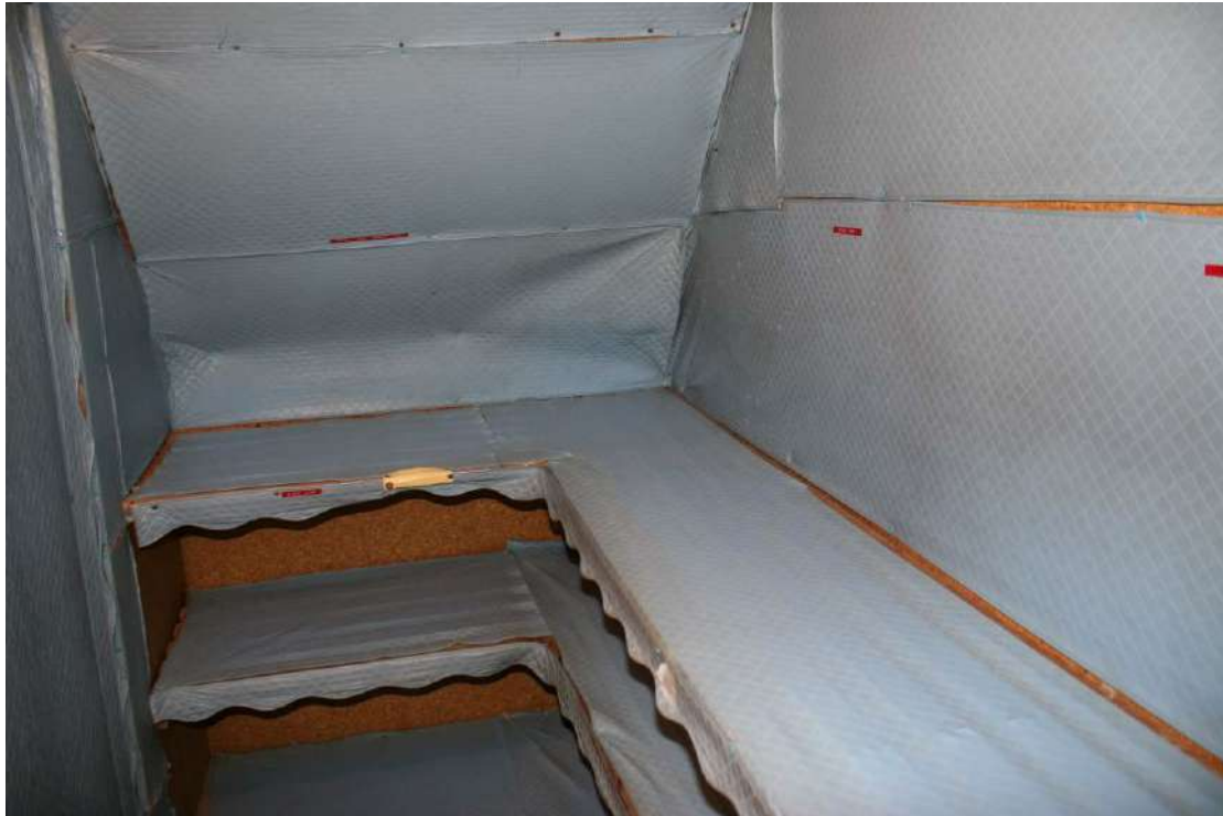
The delicates room is lined with material fixed with drawing pins.
