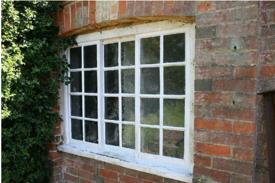
Detail of the replica horizontal sliding sash window and brickwork.
