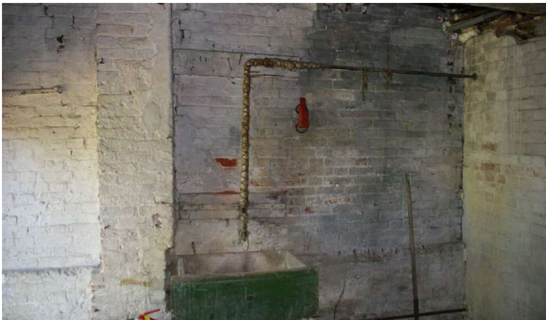
The brickwork has been remade where a fireplace has been removed.
