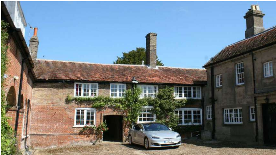
The Kitchen wing ends to the RHS of the archway. South elevation.
