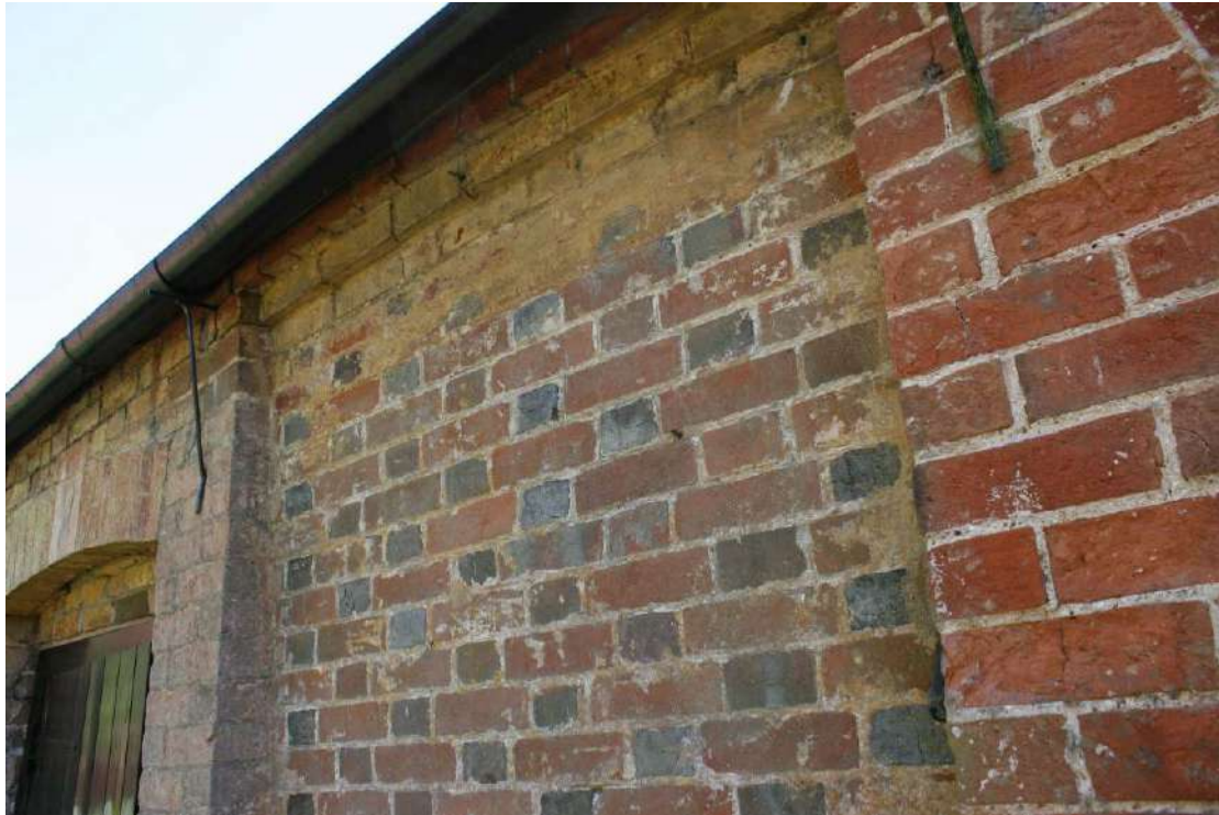
Detail of the chequerwork brick panel.
