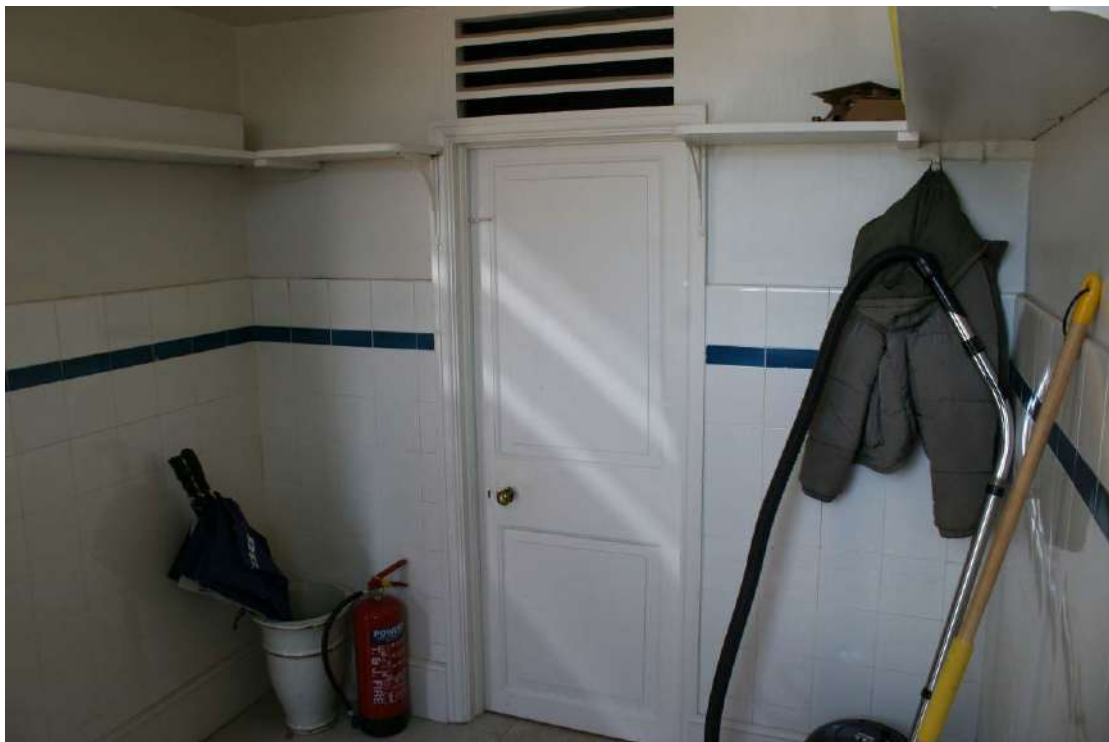
Looking N at the Georgian style two panel Closet door in the Kitchen Lobby.
