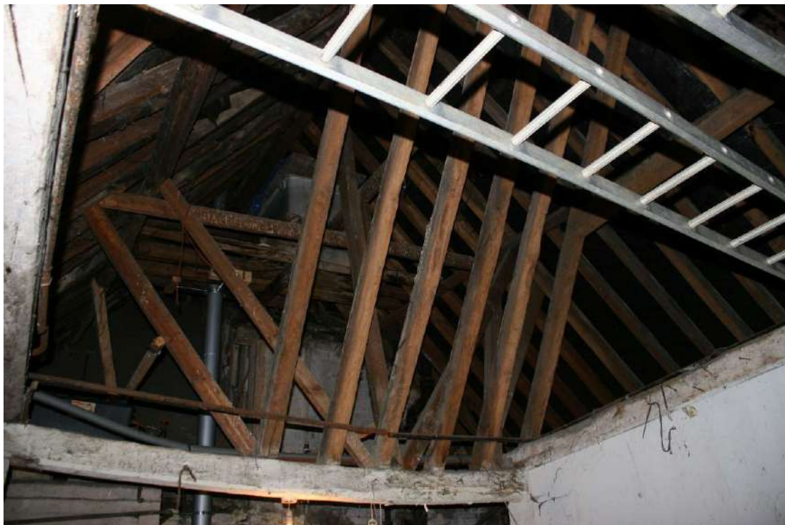
The roof looking N towards the chimney.
