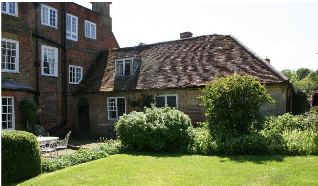
The east elevation of the Kitchen range.
