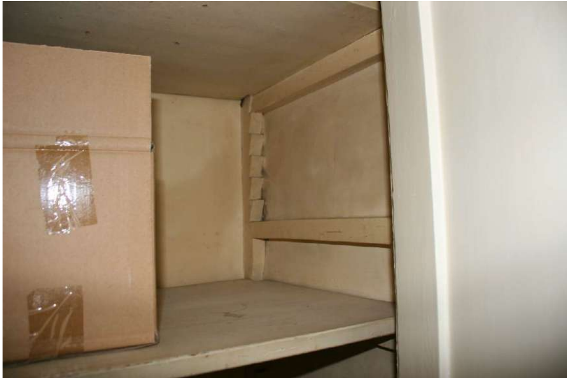
Detail of the variable height shelving inside the cabinets.
