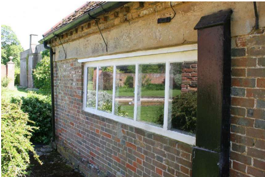
Detail of the 5 light window. Note the modillion cornice.
