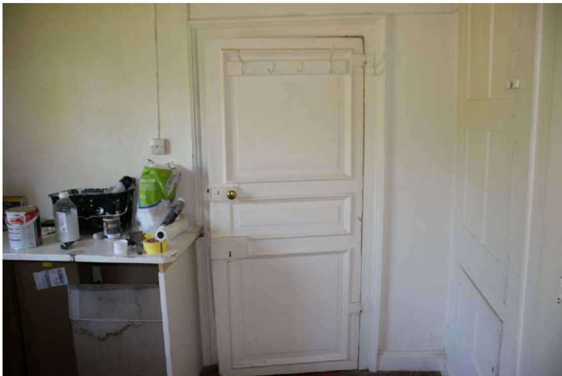
The inside face of the door.
