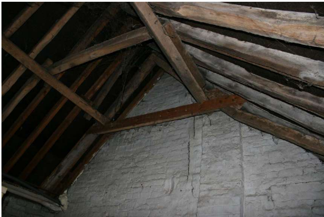
The roof above the wood store.
