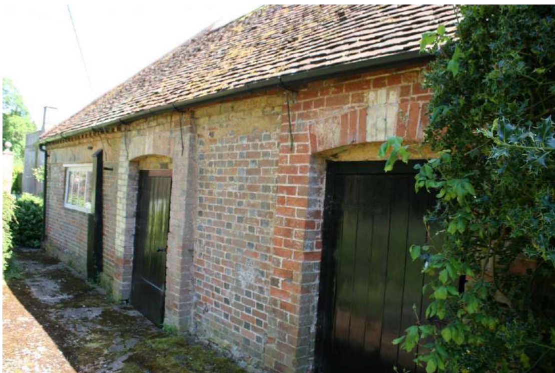
Detail of the various brickwork panels and 1939 doors.
