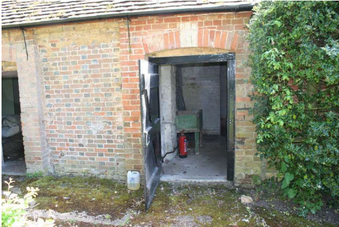
Looking S into the Boiler Room.
