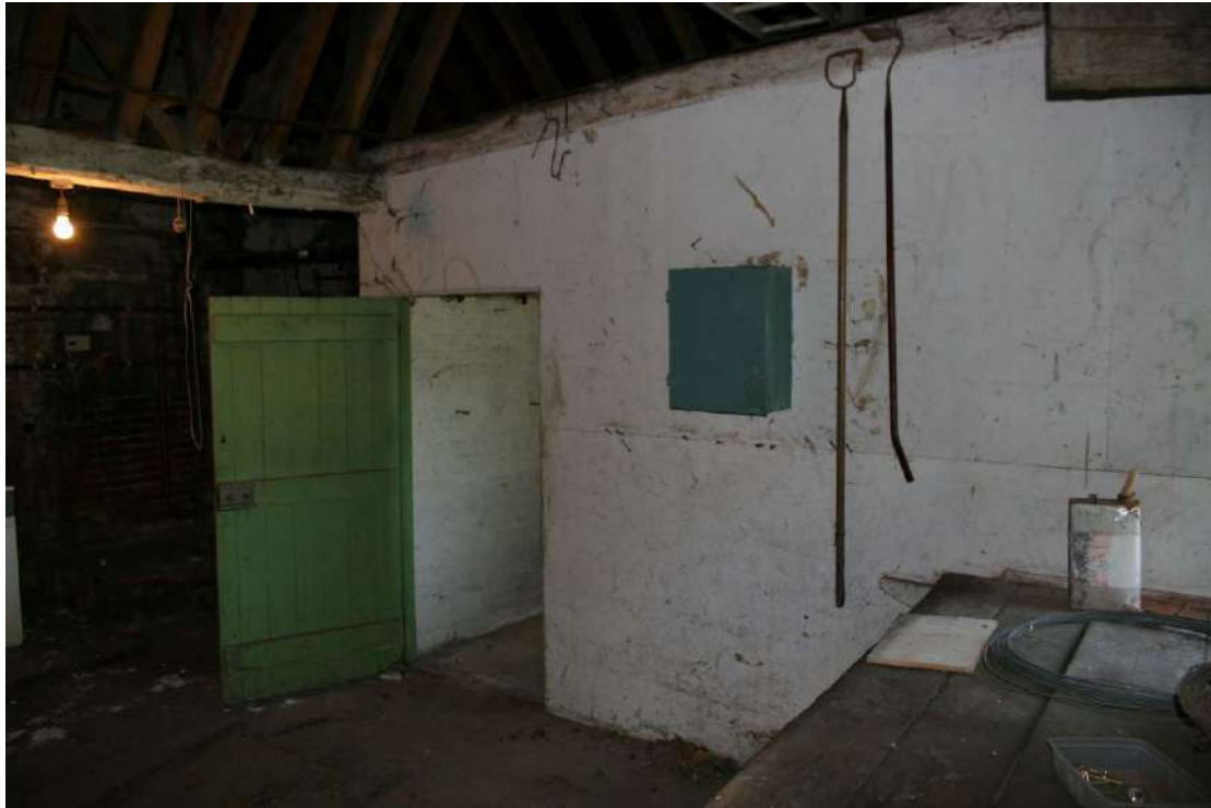
A small workshop has been inserted into the Boiler Room.
