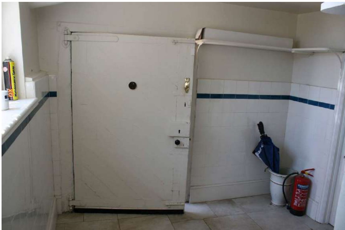
The back of the side door has been reinforced with diagonal boards.
