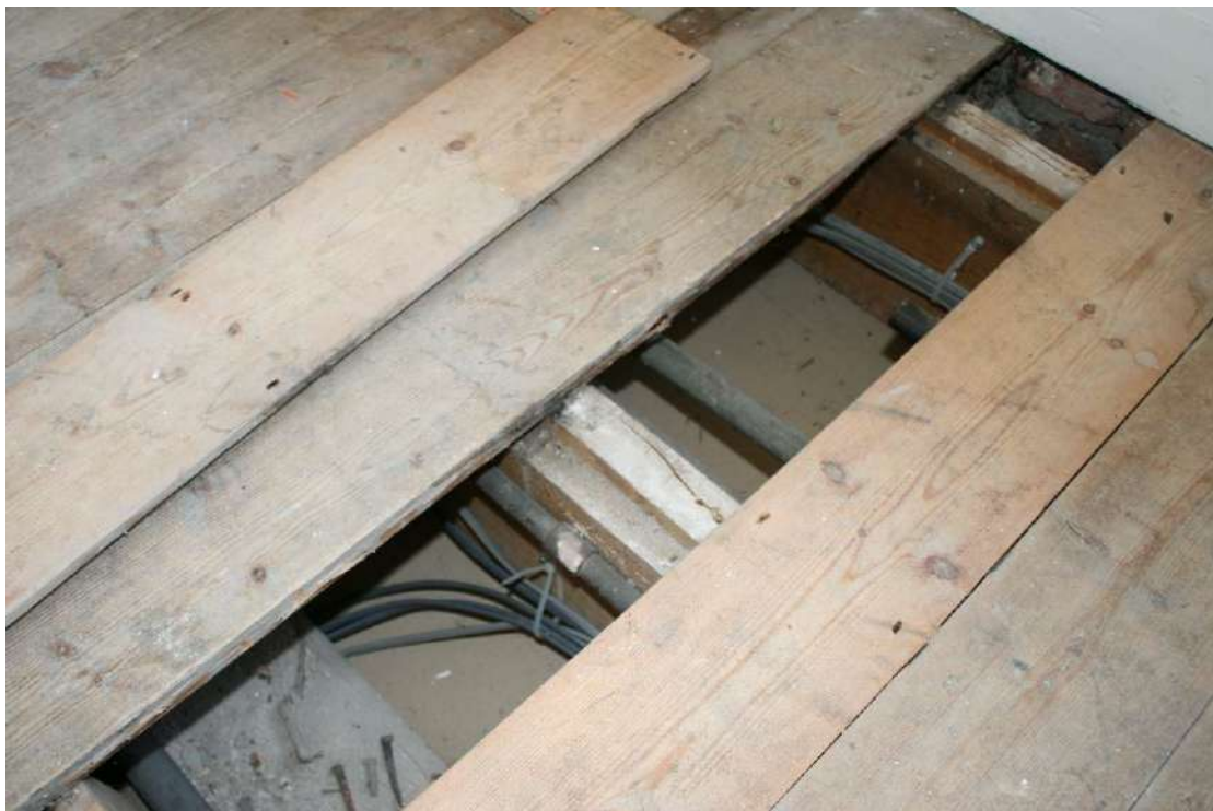
Lifted boards in the Bedroom show the machined timber joists.
