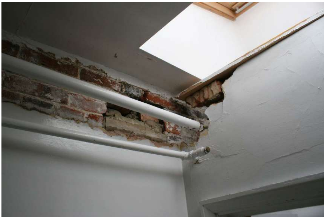
Looking S in the WC Lobby.
