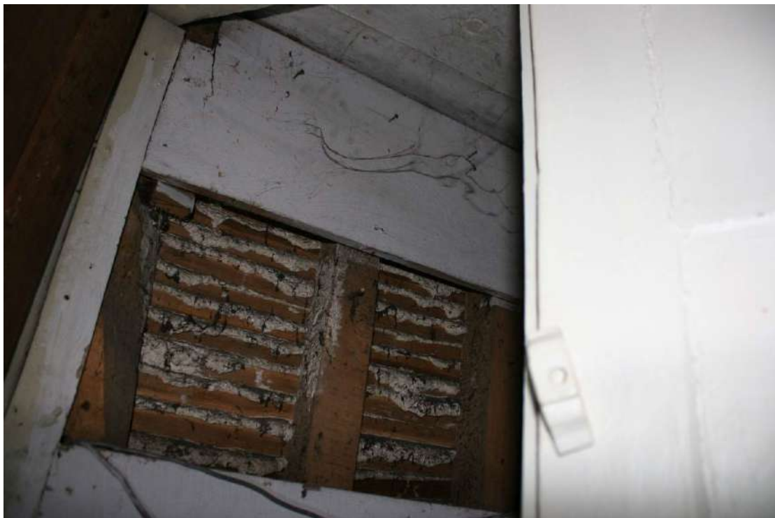
Lath and plaster panel with riven laths on machined softwood studs in the closet.
