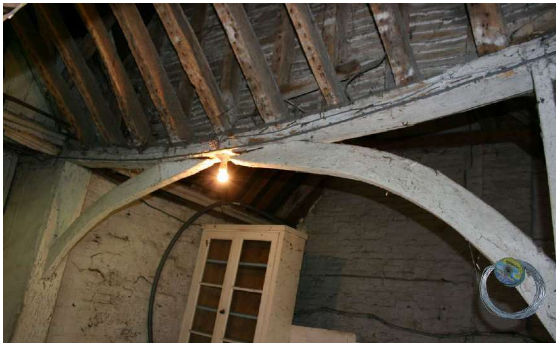
Looking E in the Store. Inserted braces.
