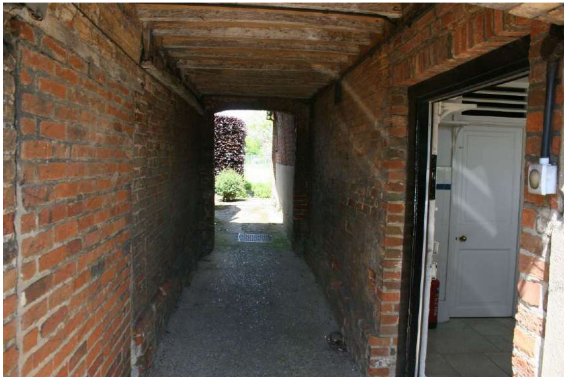
The side door to the Kitchen Lobby looking N.
