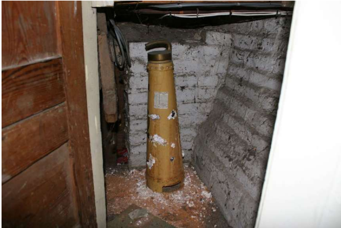
Inside the closet revealing the firestack seen in the Butler's Pantry corridor.
