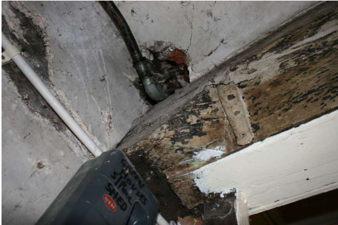
The end of the fireplace bressummer in the westernmost cupboard.
