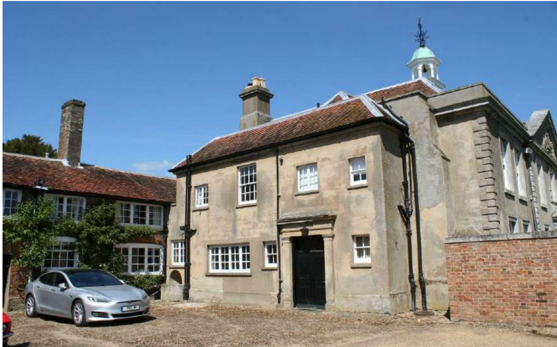
The Kitchen wing and the western elevation of the House.
