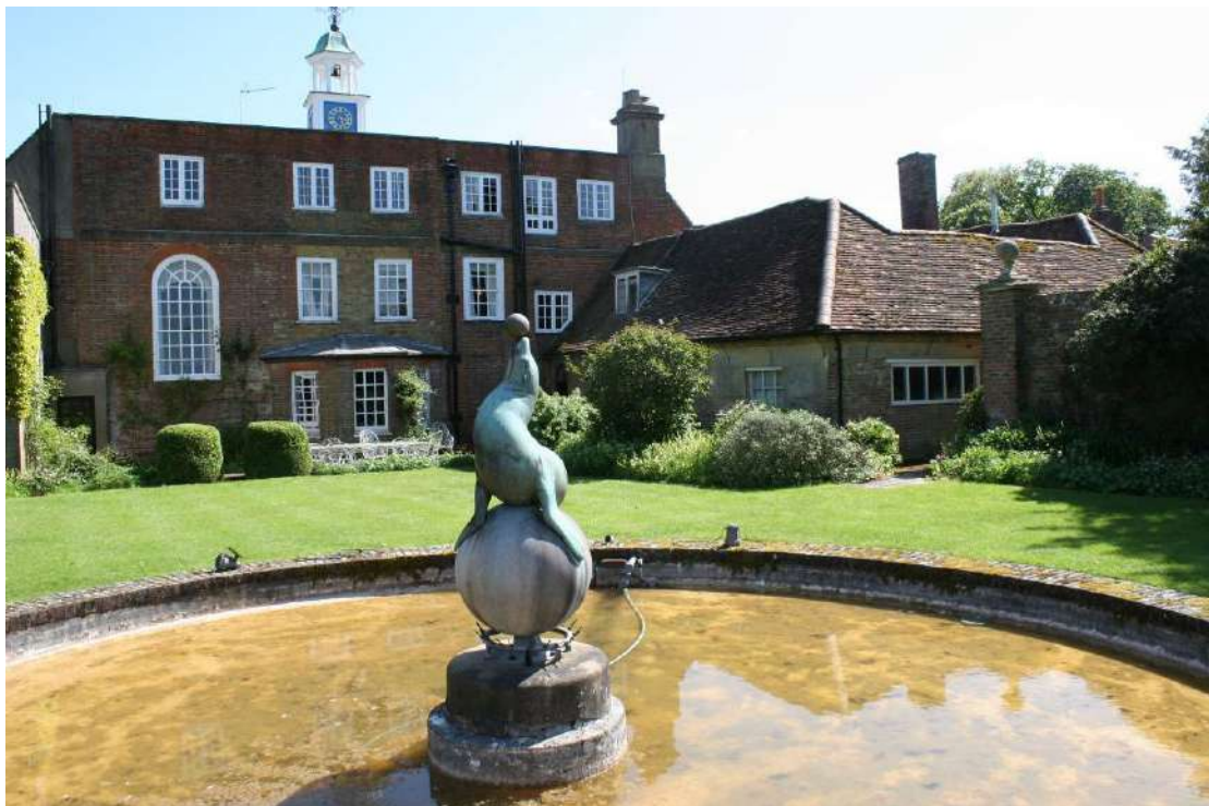
BJHC 26 05 2023. North elevation of the House with the Kitchen.
