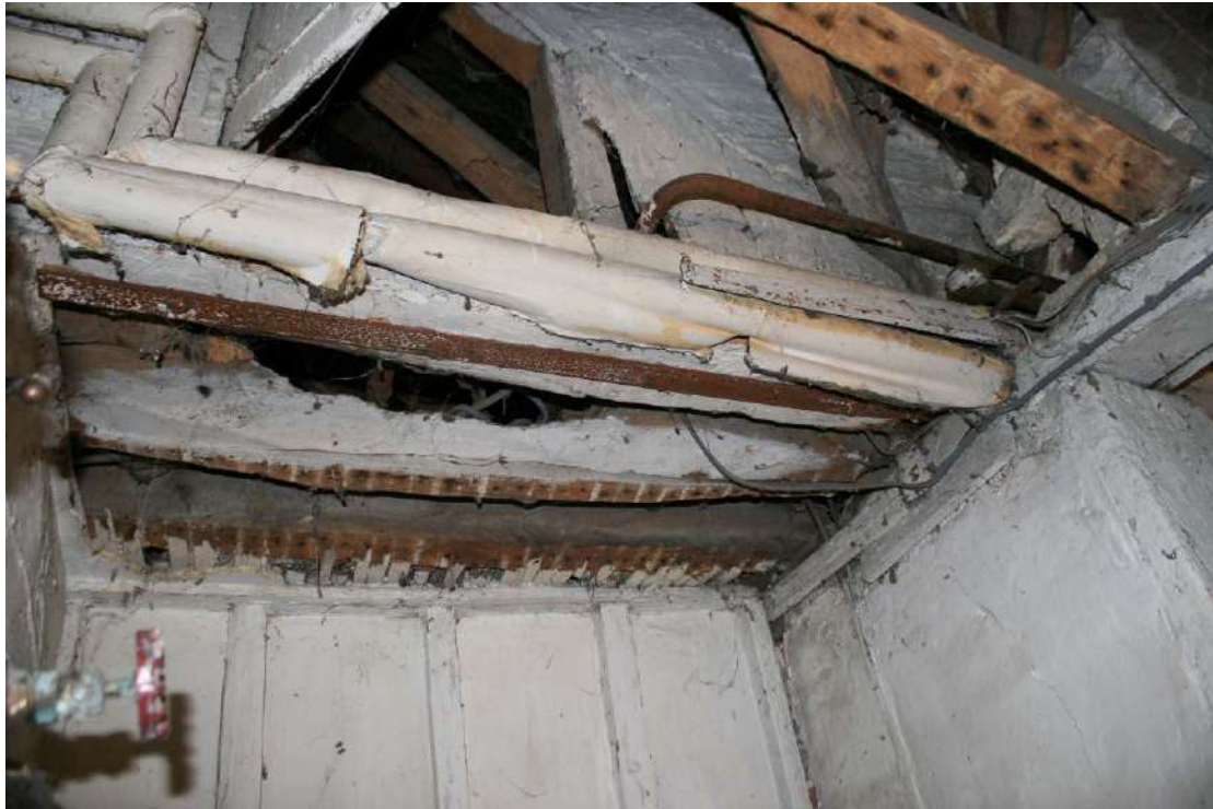
Access door above the Kitchen door. The frame is reinforced with a steel beam.
