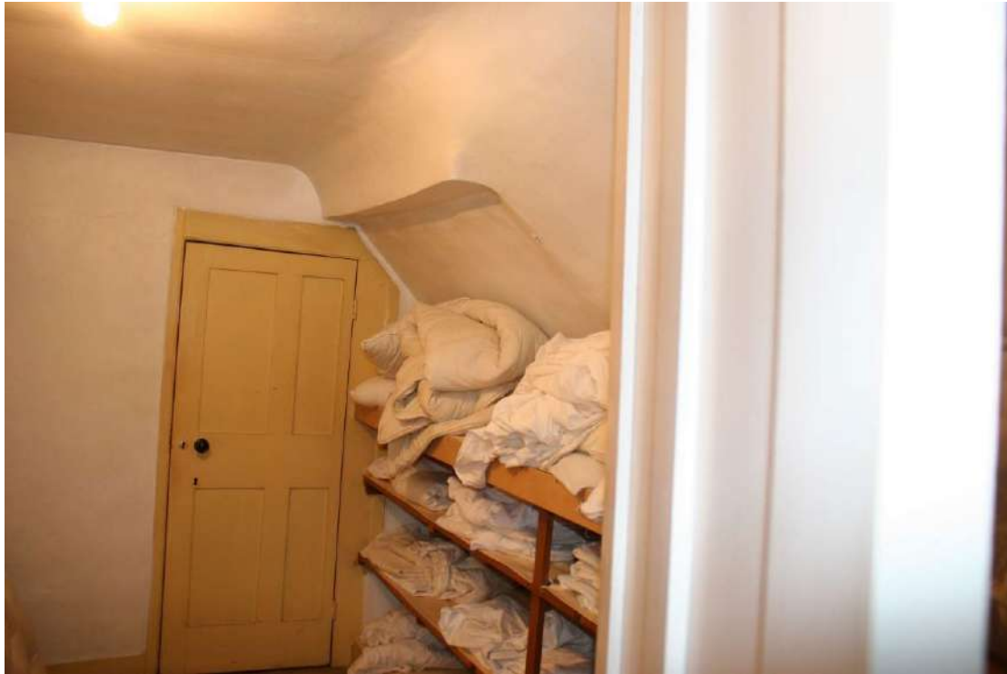
Looking N in the Linen Room.
