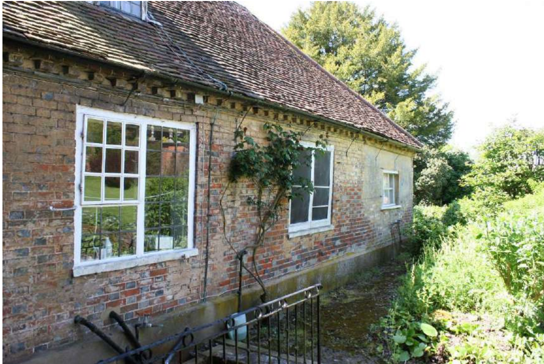
MC20th fenestration. Note the chequerwork was hidden by thick layers of limewash.
