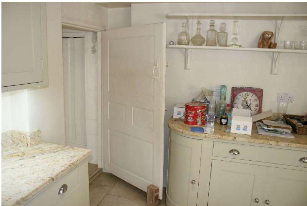
Looking NE in the Kitchen at the door to corridor. Obverse side.
