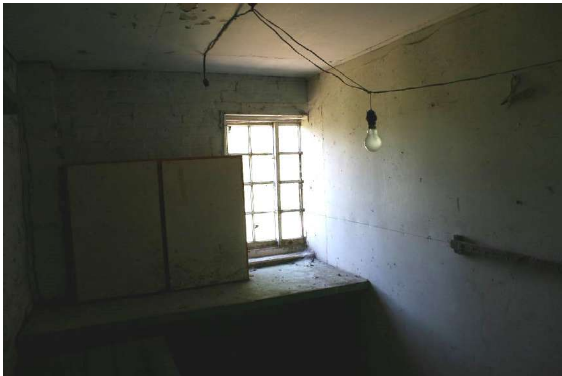
Looking N in the workshop. The partition wall meets the centre of the window.
