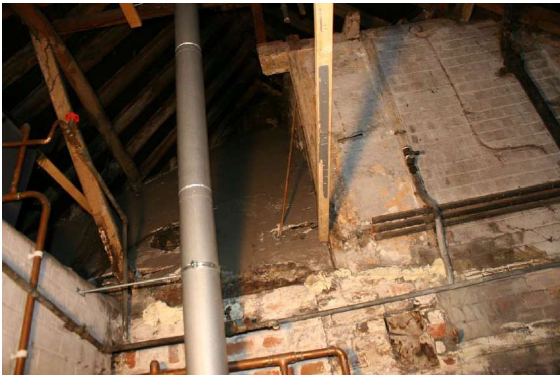
The chimney for the 1939 boiler has been taken down and new flue added.
