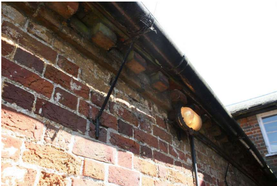
Detail of the brickwork and modillion cornice.
