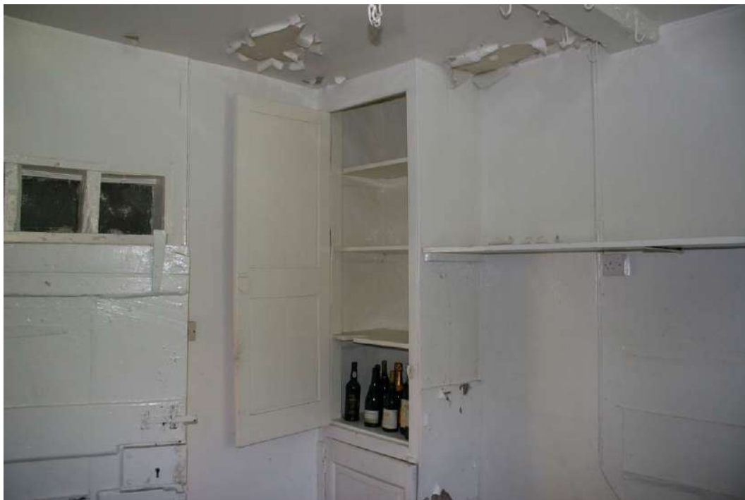
MC20th cabinets from the 1939 works.
