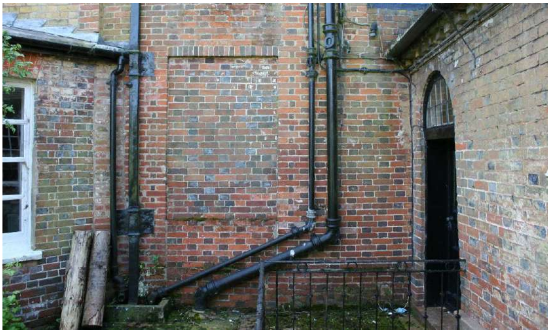
Doorway blanked off in two episodes, first to a window and now the Dining Room wall.
