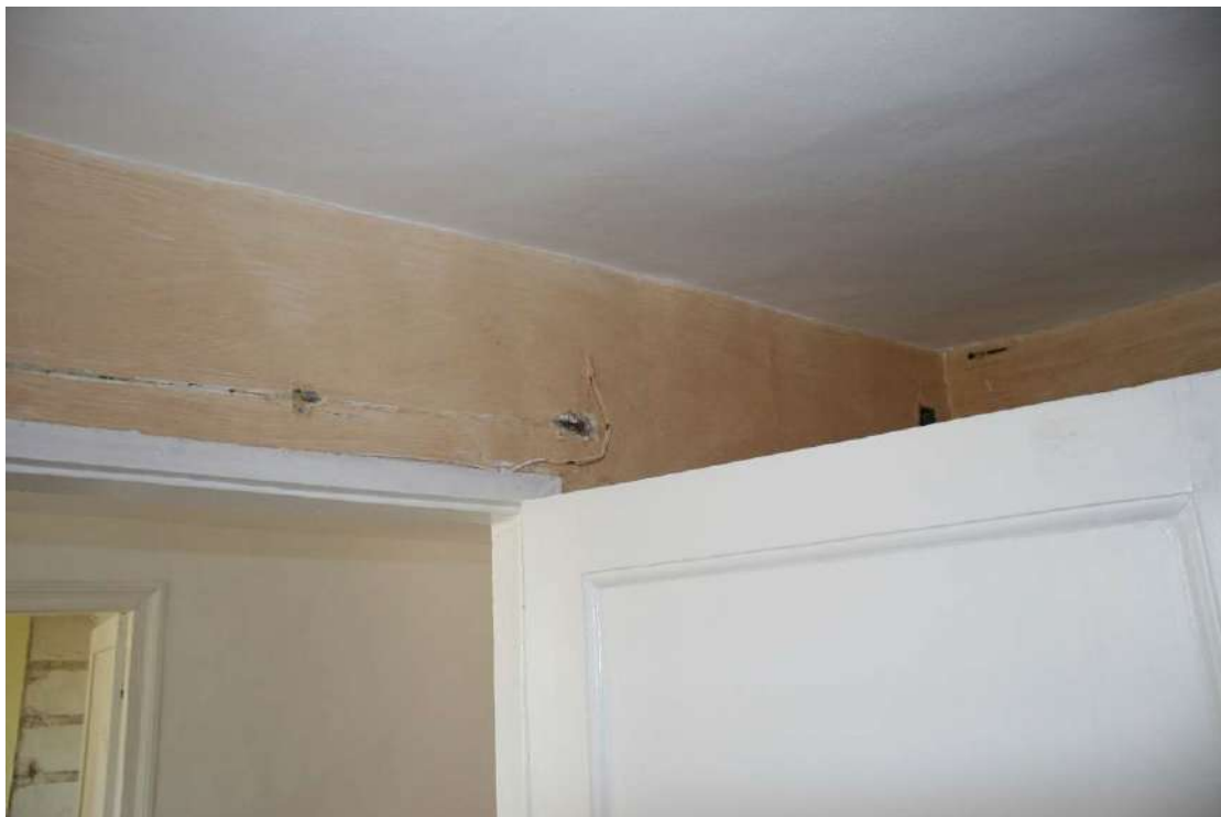
Looking at the SE corner where the old bell pull wires ran.
