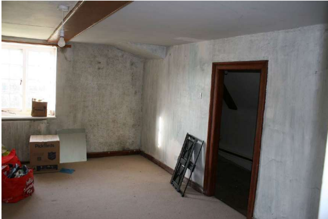
Looking N in Room 3.
