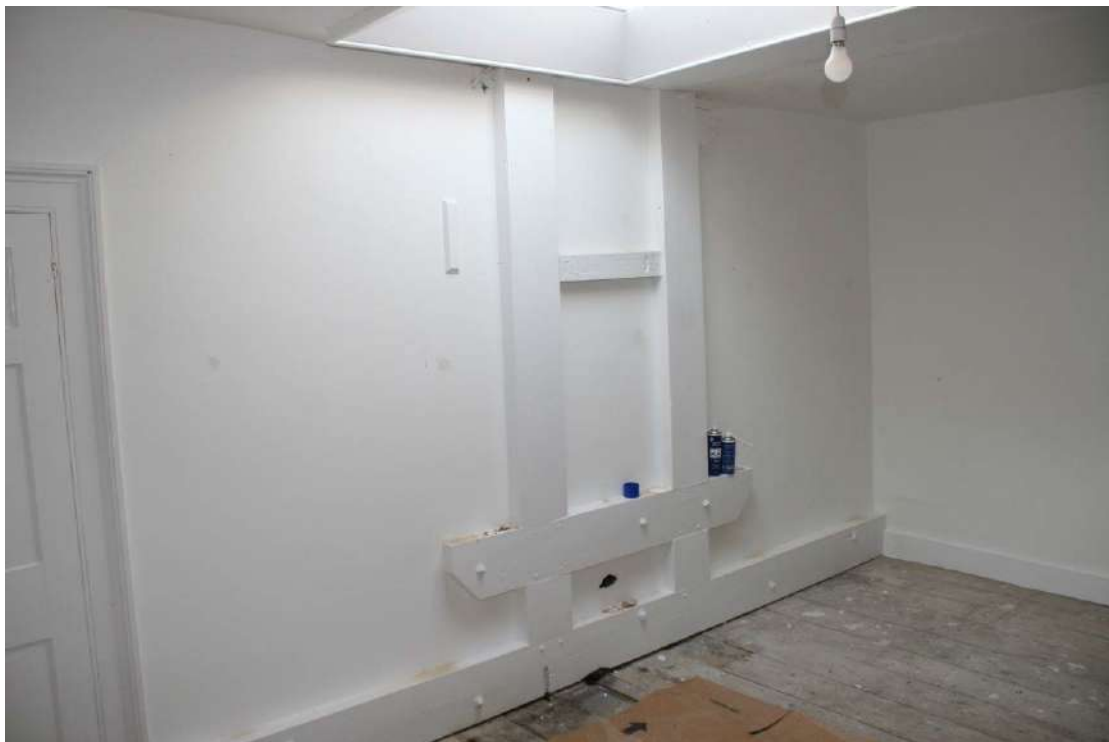
Looking NE in Room 6. The cradle supports the 1939 clock tower.
