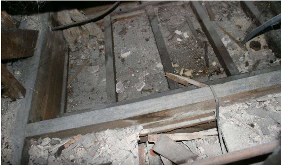
Detail of the machined softwood joists behind the studwork walls.
