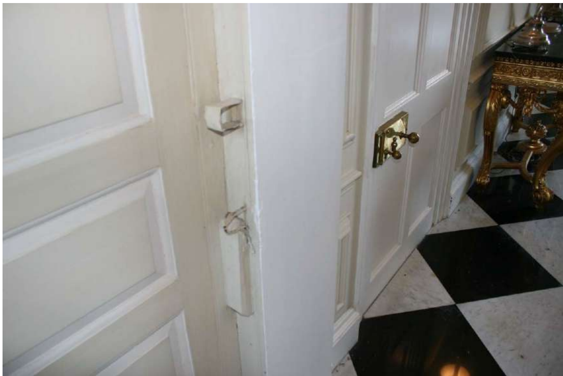
Hasp for a door bar and catch for a Suffolk latch.
