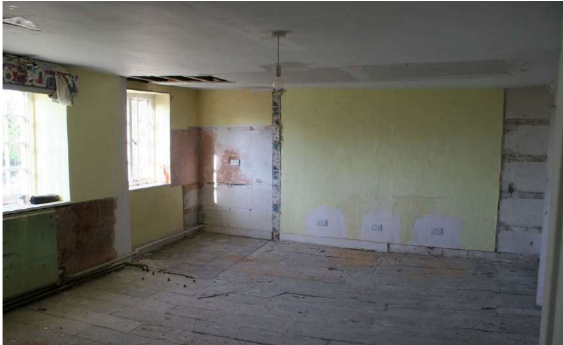
Looking E in Room 2.
