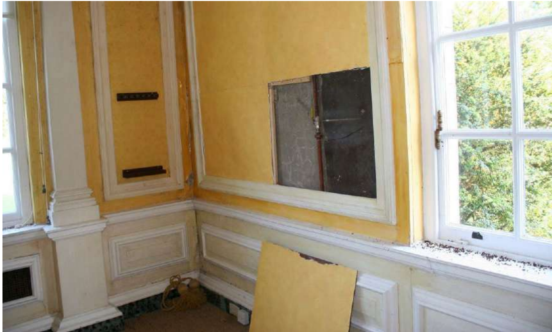
Removed panel in the SE corner.
