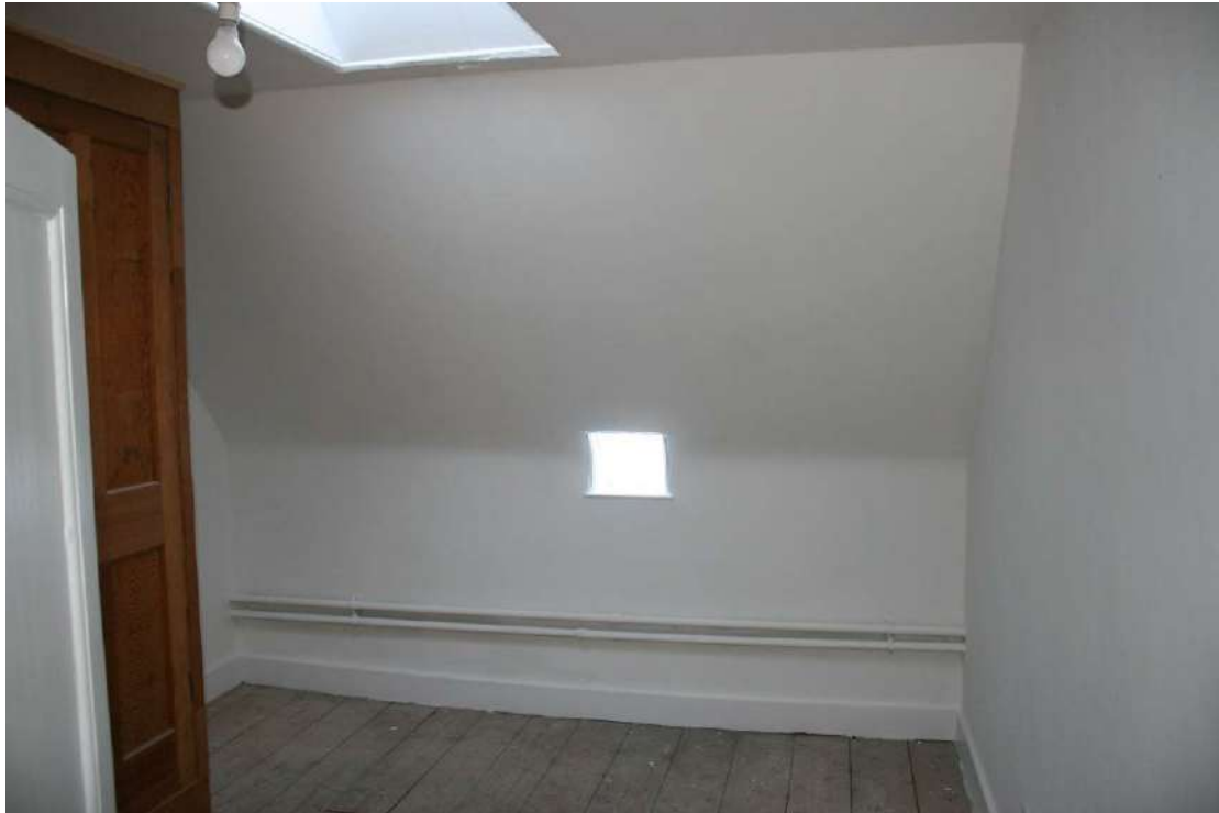
Looking S in Room 5.
