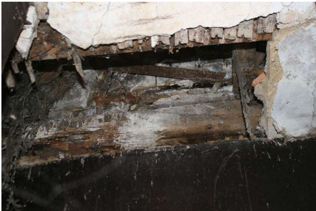
A fragment of the earlier lath and plaster panels above the shelves.
