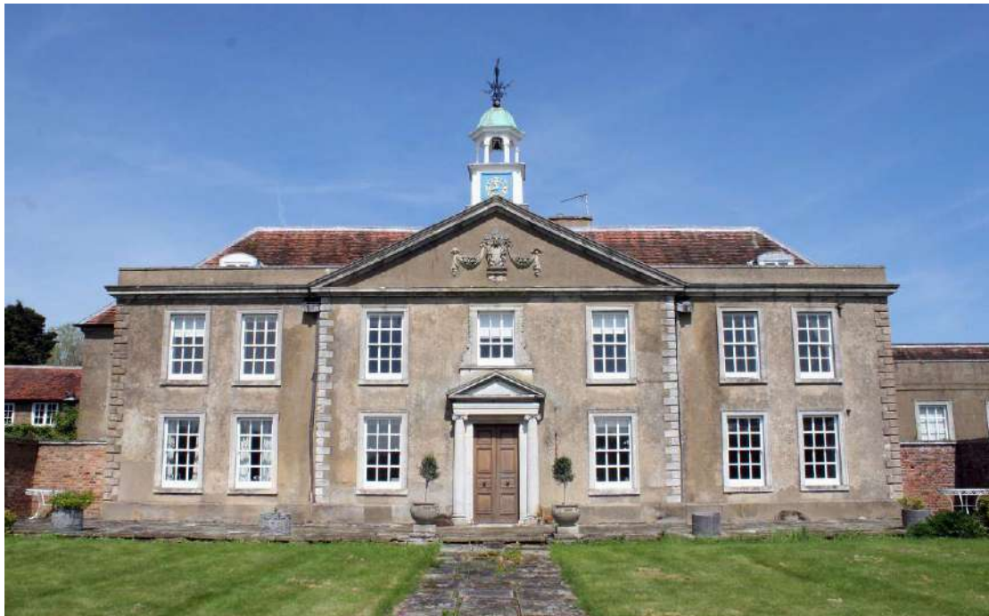
The south elevation from the gates.
