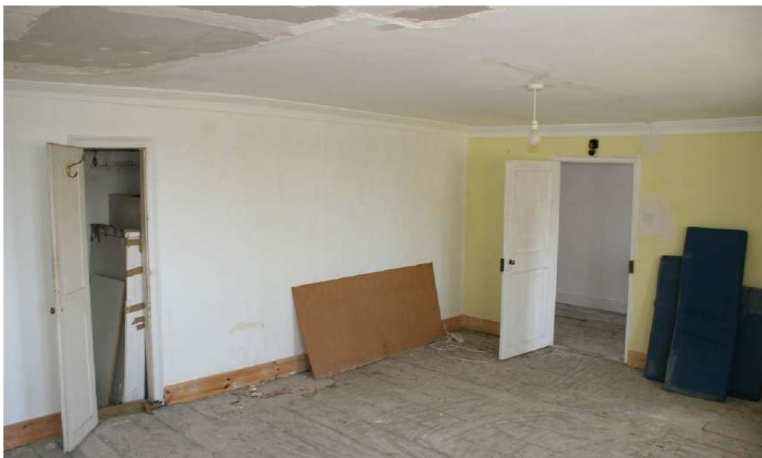
Looking SW in Room 2.
