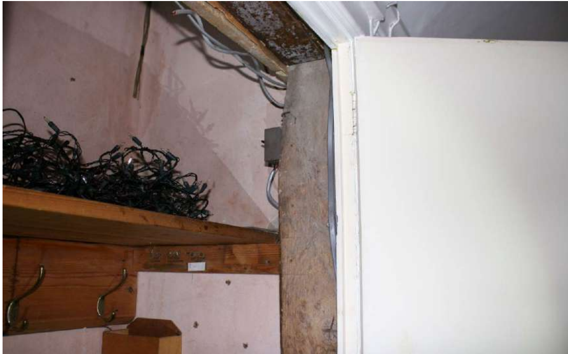
Older timber post inside the closets.
