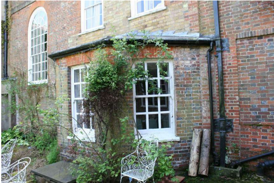
Victorian style canted bay window for the Dining Room. Note gault brickwork above.
