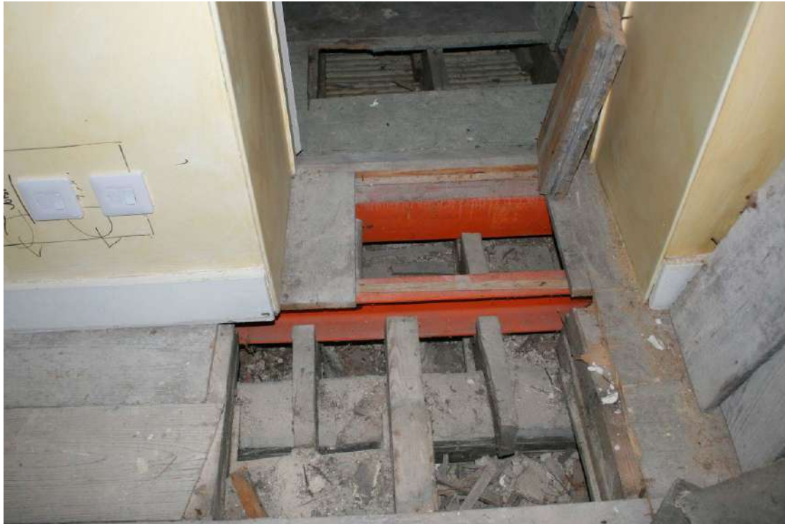
C20th steel joists parallel to a large oak joist.
