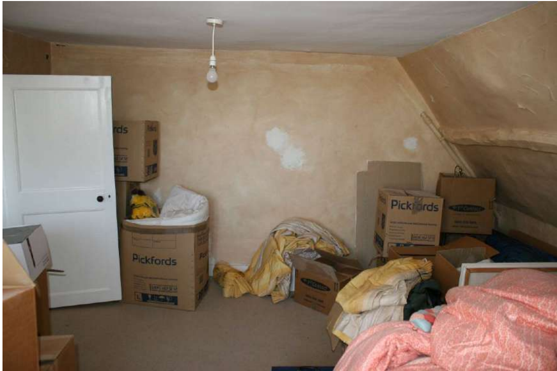
Looking S in Room 1.
