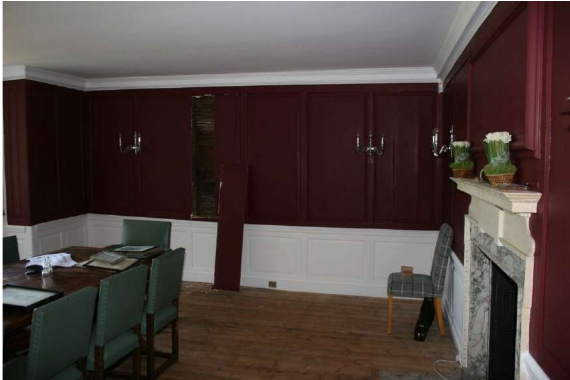
Looking E in the Dining Room. A panel has been removed.
