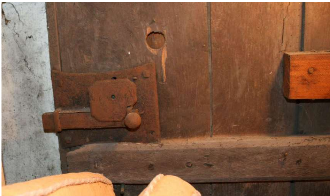
Detail of the bolt on the vertically boarded door.
