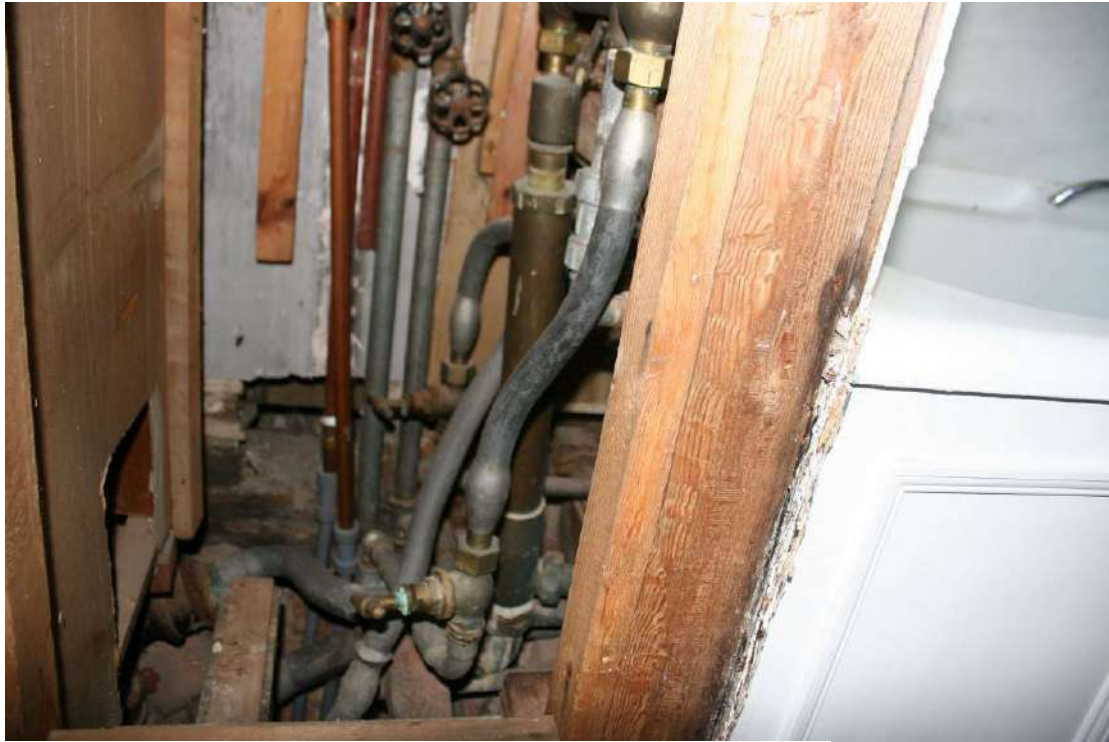
The plywood and softwood timber carcase hiding the 1939 plumbing.
