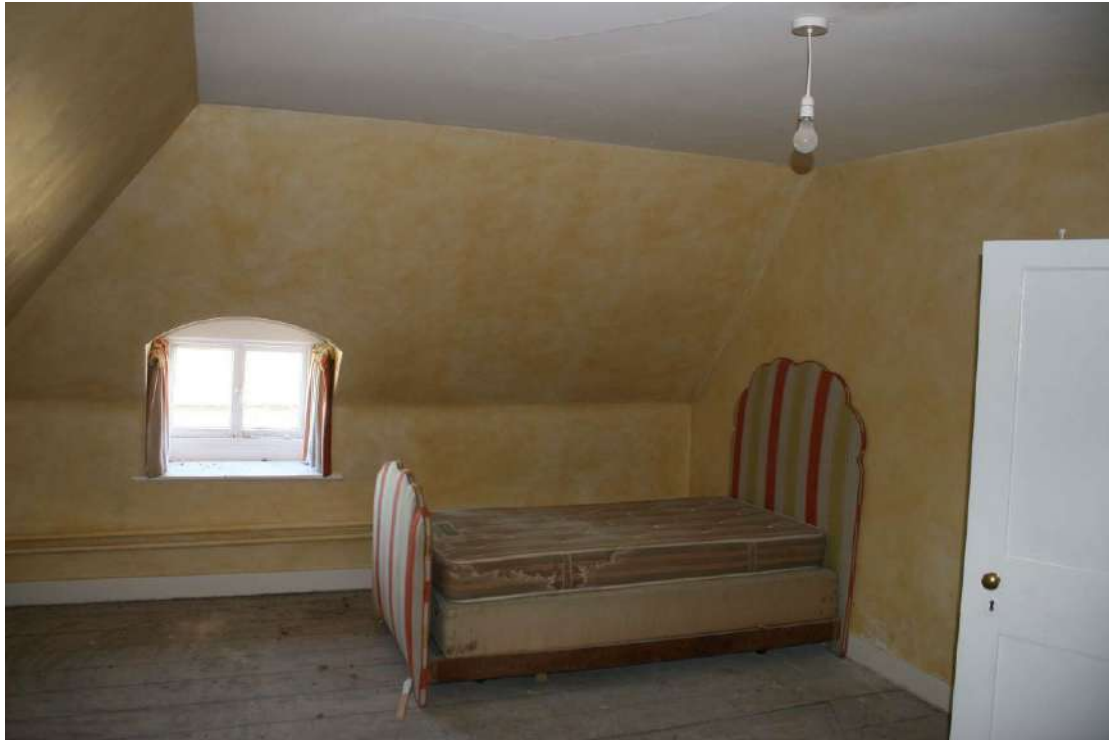
Looking S in Room 4.
