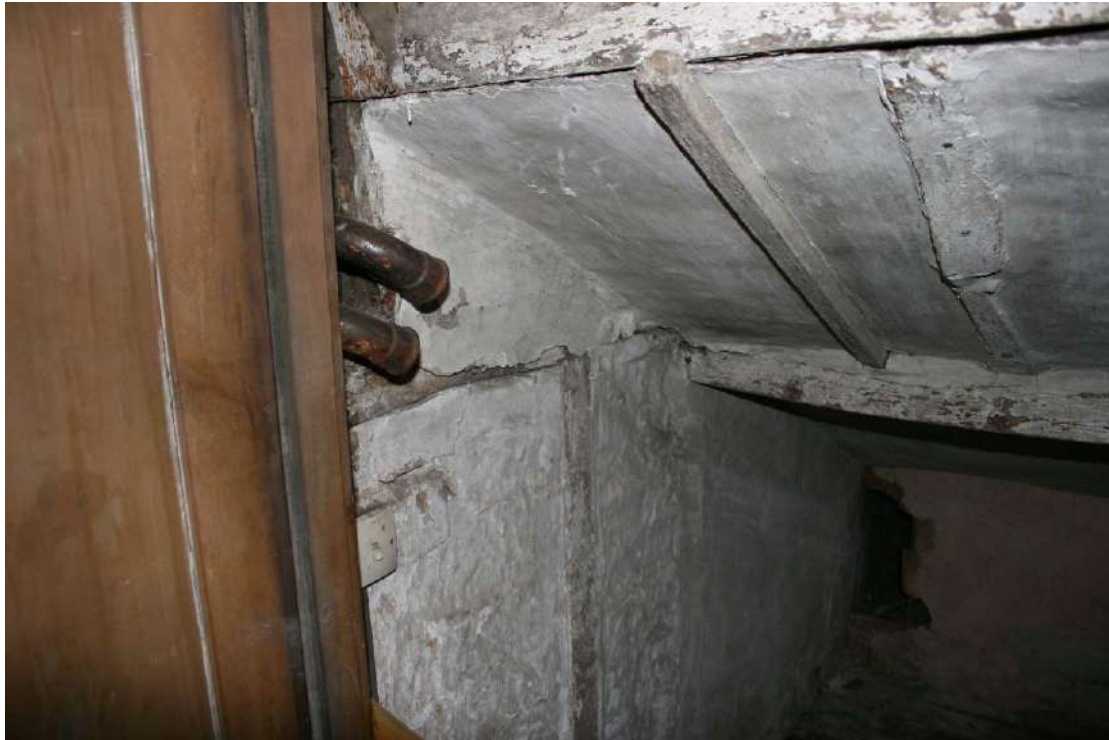
The soffit of the West Staircase. Looking SE.
