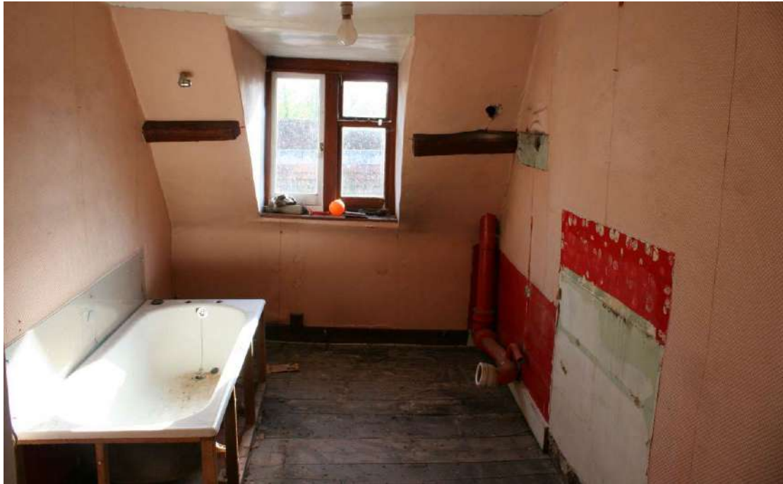
Looking W in Room 9.
