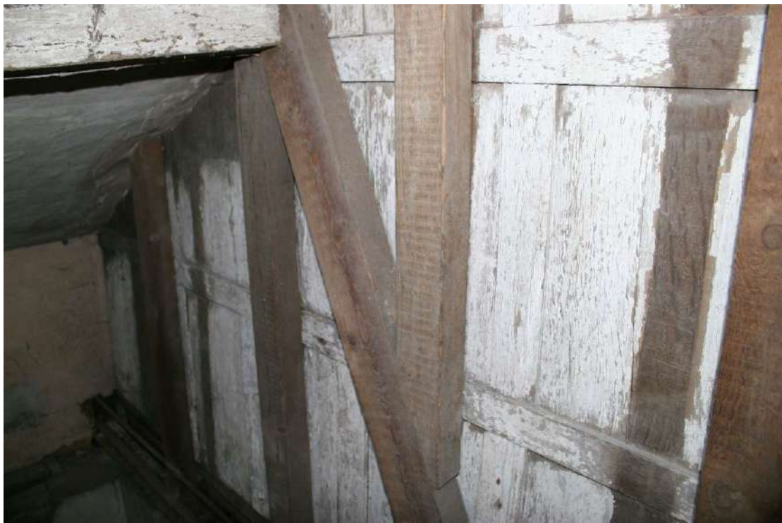
The back of the West Staircase panelling with C20th reinforcements to the staircase.
