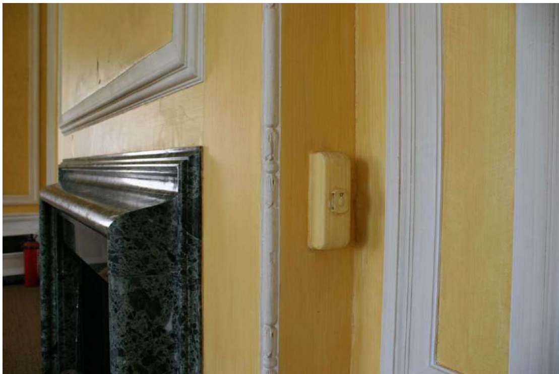
Detail of the fire surround, moulded beads and architraves. Central heating control.
