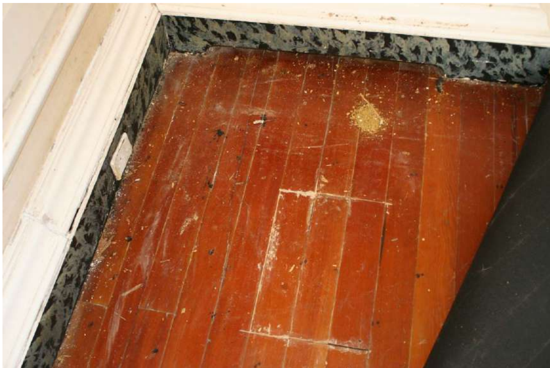
Detail of the suspended pine floor.
