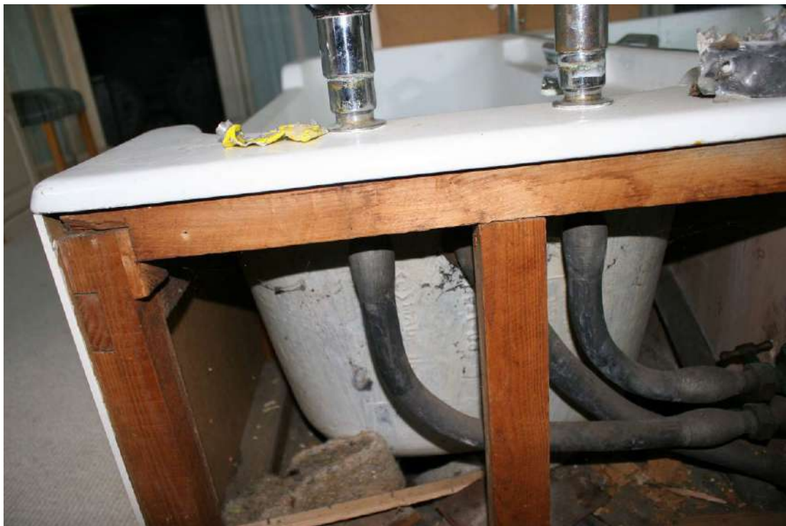
Machined softwood carcase for the cast iron bath.
