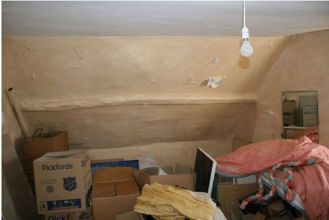
Looking W in Room 1.
