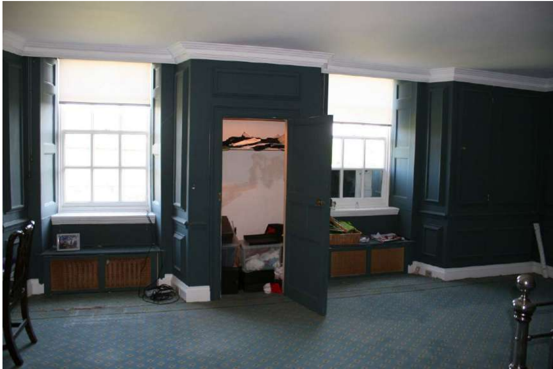
Looking S in Bedroom 2. The radiators are in the window seats.
