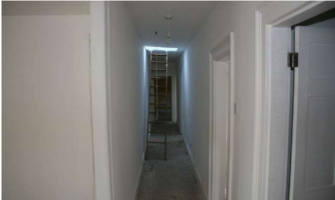
Looking E in the corridor.
