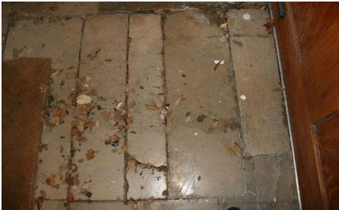
The worn stone threshold by the west door.
