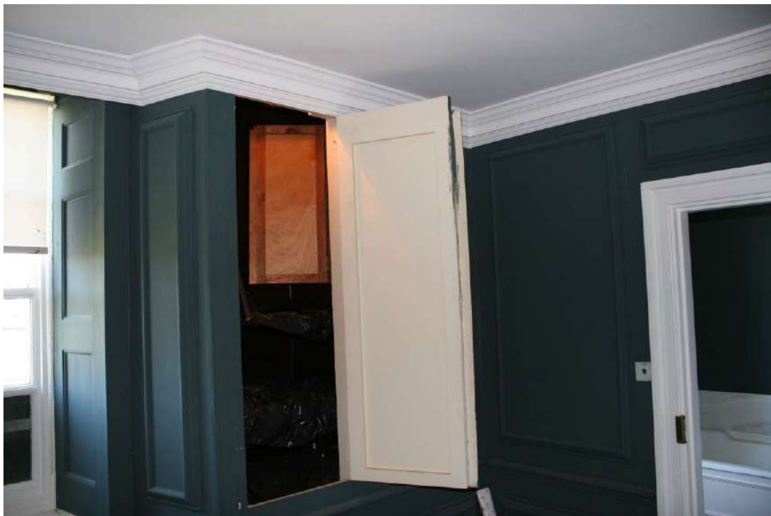
Closet containing the water cistern for the WC in Bathroom 2.
