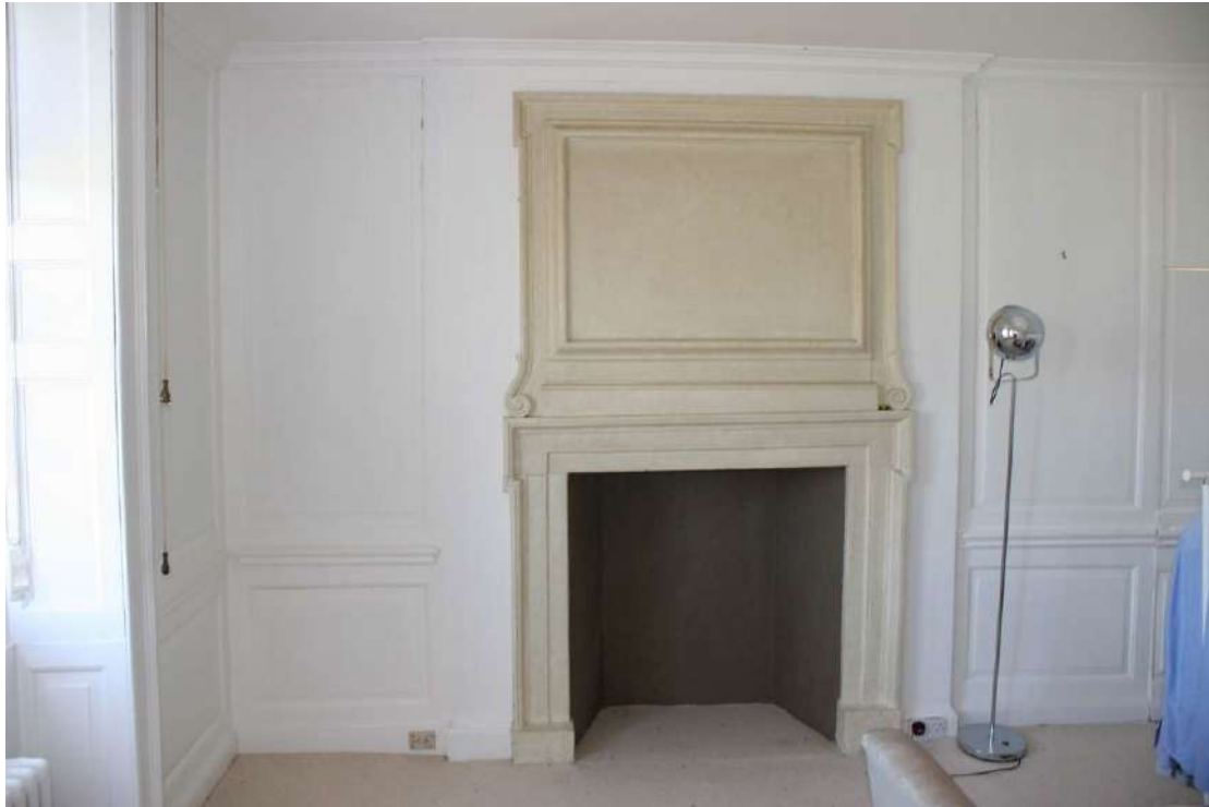
The fire surround and overmantel is resin fake.
