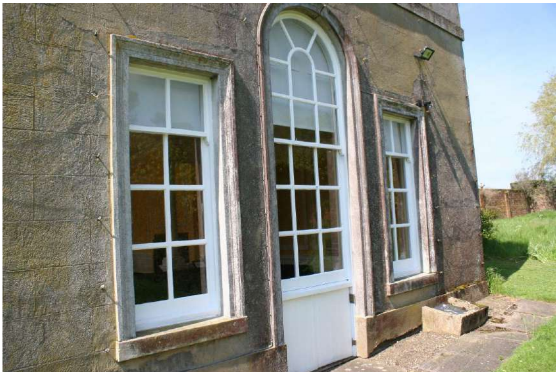
The windows and half door on the east elevation.
