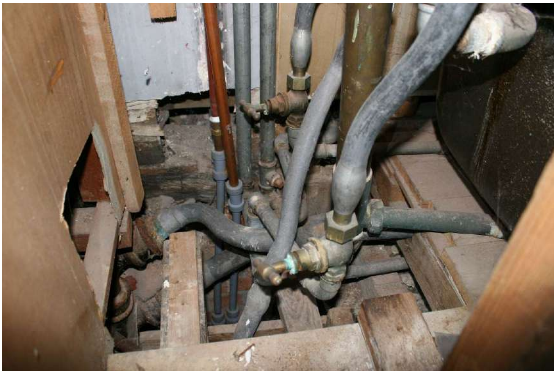
Detail of the leadwork pipes.
