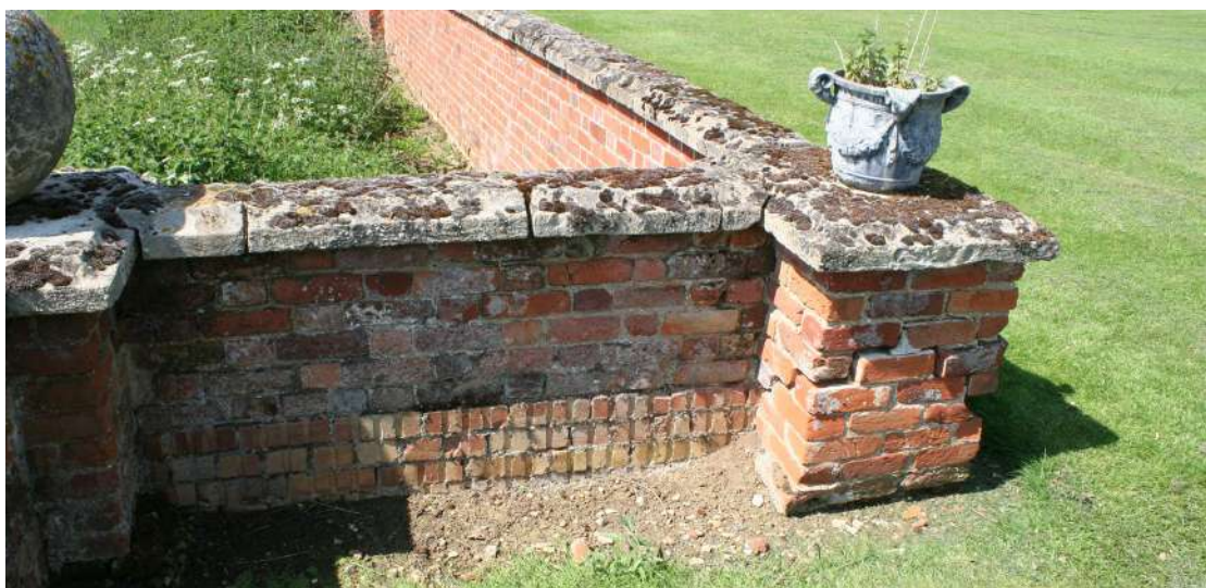
Detail of the Fletton brickwork.
