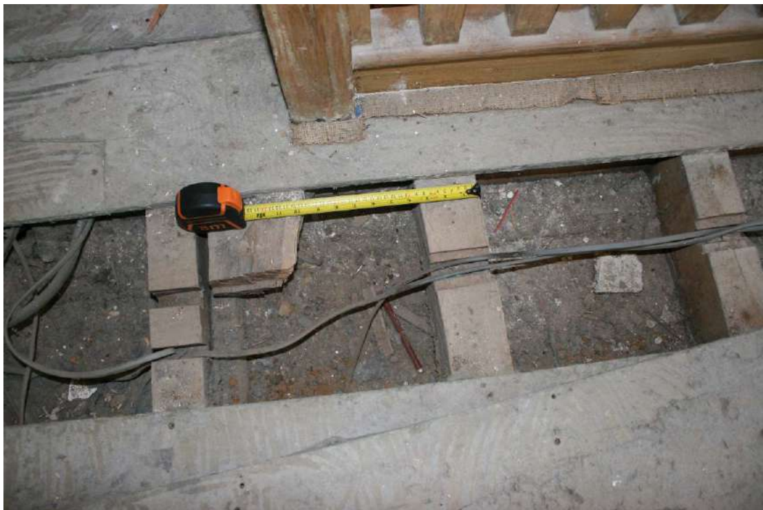
Detail of the floor joists on the Attic Landing.
