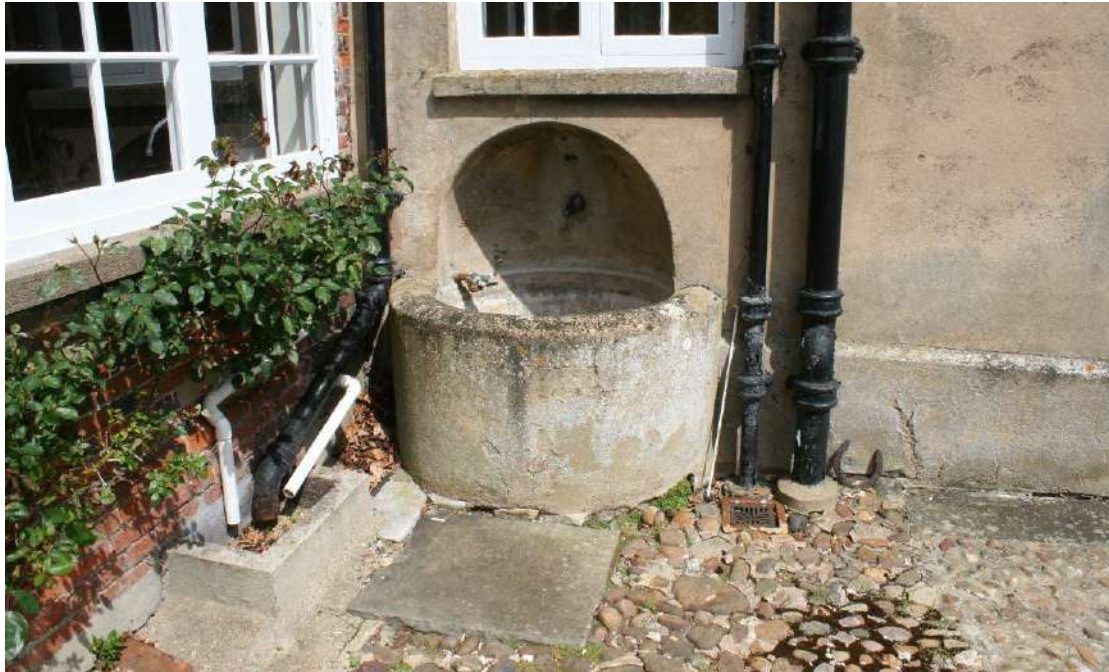
The water cistern on the west elevation.
