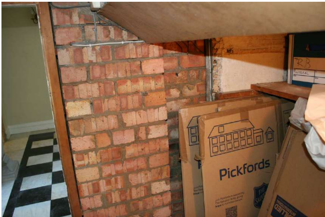
Looking E in the Store. The Atrium wall is made from Flettons set in cement.
