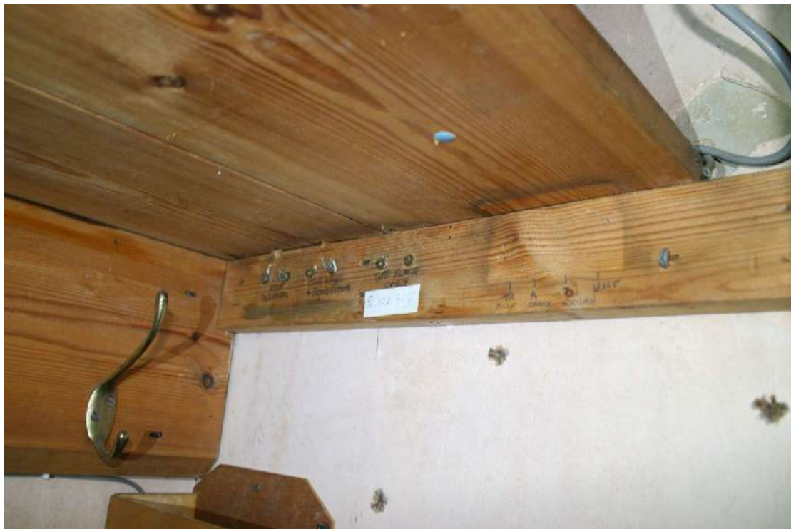
Detail of the construction of the closets with 1939 period electrical terminals.
