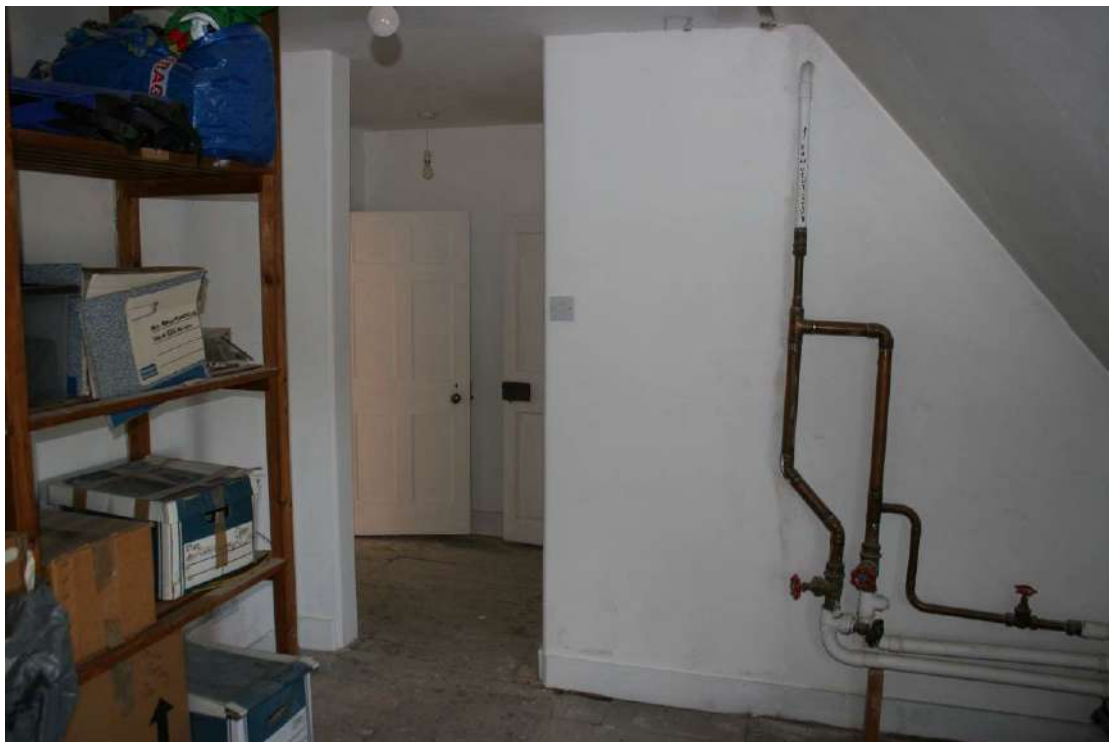
Looking NE in Room 8.
