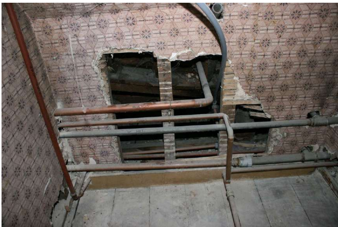
Detail of the LC20th and C21st pipework and MC20th studs and lath and plaster.
