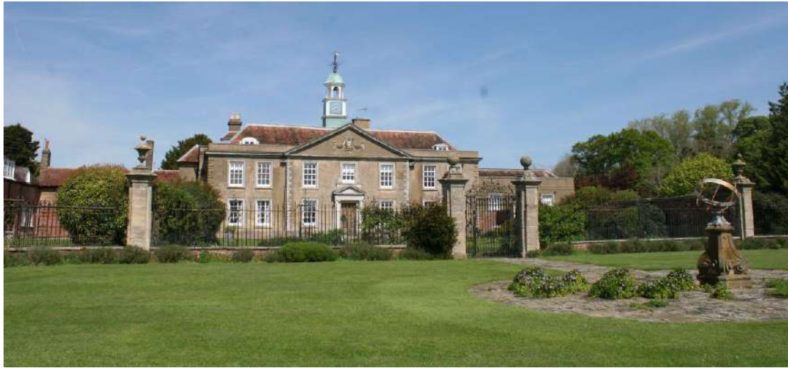
The south elevation from the terrace.
