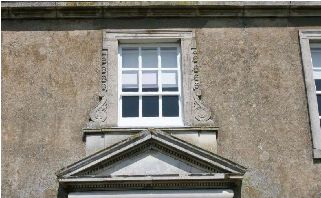
Detail of the horned sash window above the porch.
