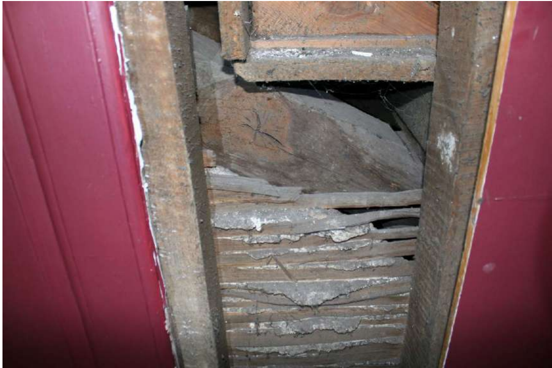
Detail of the bearer for the East Staircase and older riven laths.
