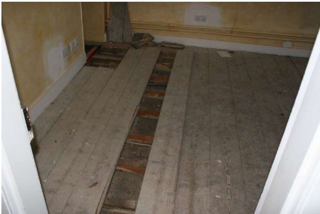
Looking E in Room 4.
