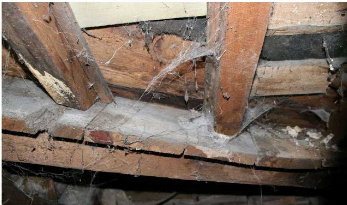
Detail of the roof structure with C20th red bracking marks.
