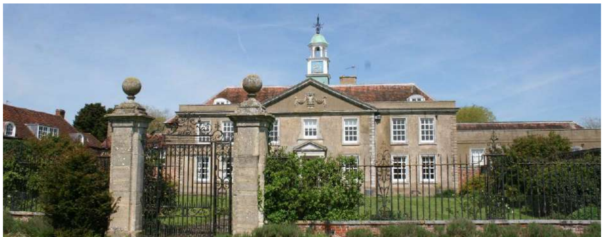
BJHC. 08 05 2024. Entrance gates and clair-voie
