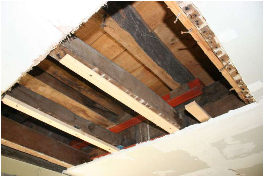
The ceiling has been repaired and has plasterboard sheets.
