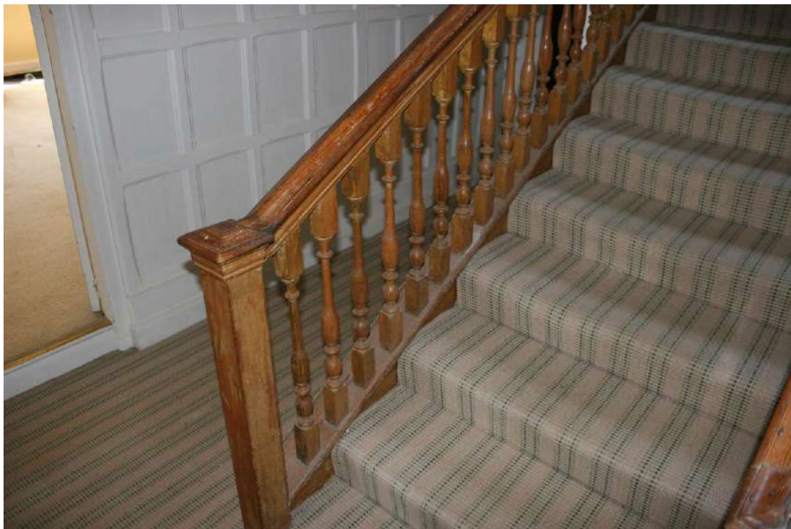
Detail of the newel post and spindles.
