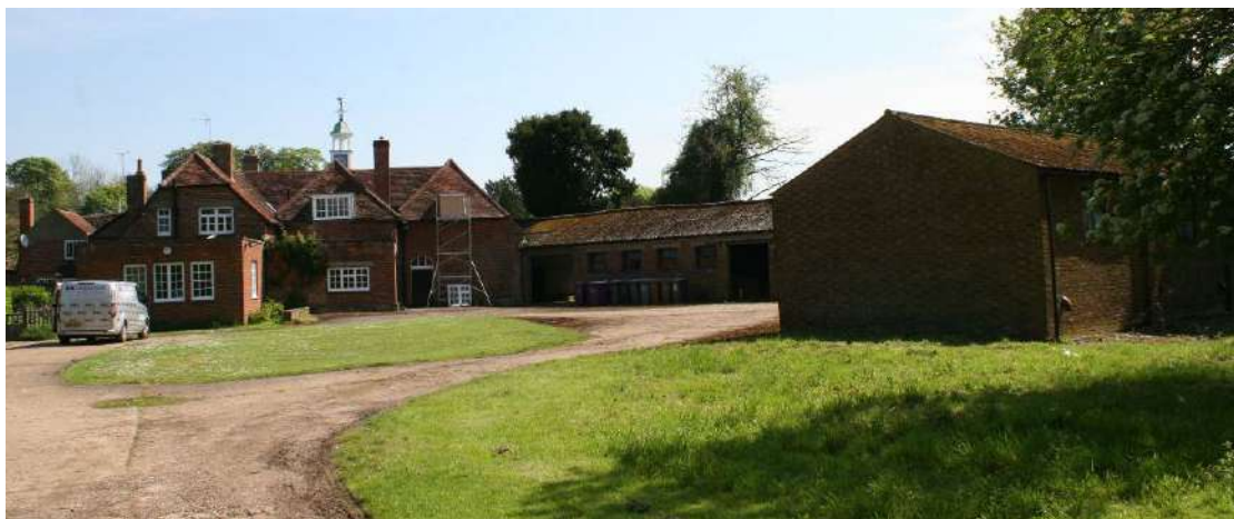
The Outbuildings looking from the west near the pond.
