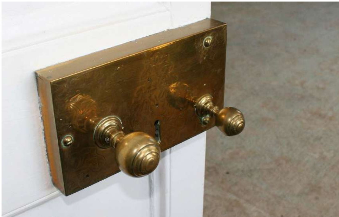
Detail of the lock box to the Library.
