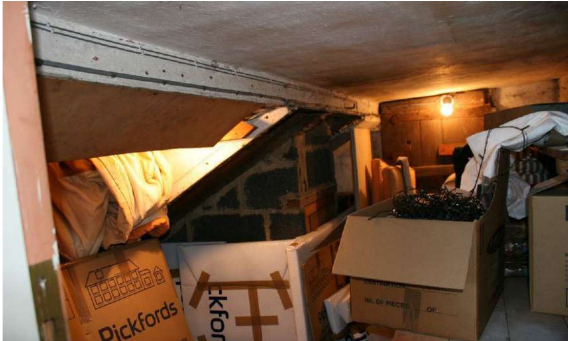
Looking W in the Store. Note the blockwork insertion and the very old door.
