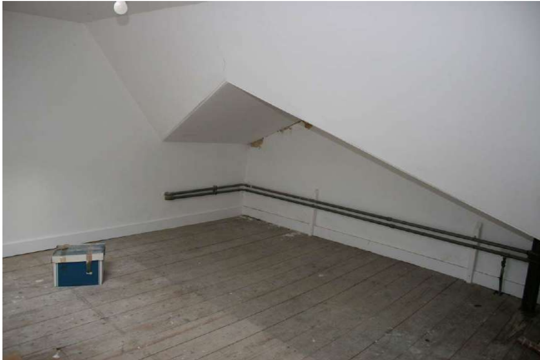
Looking SE in Room 6.
