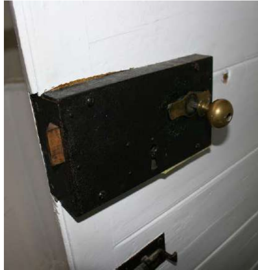
The inner door has been plated over to look Georgian. Detail of the cast iron lock box.
