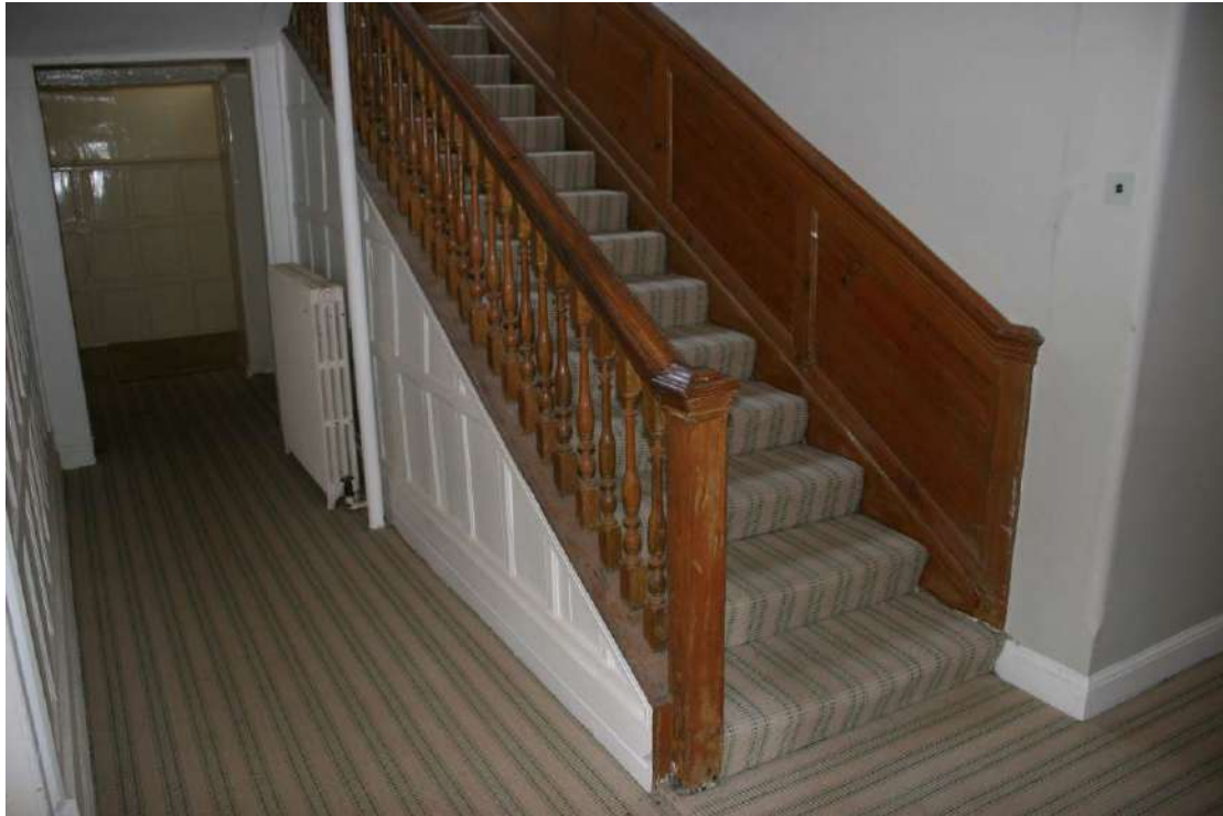
Looking N at the West Staircase.
