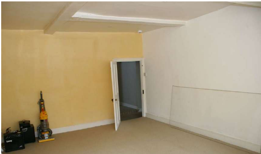
Looking SE in the Servant's Hall. Note the ceiling beams.
