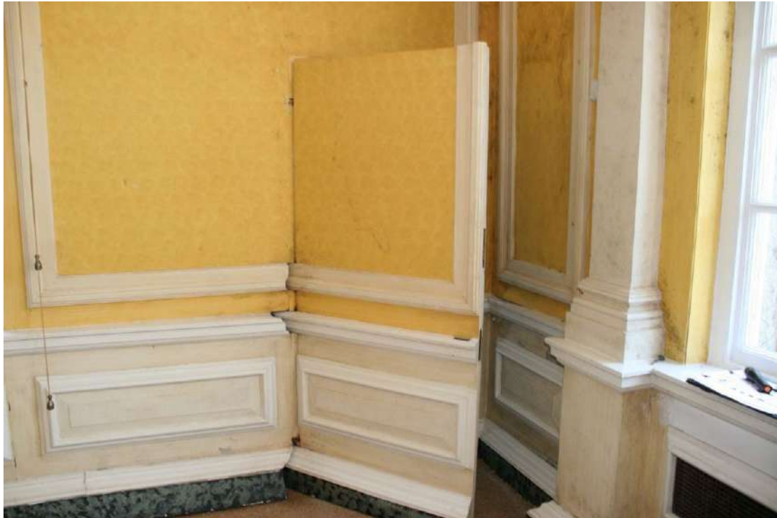
The entrance door is disguised as part of the panelling.
