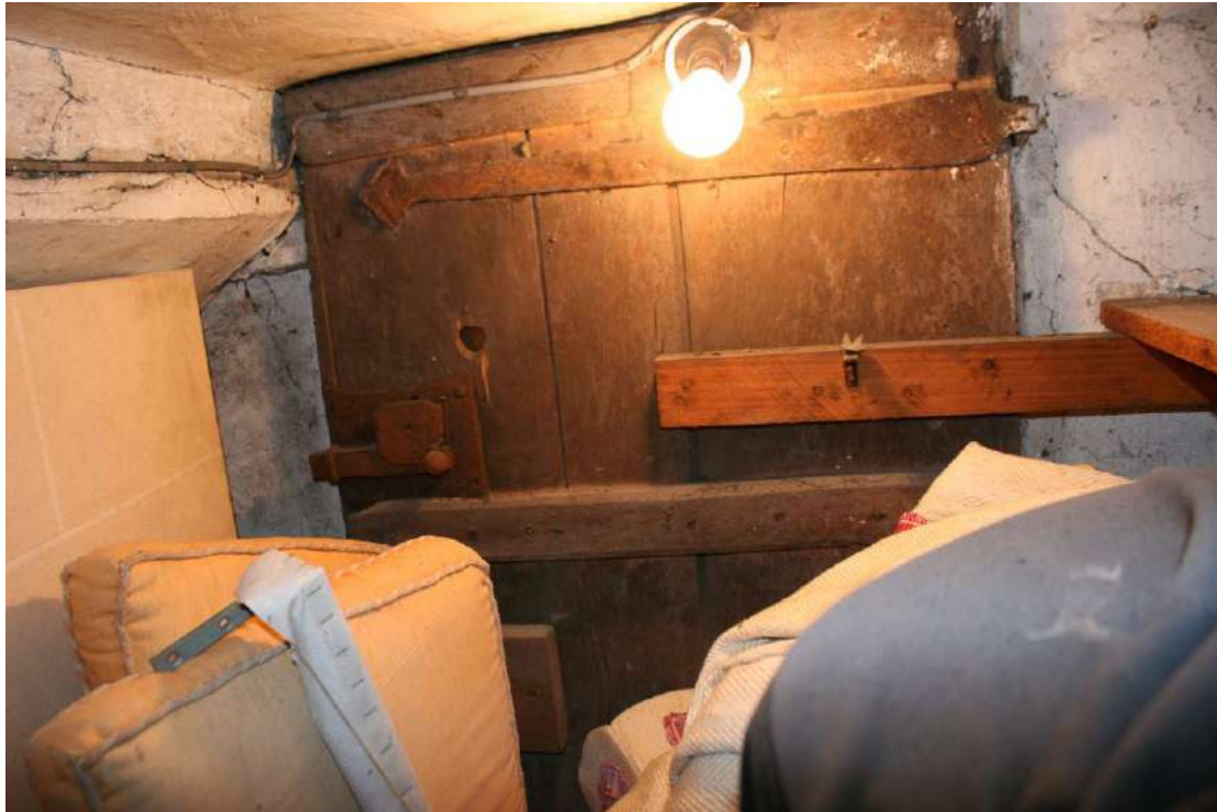
The upper part of the vertically boarded door in the Store.
