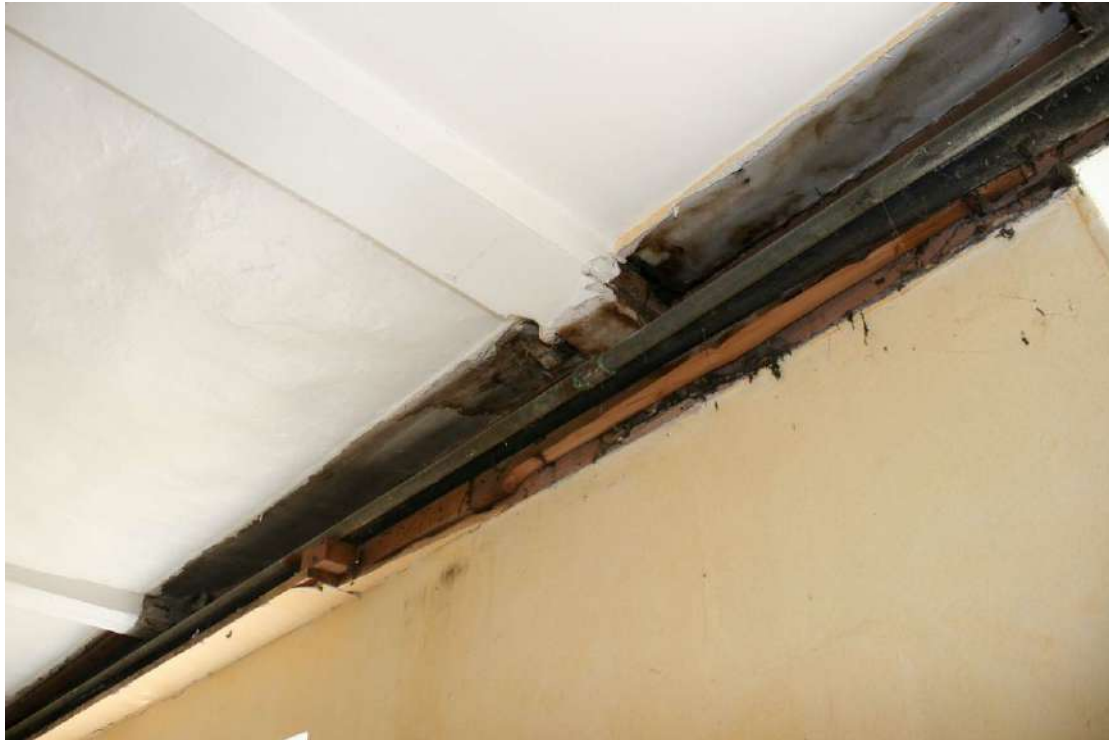
Detail of one of the boxes containing the 1939 plumbing.
