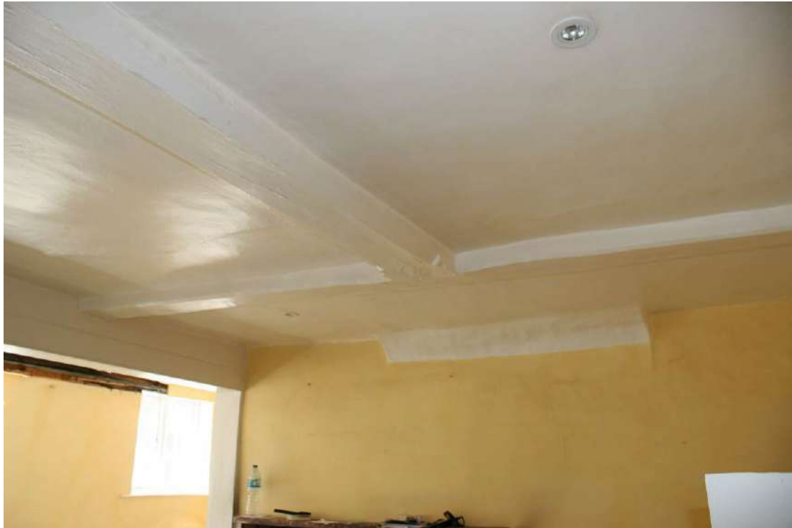
Looking NW at the axial main joist and bridging joist for the firestack bay.
