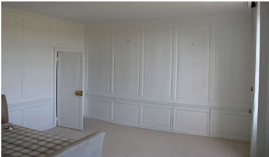
Looking E in Bedroom 3.
