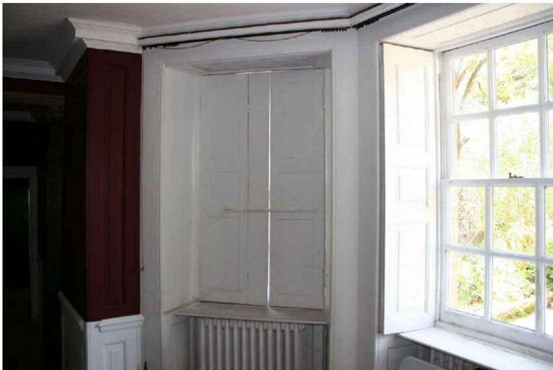
Detail of the shutter in the Dining Room Bay window.
