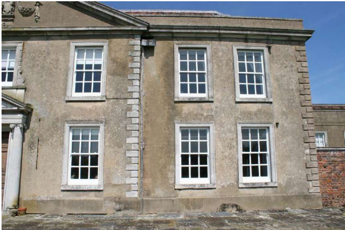
Detail of the eastern half of the south elevation.
