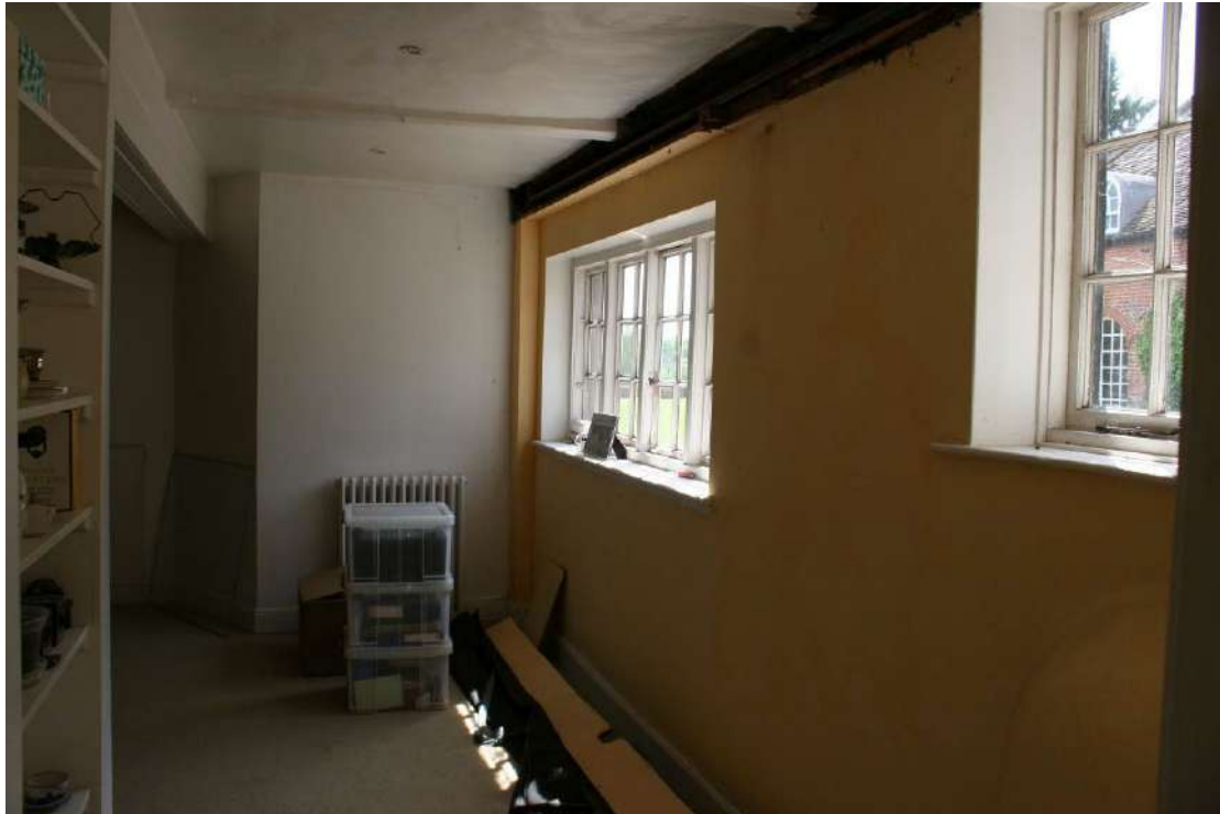
Looking S in the Servant's Hall from the Kitchen.
