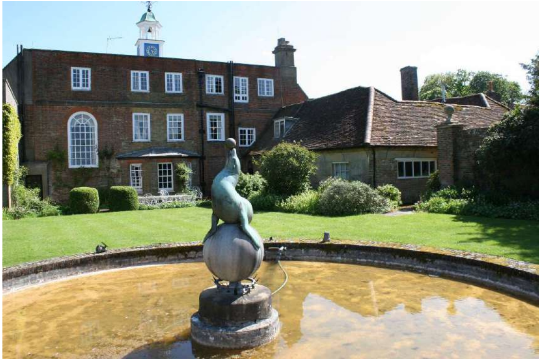
The north elevation of the House.
