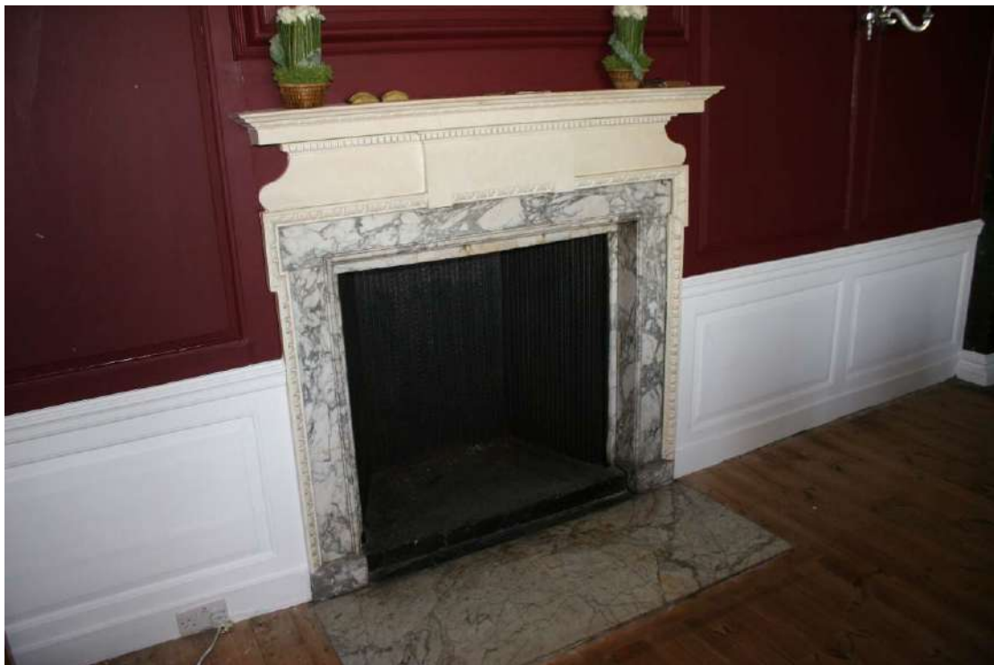
Detail of the marble fire surround and timber mantel shelf.
