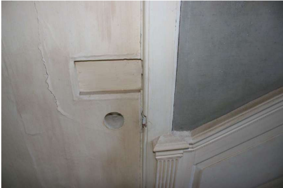
Recesses in the wall for the lock box and knob for the folding doors. (Now removed).
