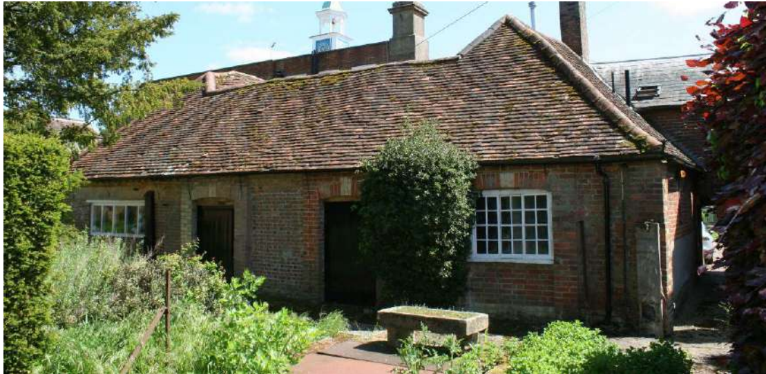
North elevation of the Kitchen.
