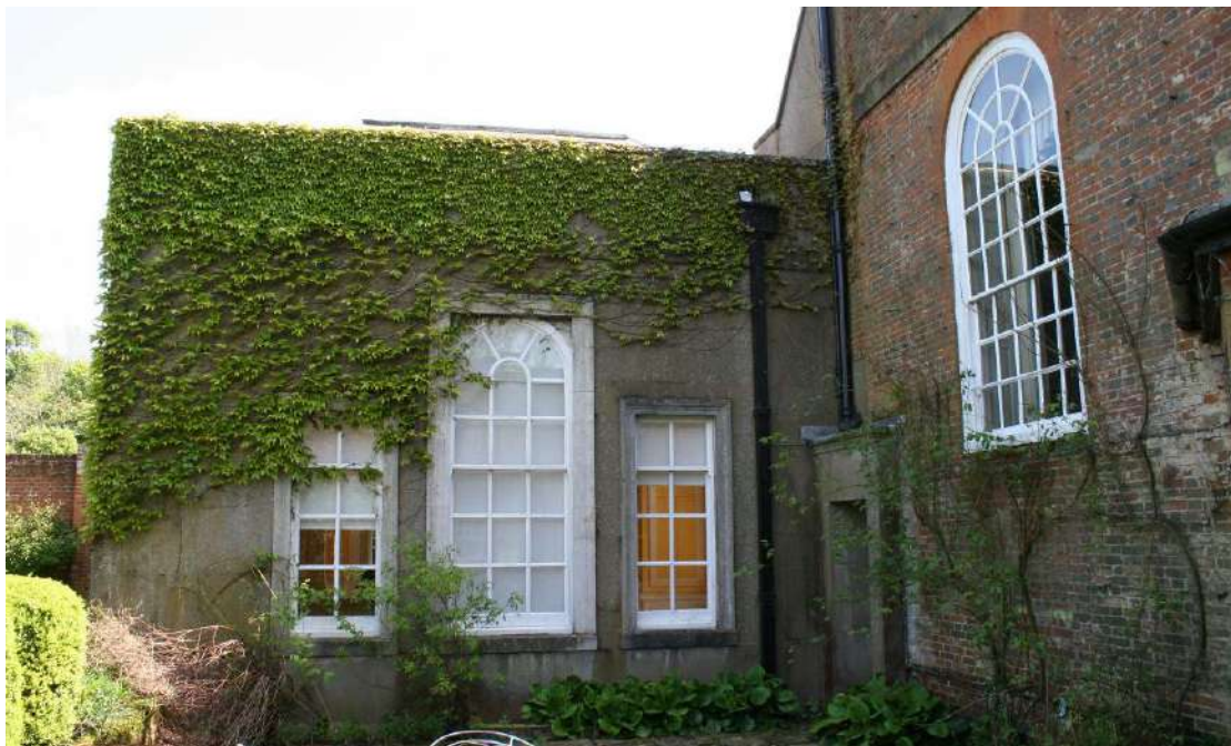
1939 inserted arch headed window is part of a suite used in the Music Room.
