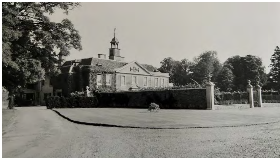
The driveway following the renovation works by Colonel Cooper
