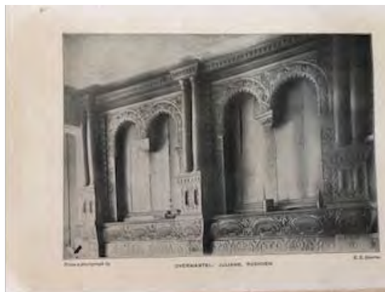
C17th overmantel (refer to Historic Building Recording)
