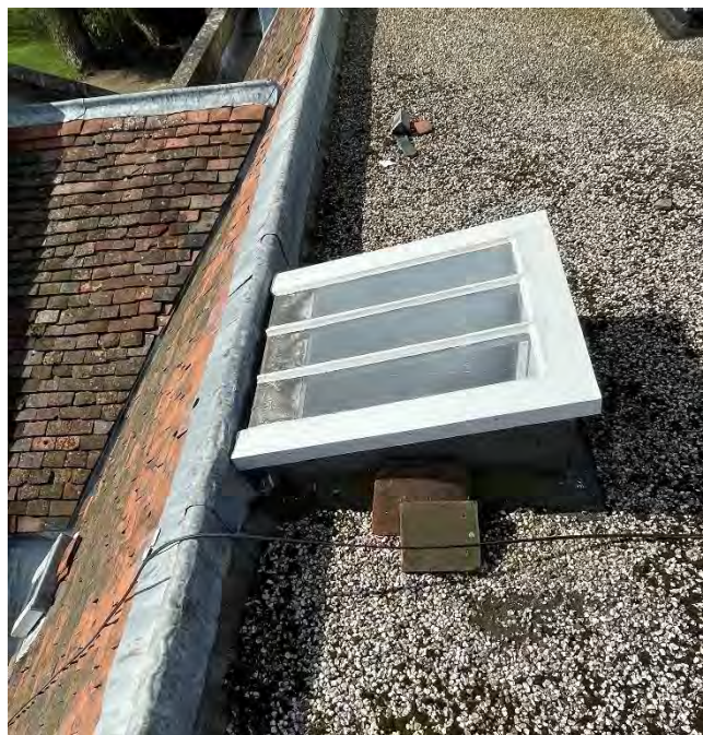
Rooflight R3 located against upstand kerb
