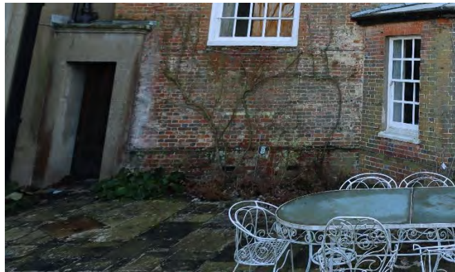
Location of infilled window at low-level
