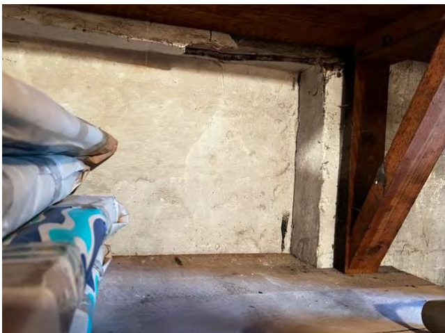
Evidence of infilled window from internal side of redundant service corridor
