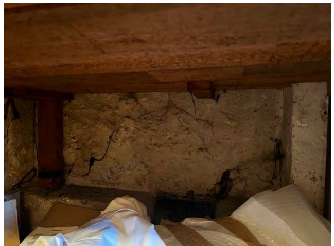
Evidence of infilled window from internal side of redundant service corridor
