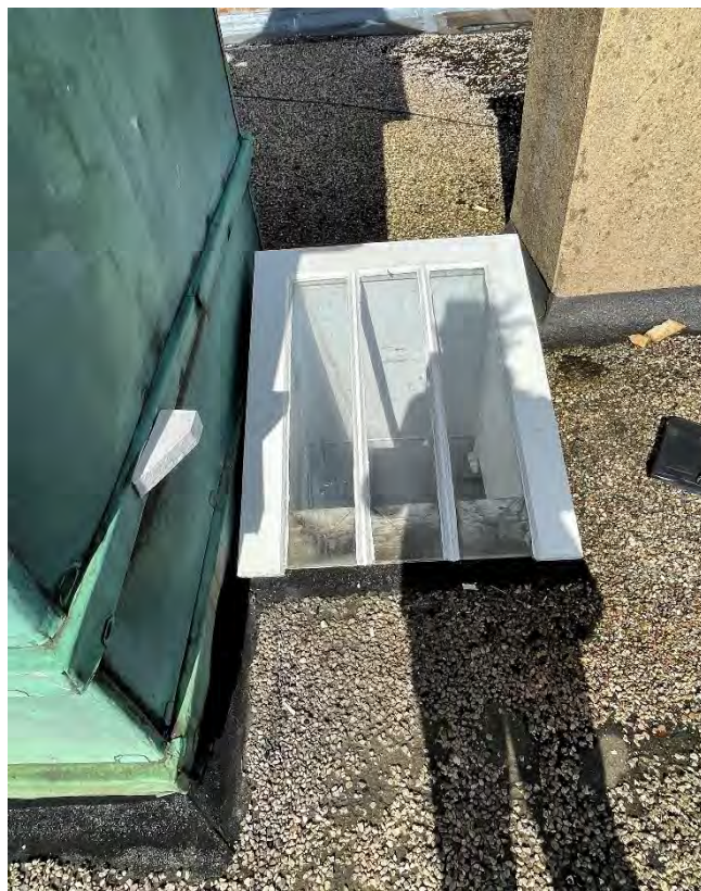
Rooflight R2 currently used for access to roof via fixed ladder in 2 nd floor corridor
