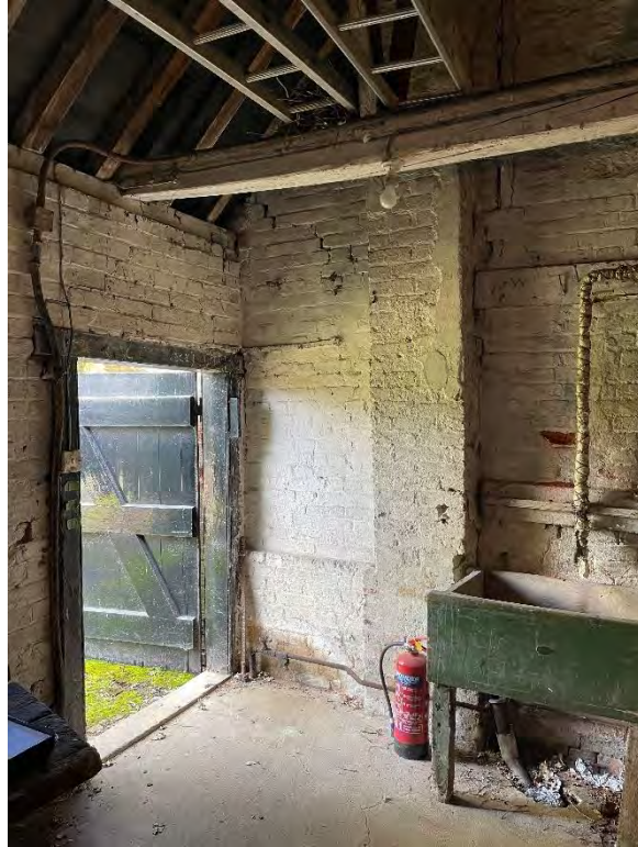
Boiler Room. Masonry flue and brick infill panel (rhs of MC20th door) to be removed
