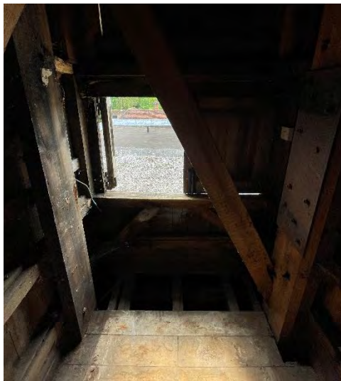
Bracing within the body of the clocktower
