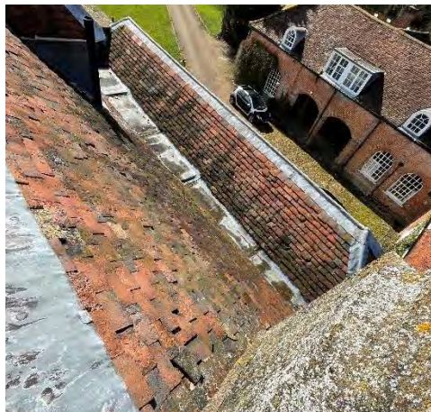
West side stepped valley gutter
