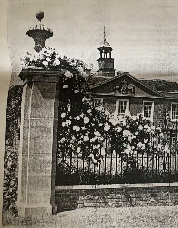
2.—ROSE ALBERTINE ON ONE OF THE FORECOURT PIERS
