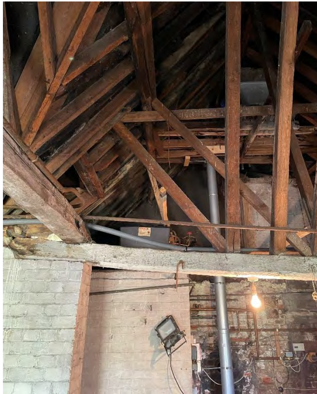
Structural solution for support of deflecting timber beam to be confirmed. MC20th corner to kitchen food cupboard behind pier
