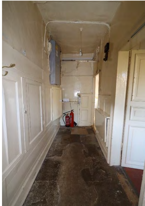
Butler's Pantry Service Corridor EC18 th reclaimed cupboard doors concealing C17 th fireplace to left side and worn flagstone floor
