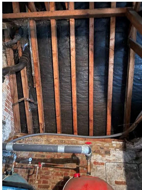
Boiler Room. West slope of roof. Machined softwood and modern sarking felt (Historic Recording P 37)
