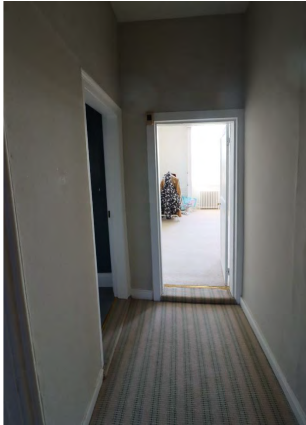
Corridor approaching Master Bedroom. Door and partition to be reinstated along line of removed partition to rhs
