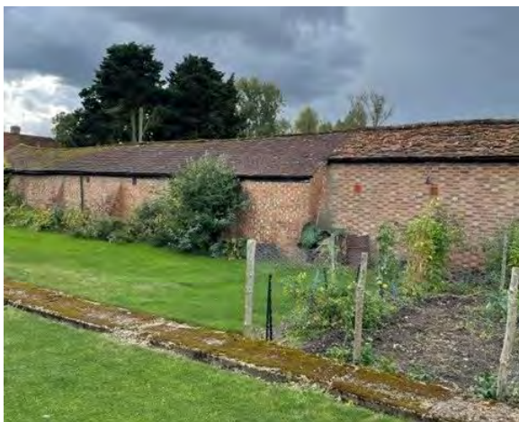
East elevation of outbuilding
