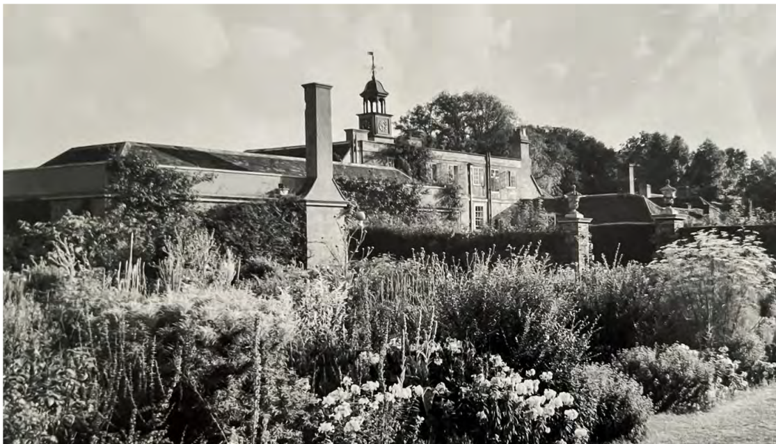
Original Music Room chimney stack
