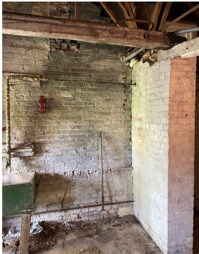
Structural solution for support of deflecting timber beam to be confirmed. MC20th corner to kitchen food cupboard behind pier
