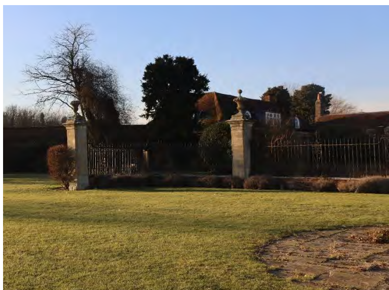
Later additions to the south wall of the Entrance Courtyard
