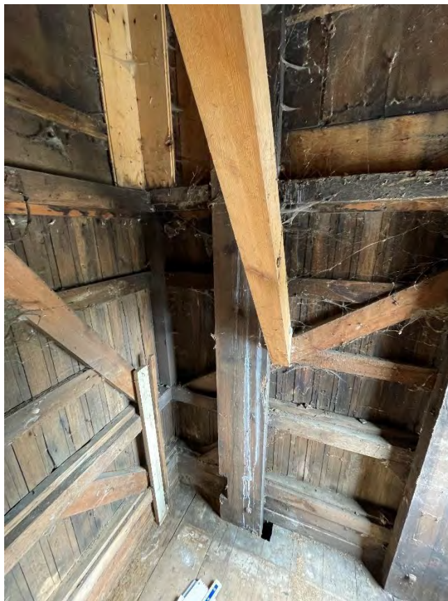
C20th bracing inside clocktower proposed to be removed to allow insertion of new ladder
