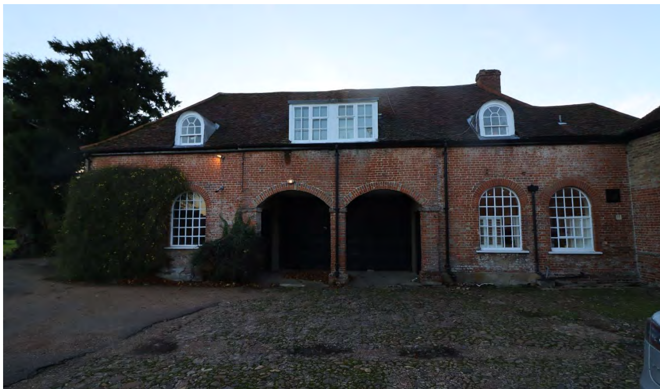
Former coach house (Home Farm) Front (East) Elevation
