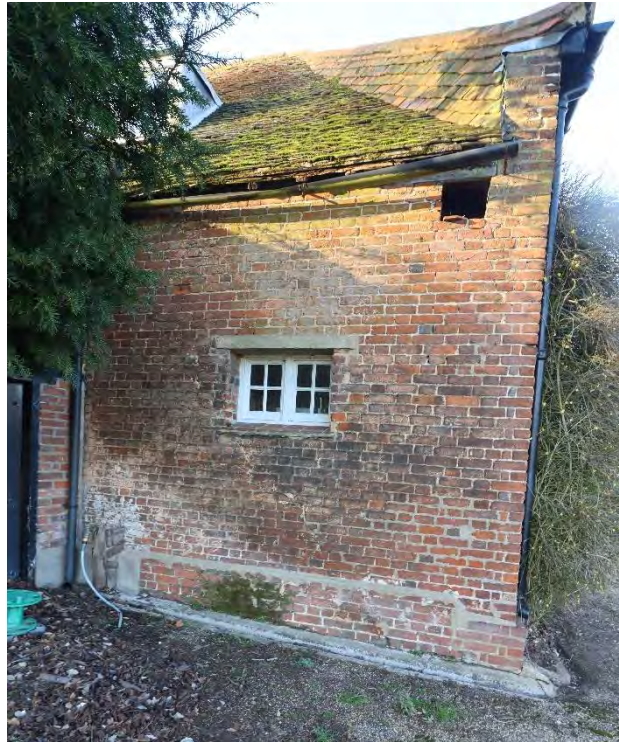
South-east corner of former Coach House
