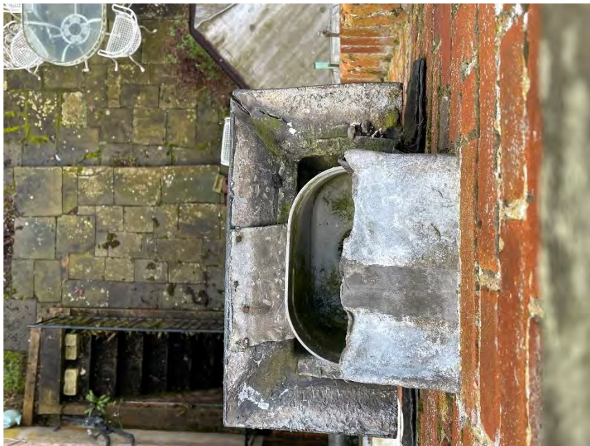
Existing rainwater outfall from flat roof to hopper (north elevation)
