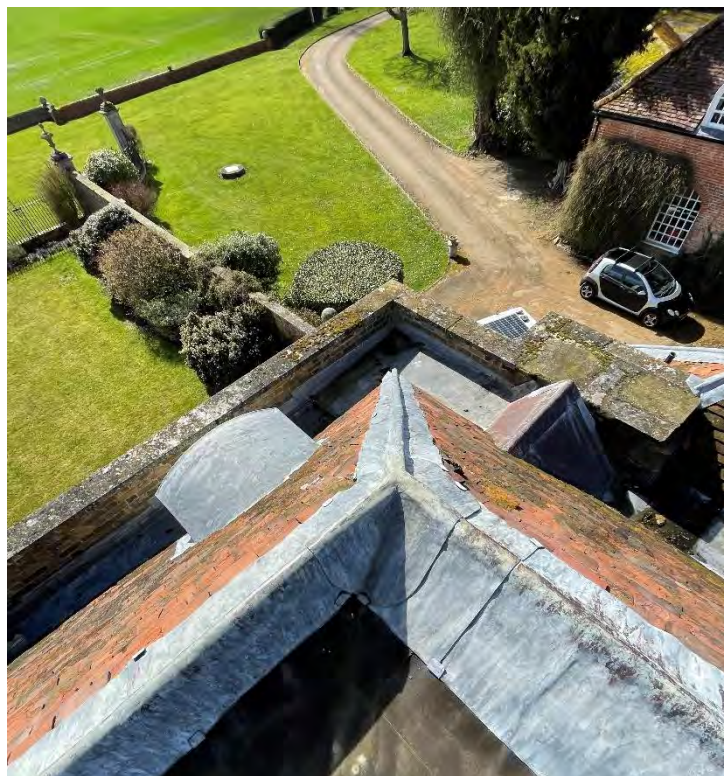
Top of west side lead clad dormer window
