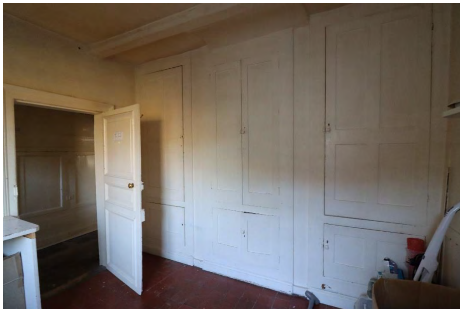
Butler's Pantry. Existing door to be relocated to form lobby in corridor. MC20th fitted cupboards to be relocated to new Butler's Pantry
