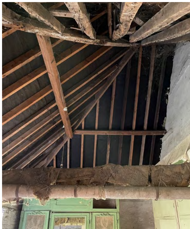
Location above existing store for new floor
