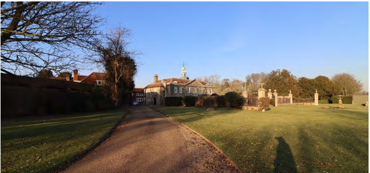
Single drive continues to courtyard adjacent to west elevation of villa
