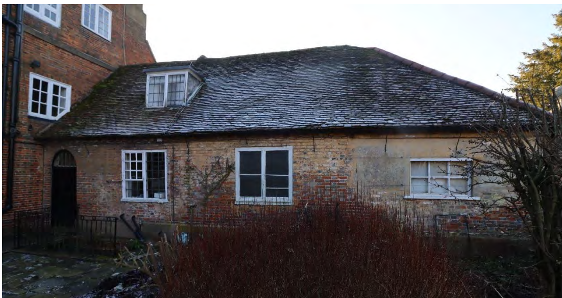
West elevation of service wing
