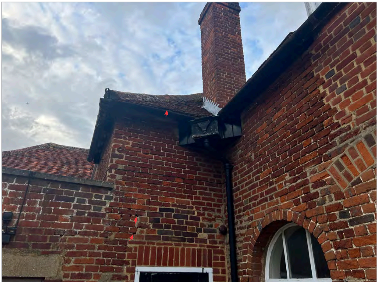
Coach House common pipistrelle and brown long-eared bat roost exit points (red arrows)
