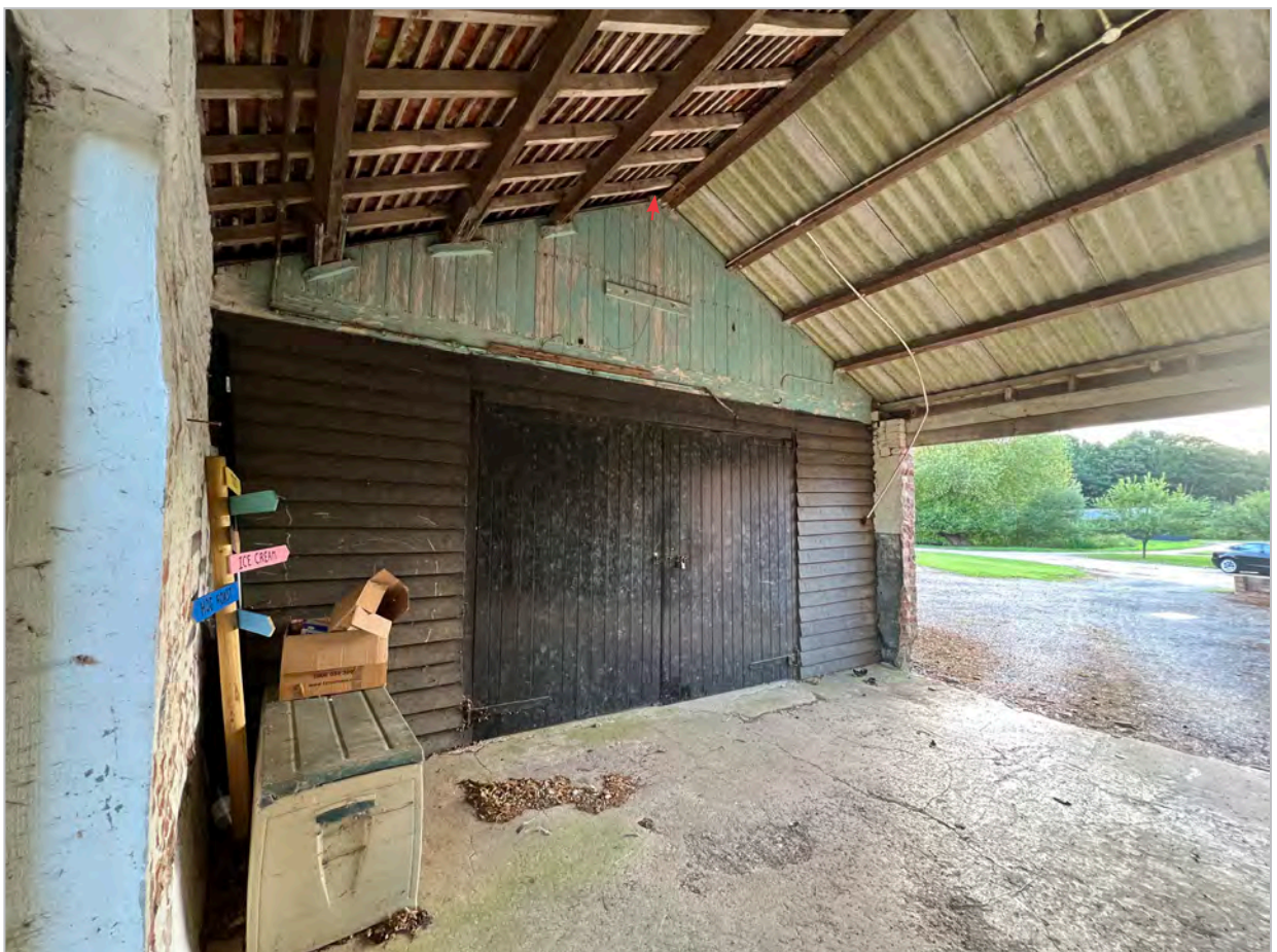
Gap above garage doors at east end of building used by brown long-eared bats to move between garage sections
