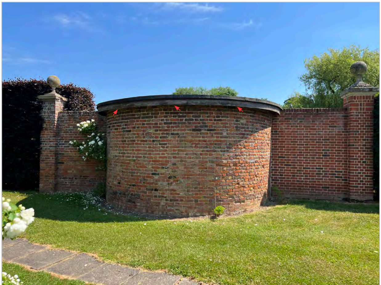
Pool Building common pipistrelle roost exit points
