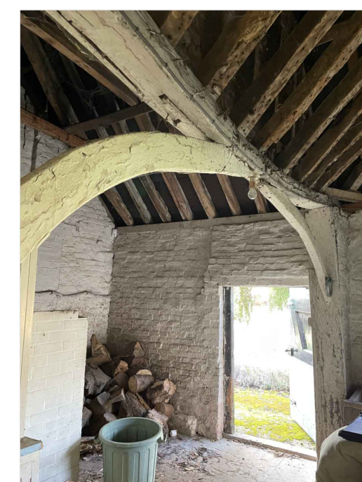
Photo of existing timber brace in store
