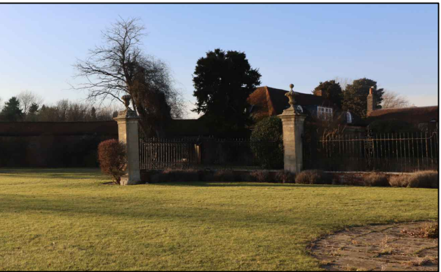
Photo D: Curved wall and railings and 'leaning' pillar as existing
