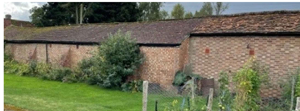
Photograph of South-East Elevation
