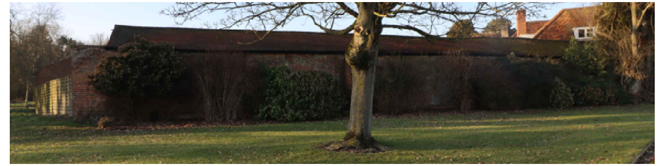
Photograph of South-East Elevation
