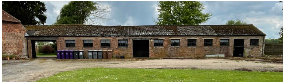
Photograph of North-West Elevation
