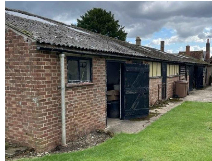
Photograph of North-West Elevation
