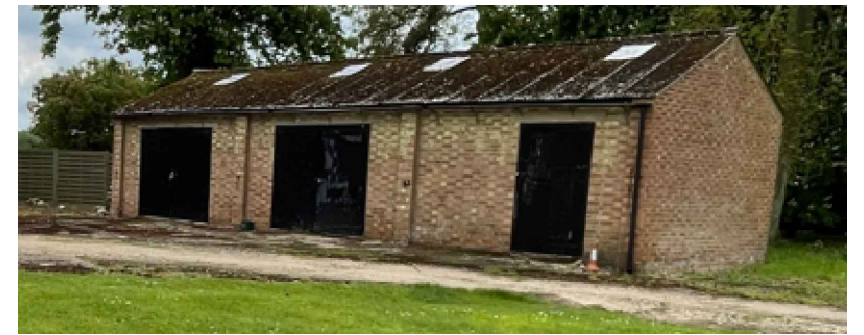
Photograph of North-East Elevation
