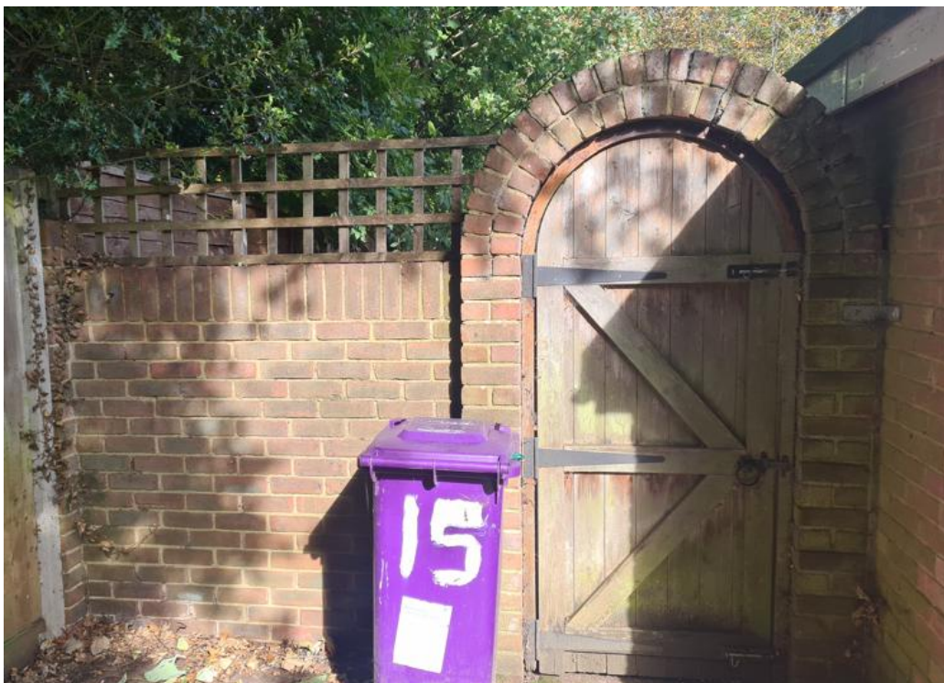
Figure 7 – Modern gate/wall to be removed within the proposal
