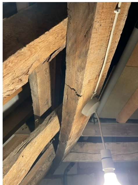
Historic purlin beneath original rafters and lots of modern packing down from the new rafters
