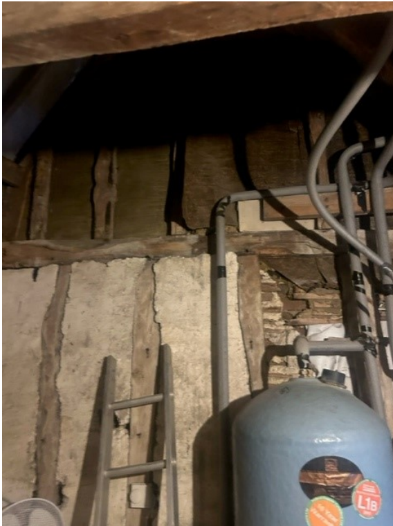
Hot water cylinder will be removed and replaced as part of a conversion to a pressurised system
