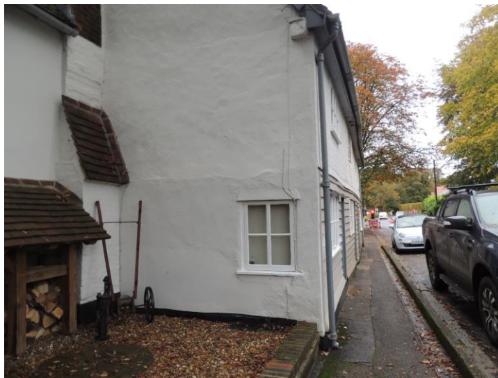
Photo 13: Showing proximity of front of property with road
