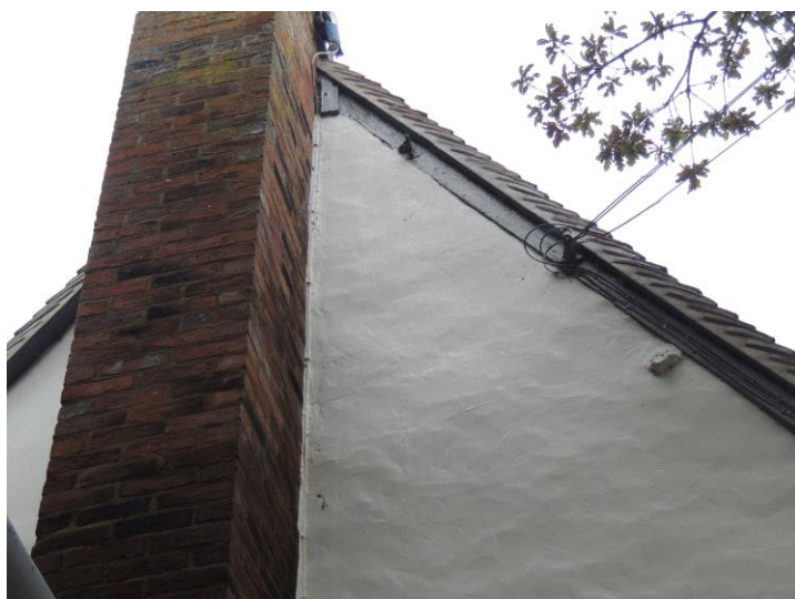
Photo 9: Note tight seal to gable
