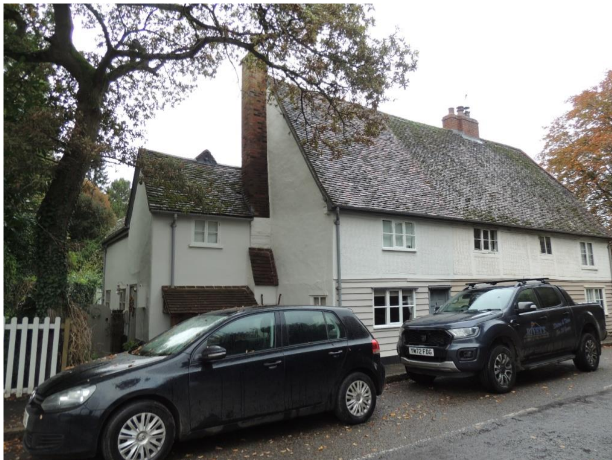
Photo 1: Front (eastern) elevation
