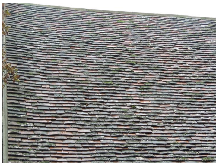
Photo 10: Note tight seal to roof tiles
