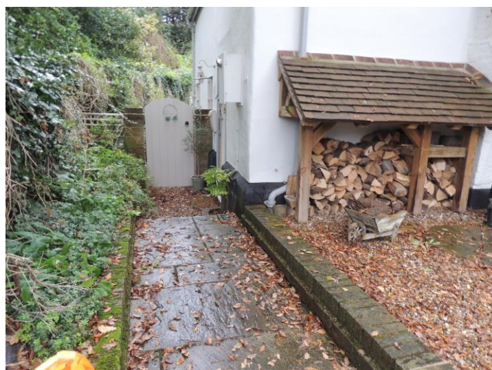
Photo 14: Southern side of the house
