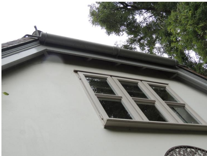
Photo 11: Note tight seal to eaves
