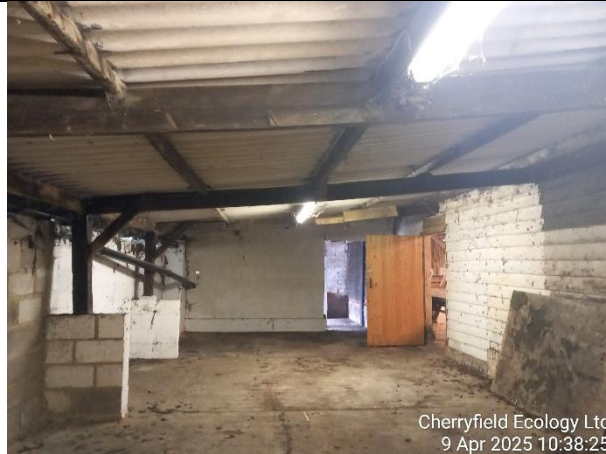
Figure 7: Interior of B1.
