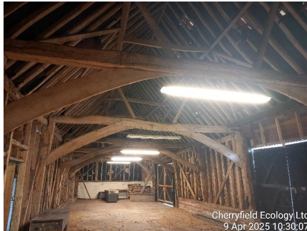
Figure 5: Interior of B1.
