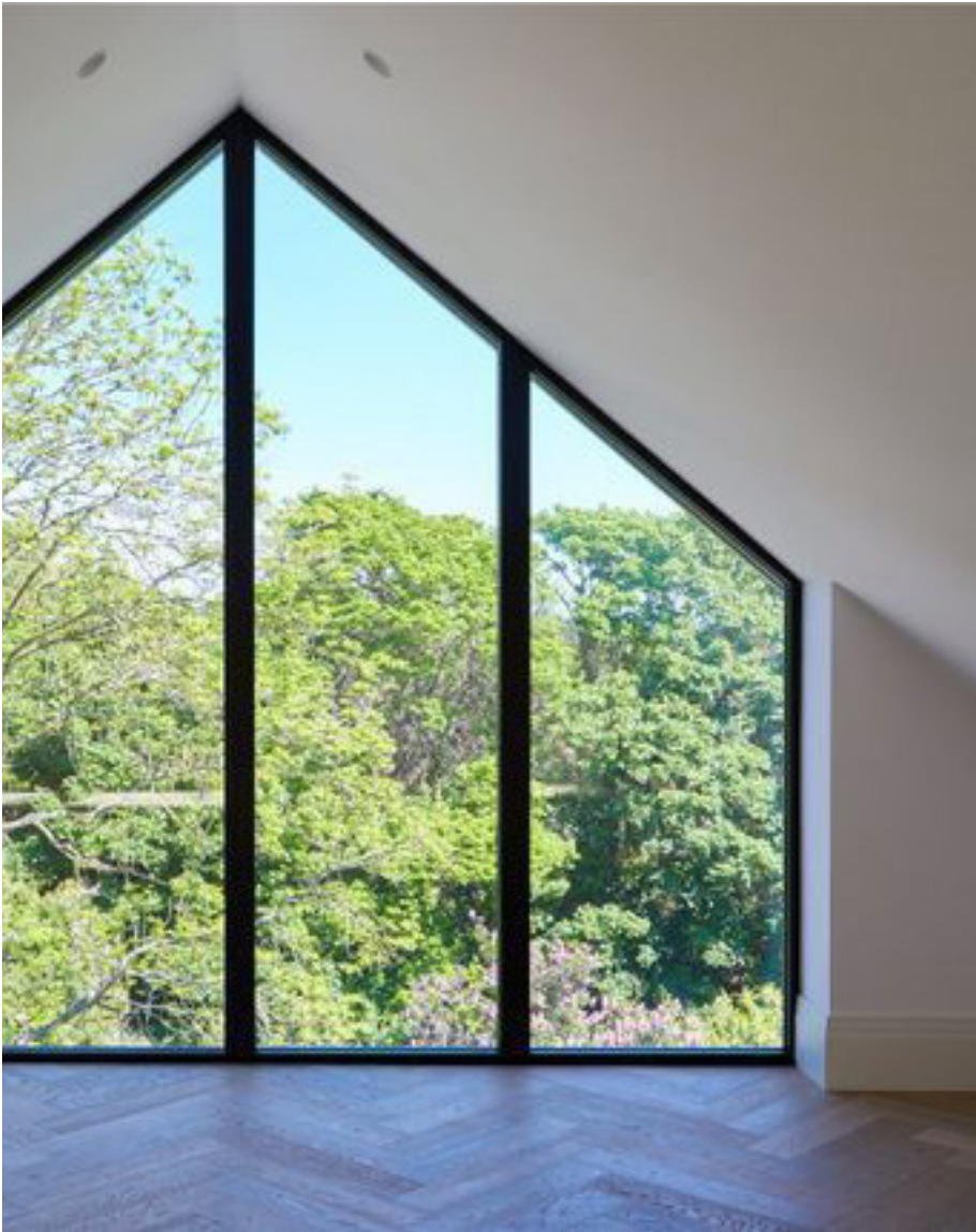
Window at the gable
