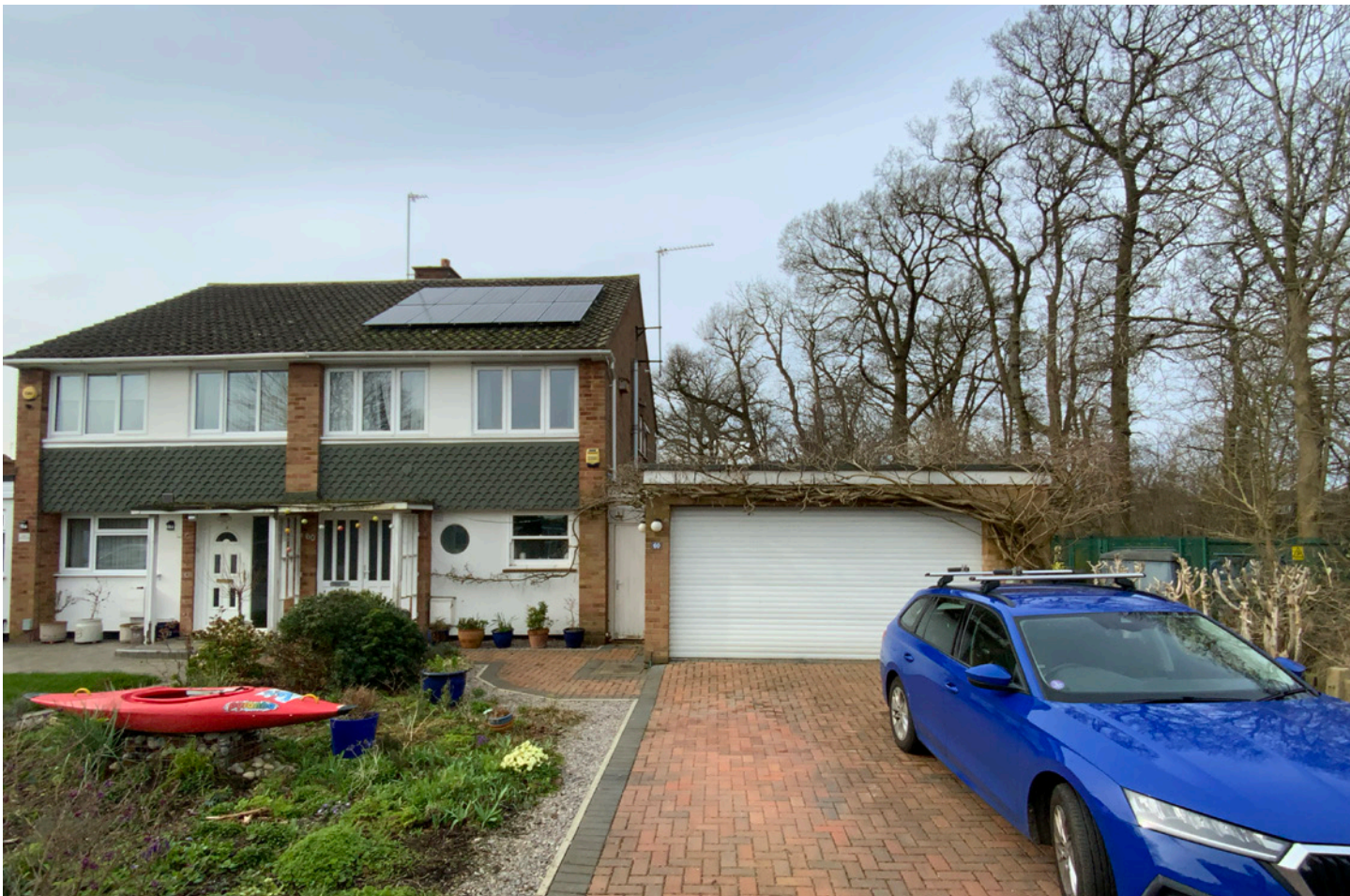
60 Howard Drive - Front elevation, front garden and access - view from Howard Drive
