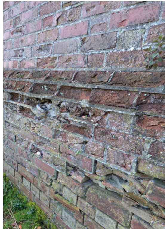
Structural failure / inward lean to arch
