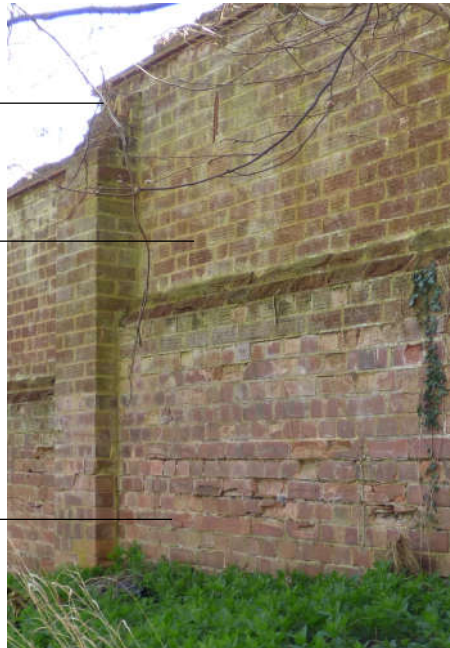
Original section A2 adjoins rebuilt section A1
