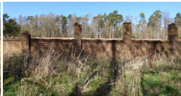
middle section of wall with slender piers
