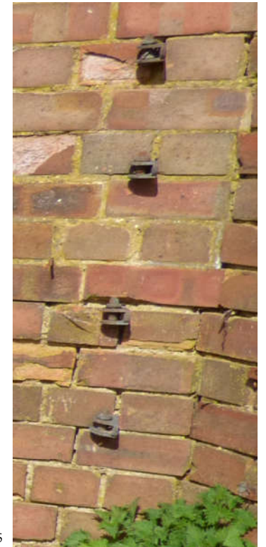
Surviving tension spools for vine wires
