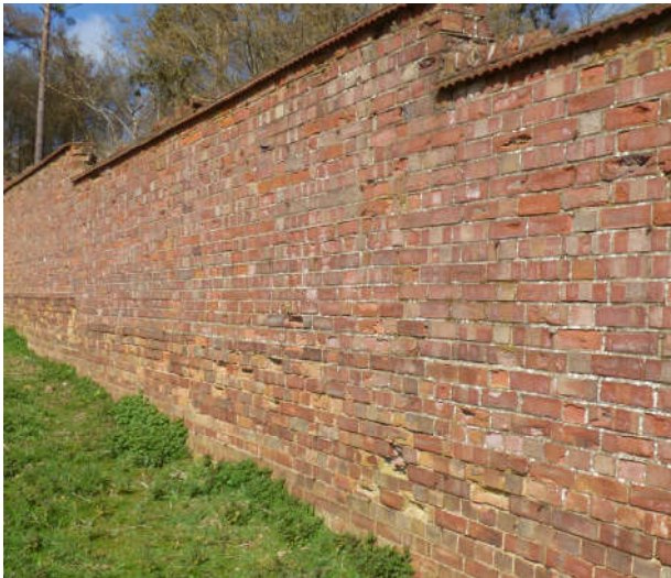
Sequence / construction break in brick type + jointing visible as increased erosion of lower 10-12 courses
