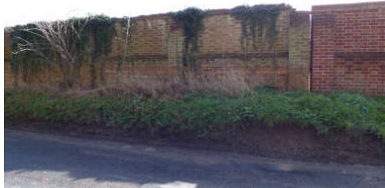
Original section A2 adjoins rebuilt section A1
