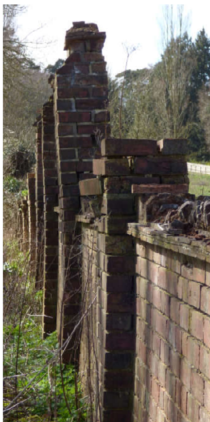
Right – Slender piers, open jointed and out of vertical.
