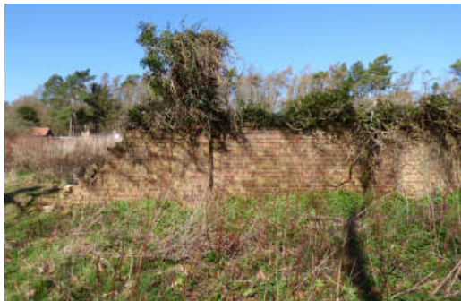
Southerly end of wall section (C) – low level without piers
