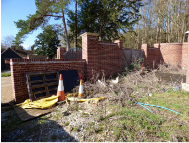
Section A1 - Wall rebuilt at entrance + electric sub-station
