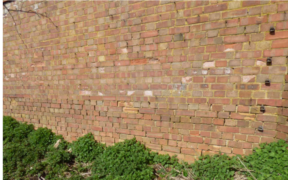
A2 also exhibits the visible change in construction at low level seen clearly along elevation B1-B2
