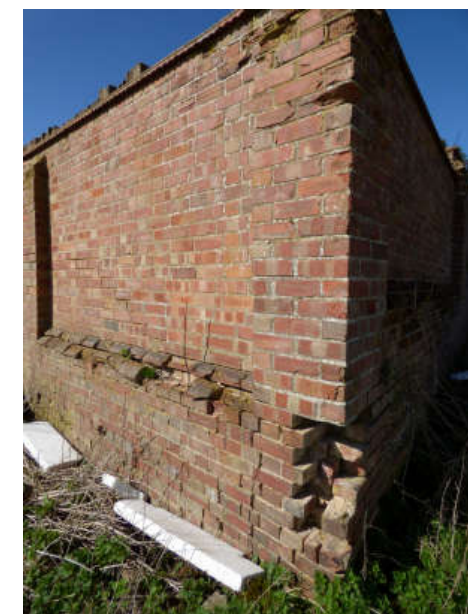
Above – Damaged brickwork at external corner of sections (C) – (B). Decayed plinth and low level brickwork continues.
