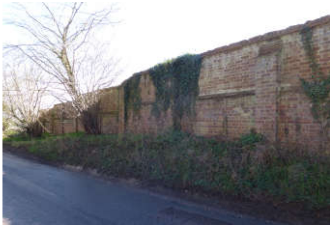
External face of section A2
