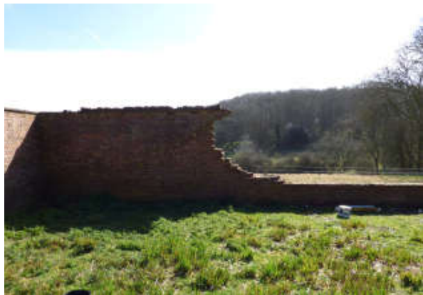
South East wall Section C I----- fallen section -----I
