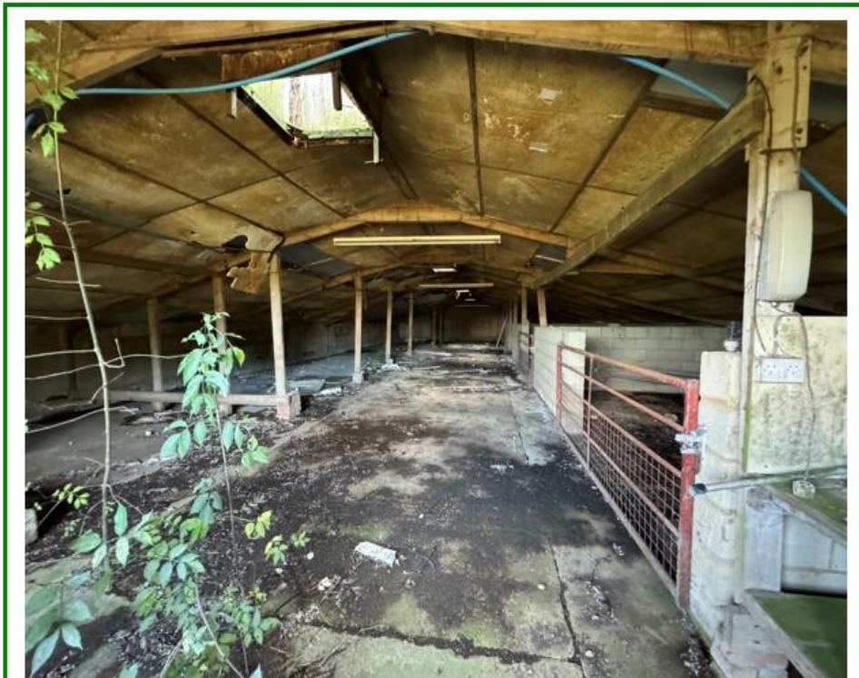
Photo No.12: Facing west inside the far eastern extent of the poultry shed and eastern section showing animal pens
