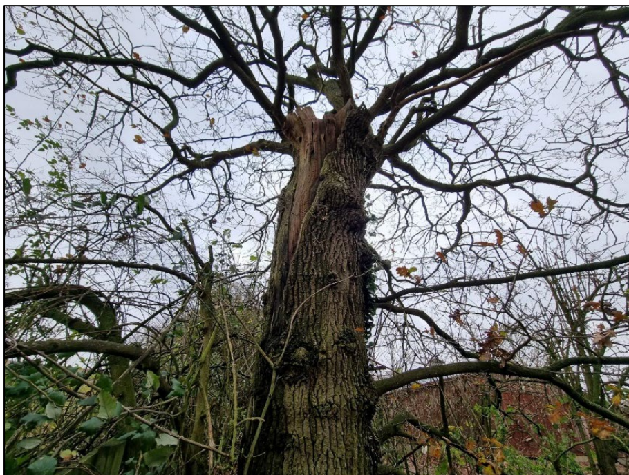
Oak tree on the northern boundary with bat roosting potential
