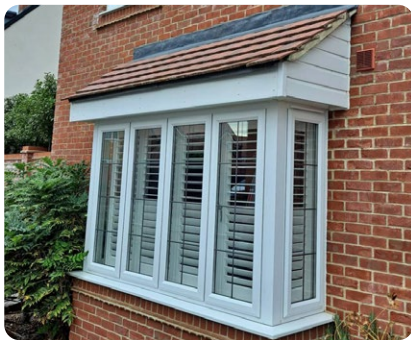
8 Feature Bay Windows
