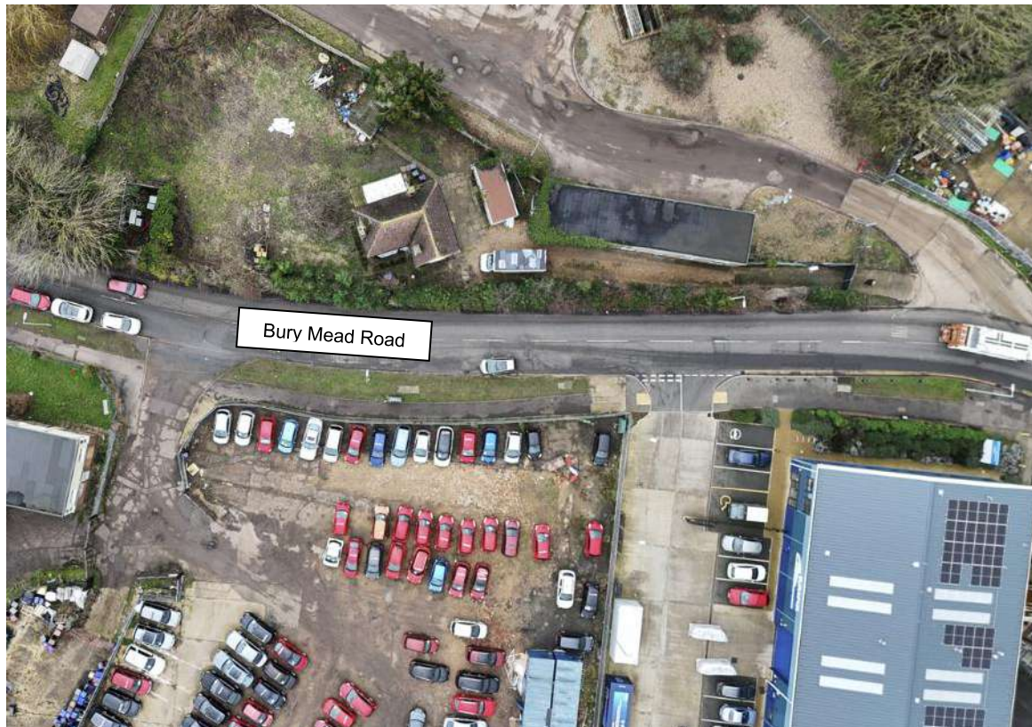
Figure 15 – Bury Mead Road – NW/SE
