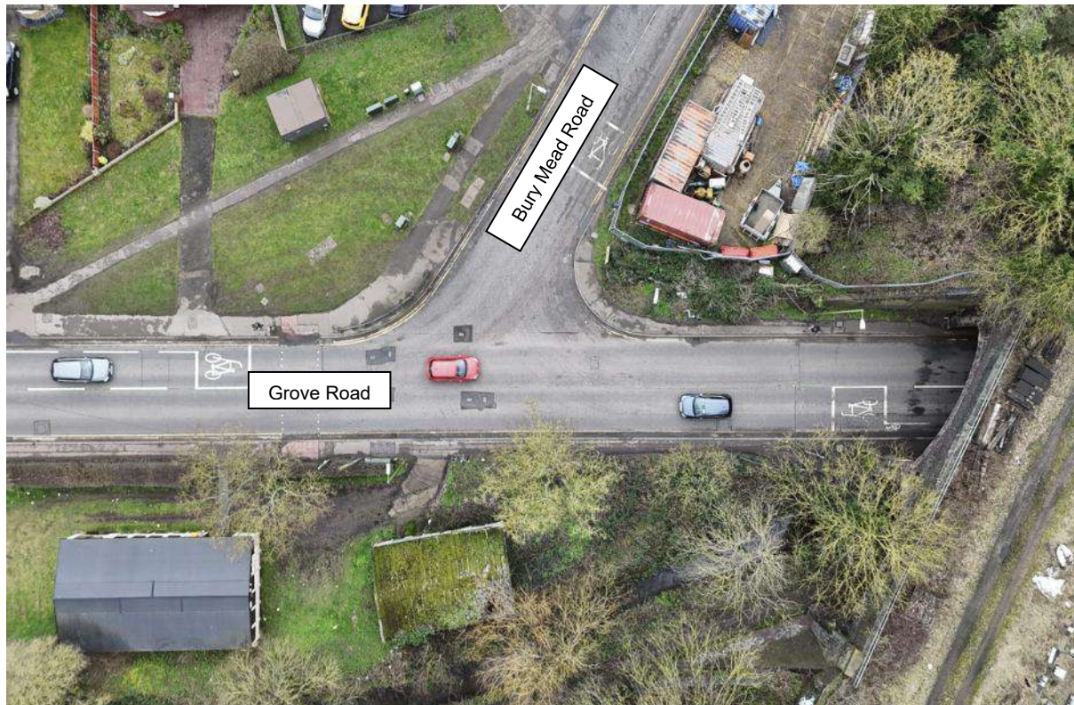
Figure 17 – Grove Road / Bury Mead Road signal controlled junction - SW/NE
