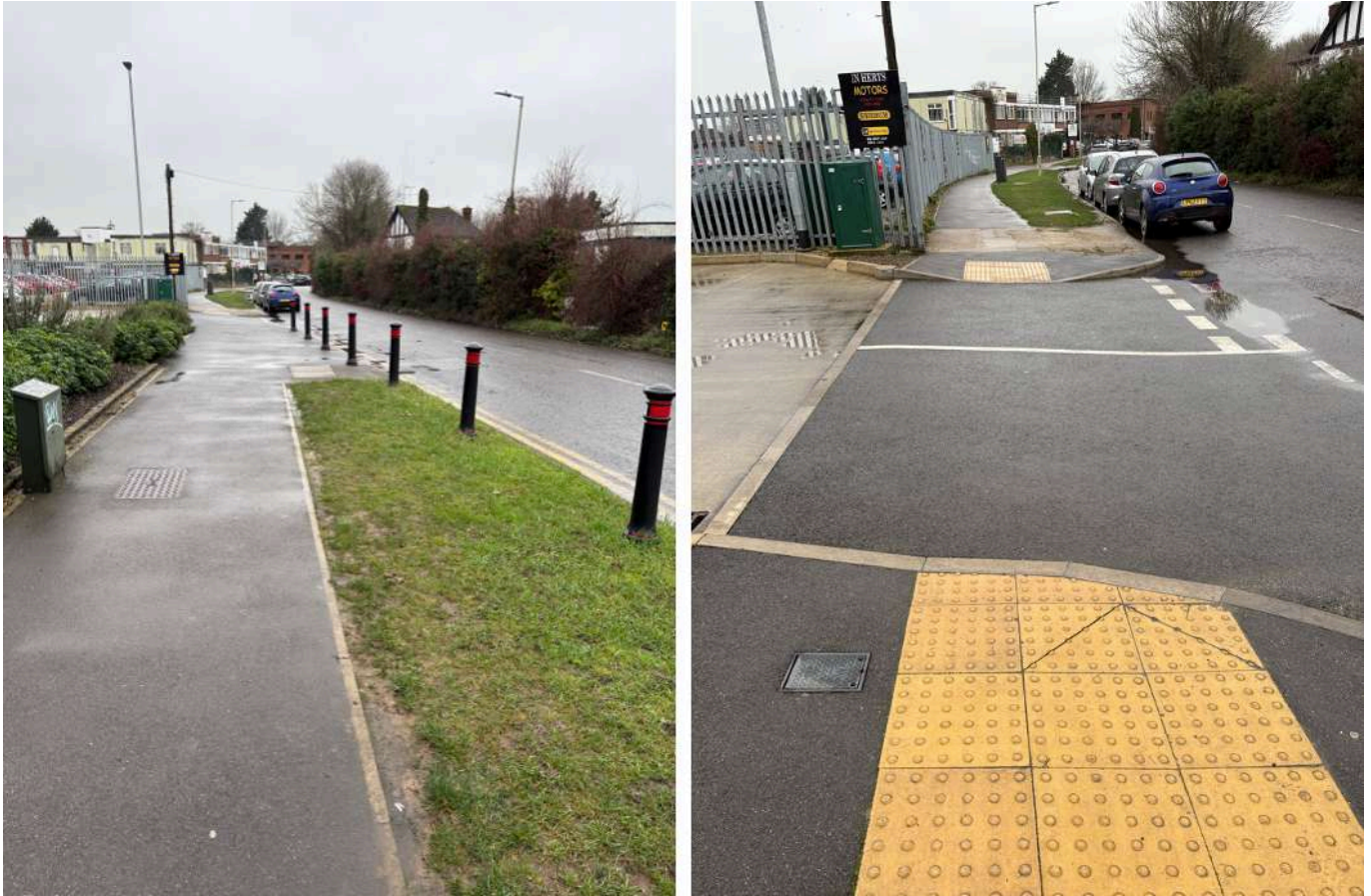
Figure 5.1 Existing Conditions at Southern End of Bury Mead Road
