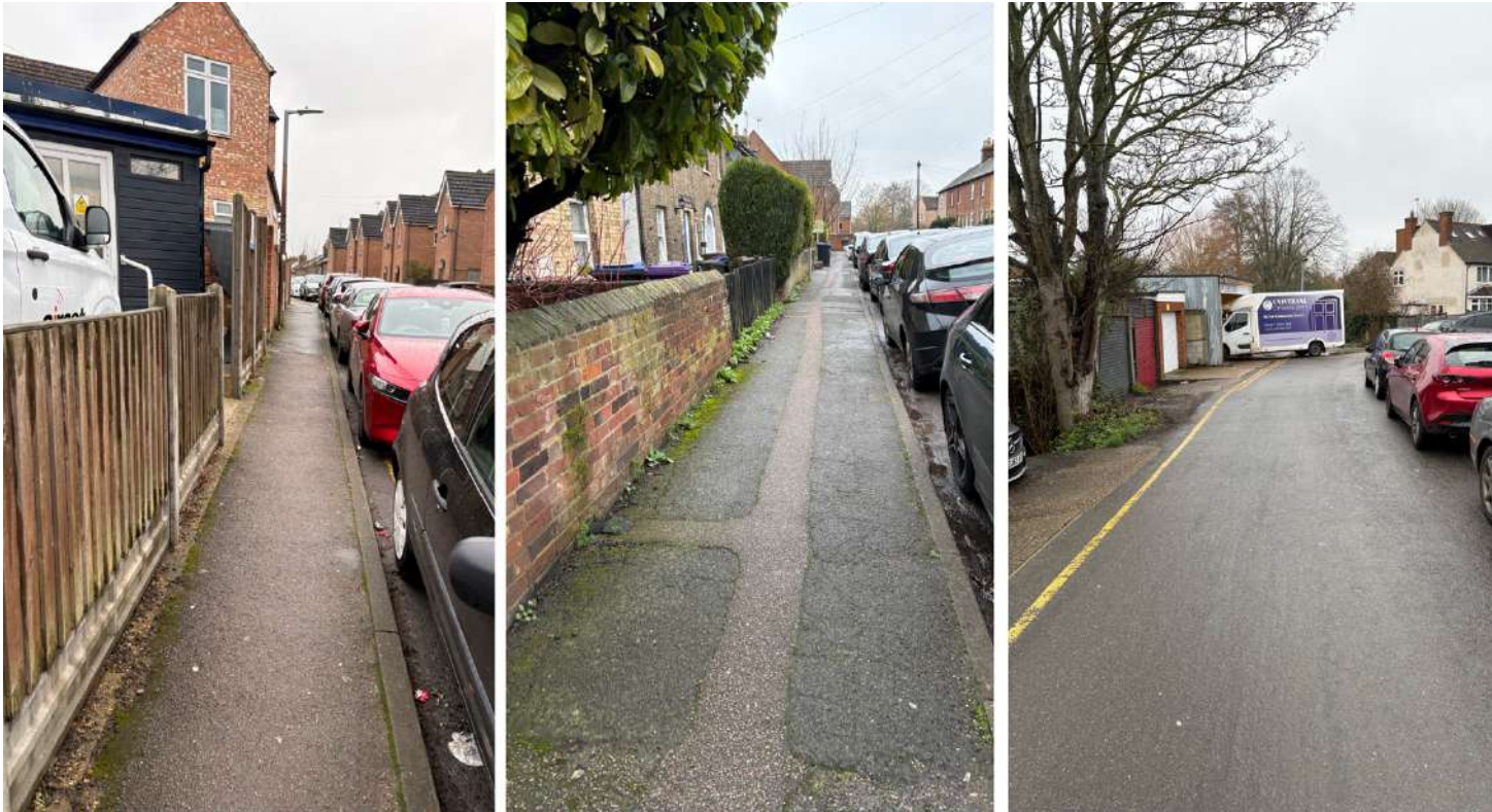
Figure 5.4 Florence Street Footway
