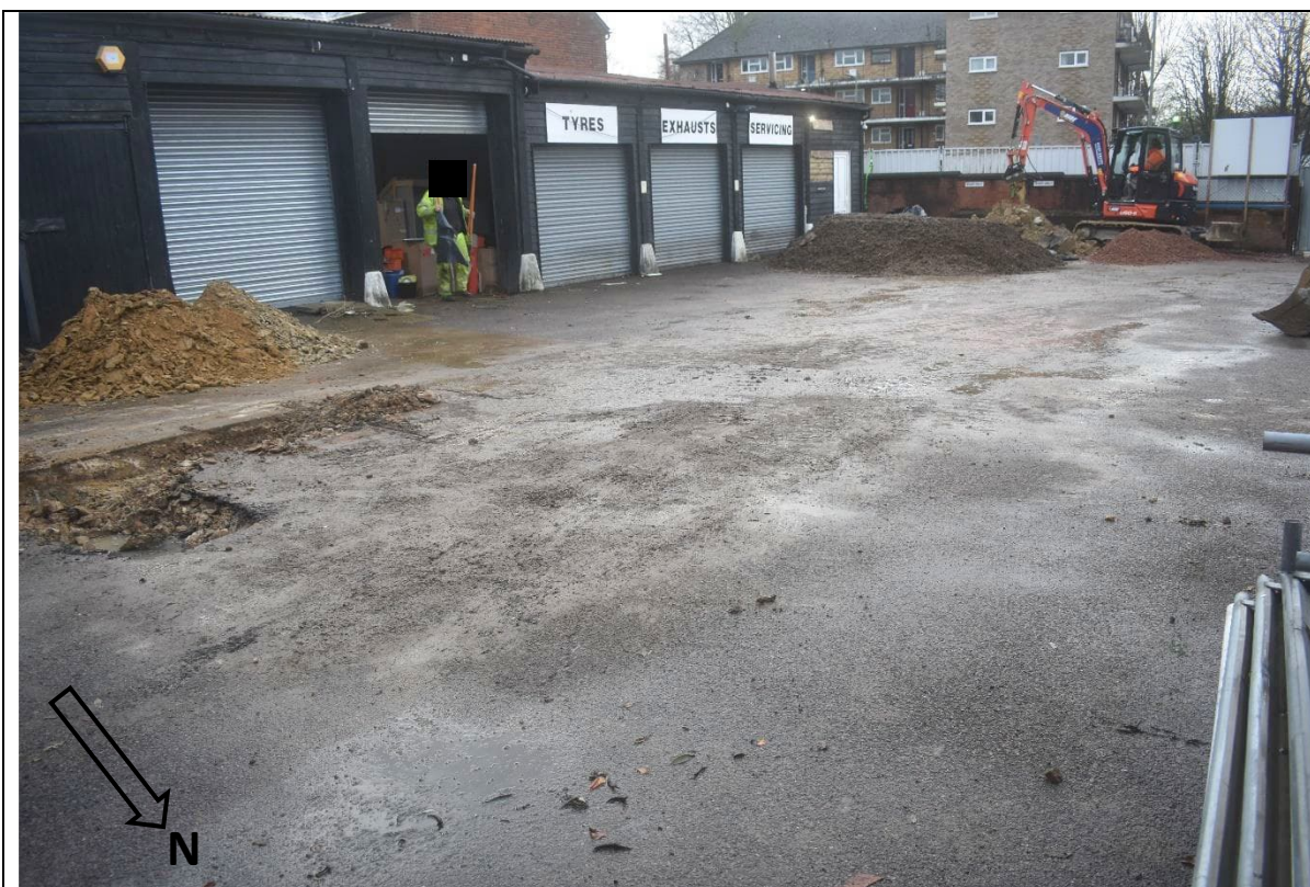
Plate 1: Pre-excavation view across the site, looking south-west, showing tarmac hardstanding (100 and 200)
