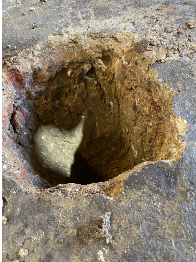
Photo 3—HP102 conducted within the existing garage building to the southern end of the site which is proposed to become part of the proposed residential gardens
