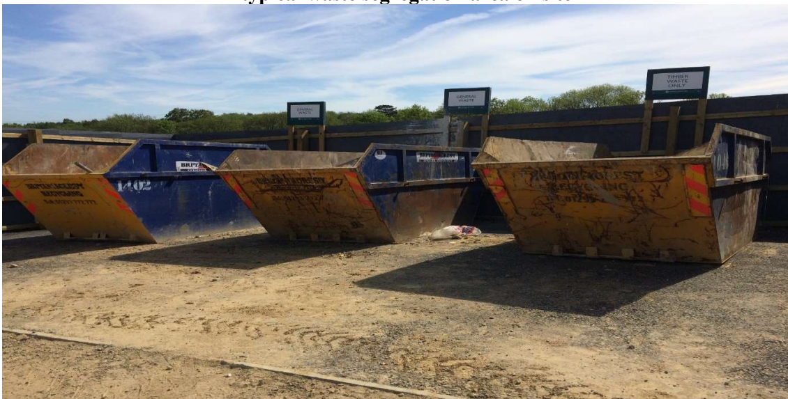
A typical waste segregation area on site
