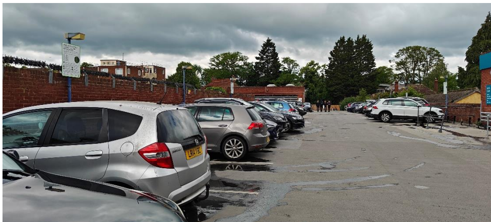
Photograph 1: Rooftop car park
