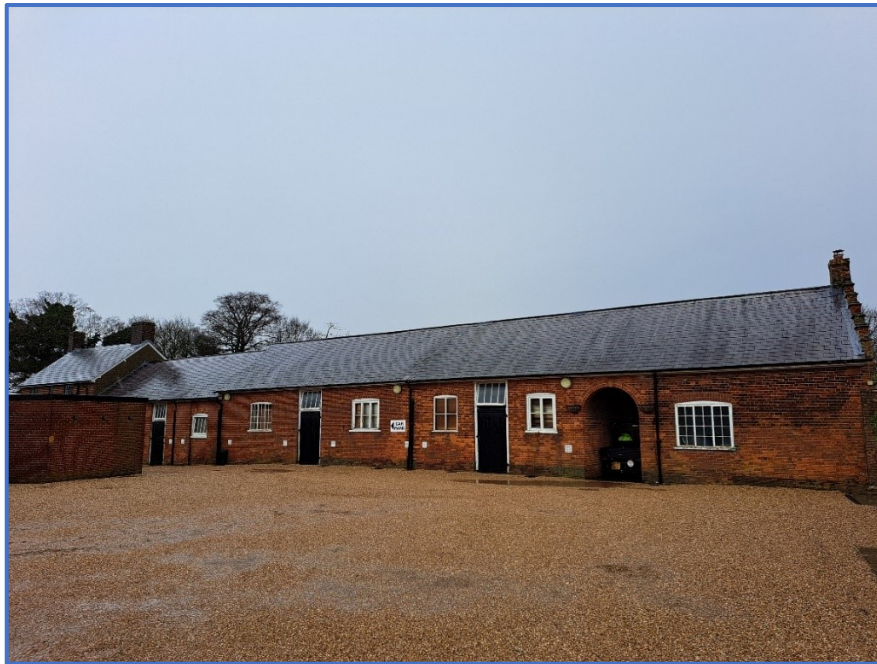
Figure 3 – Front elevation of stables building
