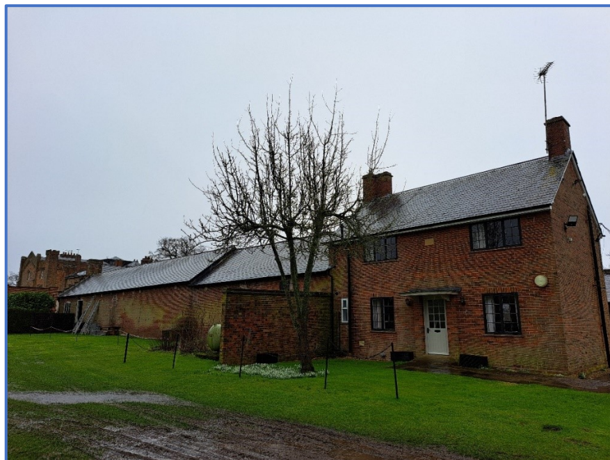
Figure 4 – Rear elevation of stables building
