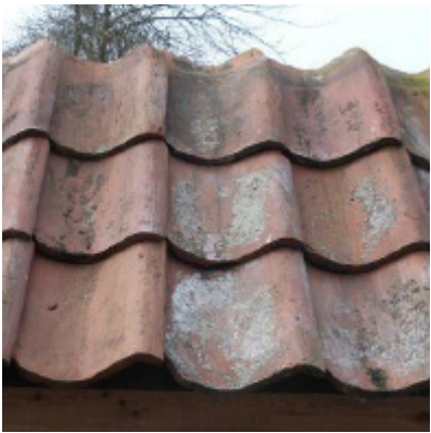
8. Existing Roof Tiles Material. Red Clay Pantiles Location. Existing Main Barn Colour. to match existing in all respects
