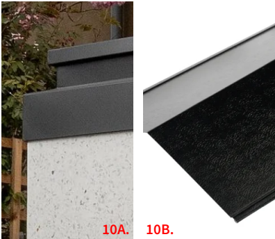
10 A. Capping Material. Powder Coated Aluminium Location. Lean-to & Family Bath. Link Colour. Graphite Black RAL 9011
