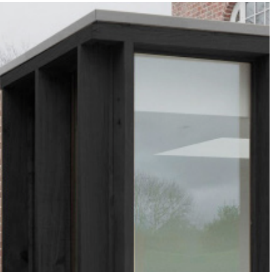
3. Window Posts Material. Black Natural Oil Wood Stain Larch Posts. Location. Bedroom Wing Extension Colour. Black
