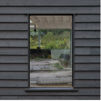
6. Windows & Doors (B) Material. Aluminium Glazing. Double Glazed, Laminated Location. Existing Main Barn & incl. NE Elevation of Lean-to Supplier. Maxlight Colour. Graphite Black RAL 9011
