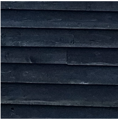
7. Existing Feather Edge Horizontal Timber Cladding Material. Black Natural Oil Wood Stain Timber Cladding Location. Existing Main Barn Colour. to match existing in all respects
