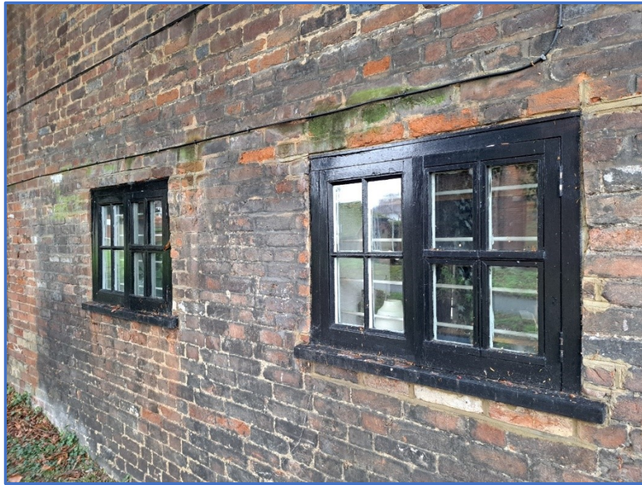
Figure 2 – Ground floor windows to side elevation
