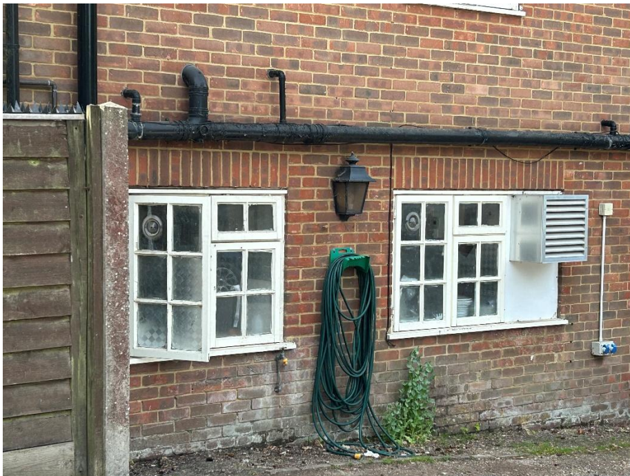
EXISTING INTAKE GRILL TO RH WINDOW
