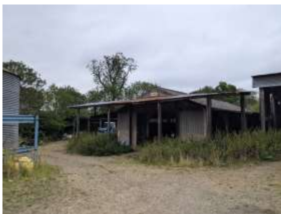
Photo of one of the buildings on Site
