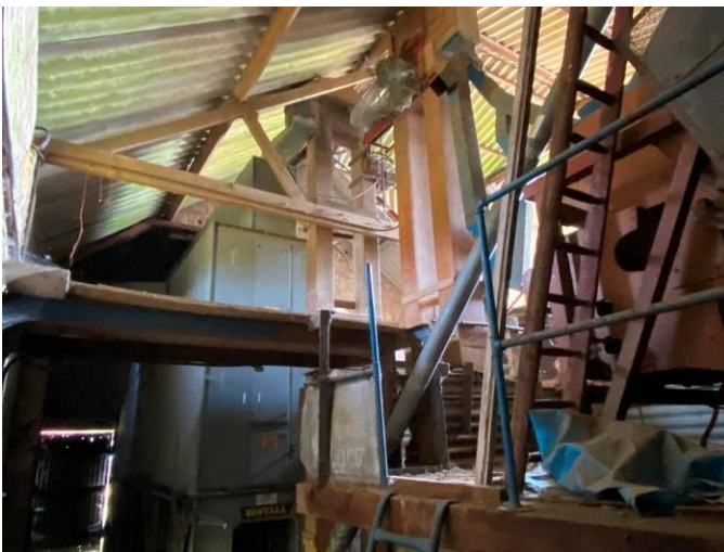
Machinery at north end of Building 1
