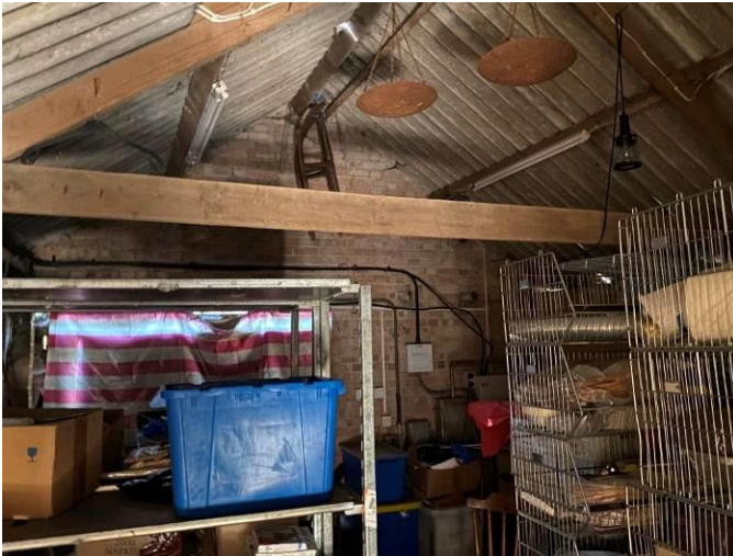
Store at south end of Building 1
