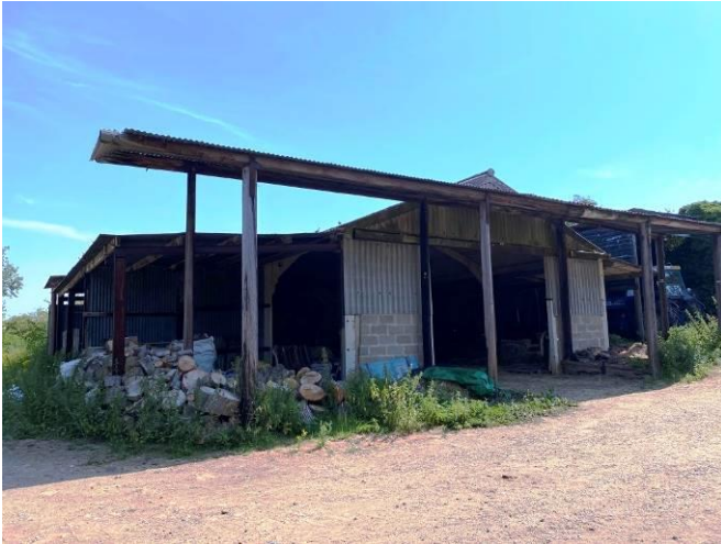
Southwest and northwest elevations of Building 3
