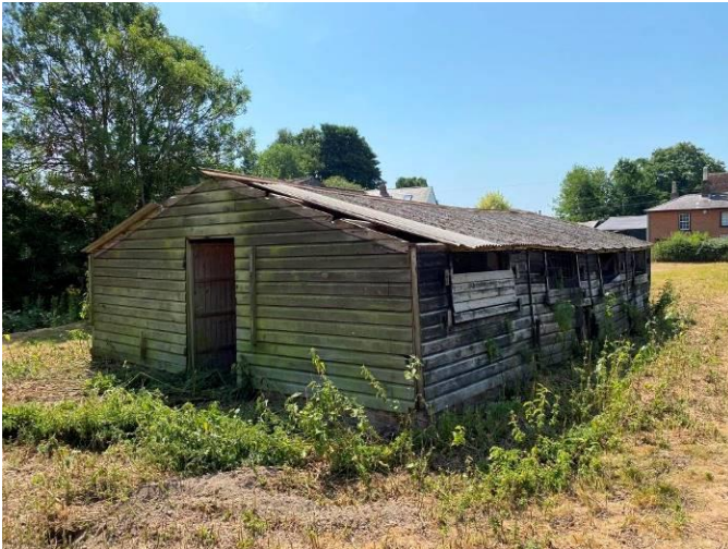
North and west elevations of Building 5
