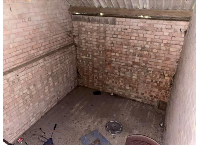
Grain store in centre of Building 1
