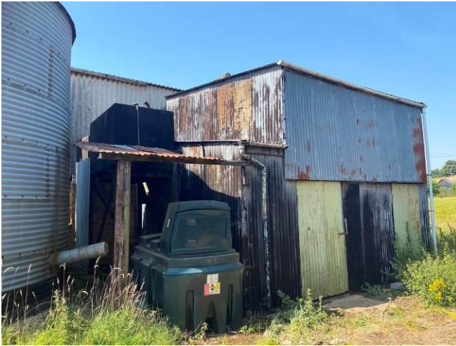
Corrugated iron shed to north of Building 1
