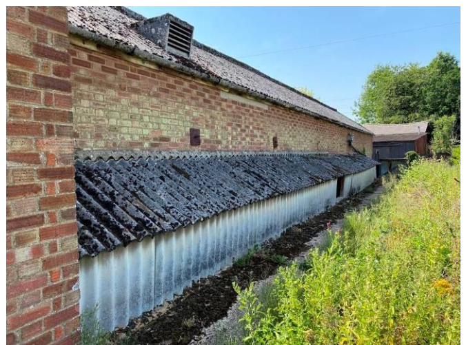
Exterior of walkway on west side of Building 1
