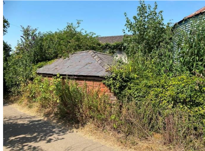
Barn attached to east elevation of Building 2
