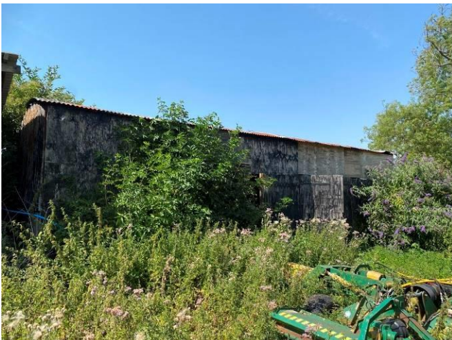
Curved roofed shed to northeast of Building 3
