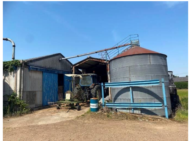
Machinery store and silo to north of Building 1
