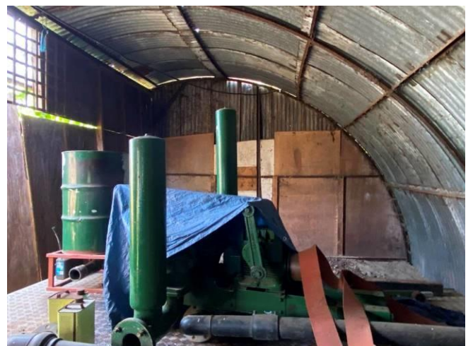
Interior of curved roofed shed
