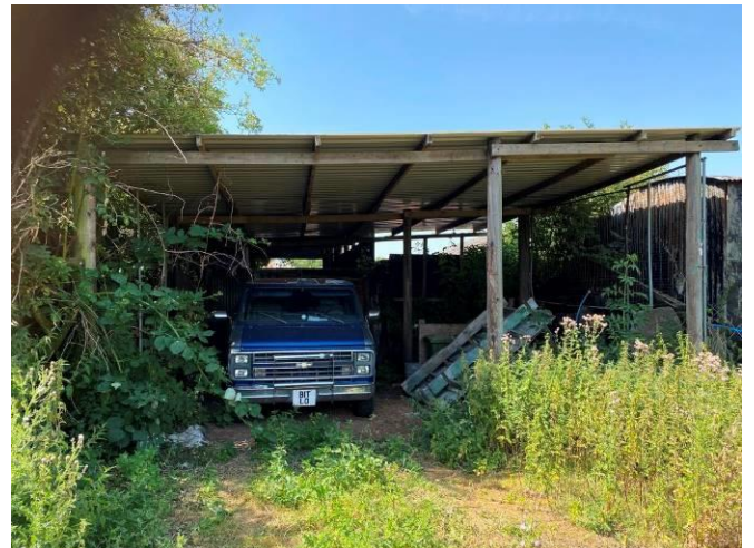
Shed to northeast of Building 3
