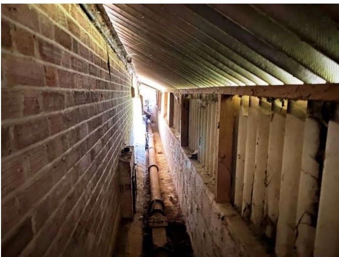
Walkway on west side of grain stores in Building 1
