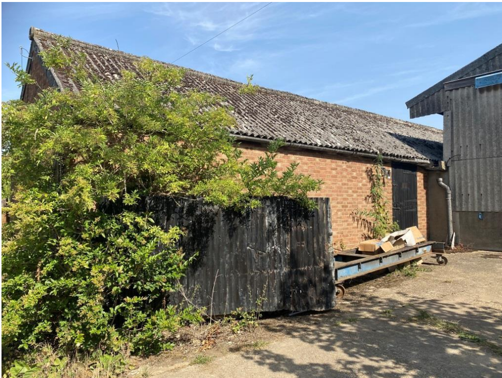
East elevation of Building 1
