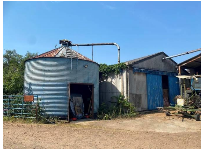
North and east elevations of Building 2 and silo
