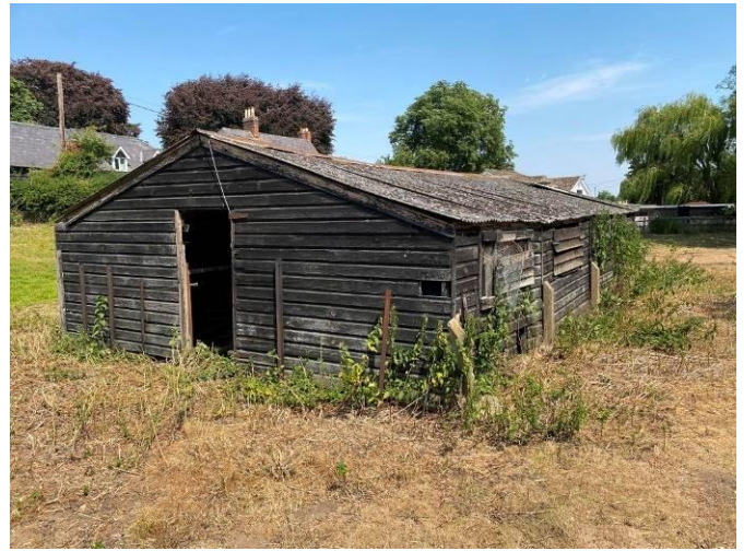
South and east elevations of Building 5
