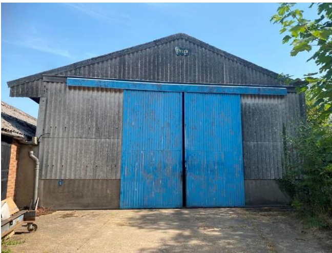
South elevation of Building 2
