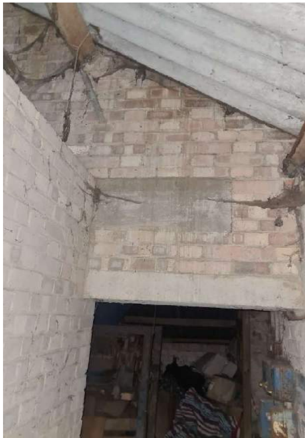
Photograph 21 – Cross Wall Opening between Barns A & B
