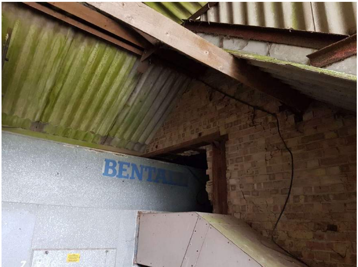
Photograph 27 – Opening Through Cross Wall between Barns B & C
