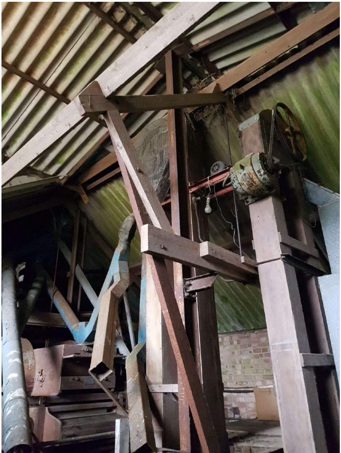
Photograph 28 – Disused Agri-plant and roof support in Barn B
