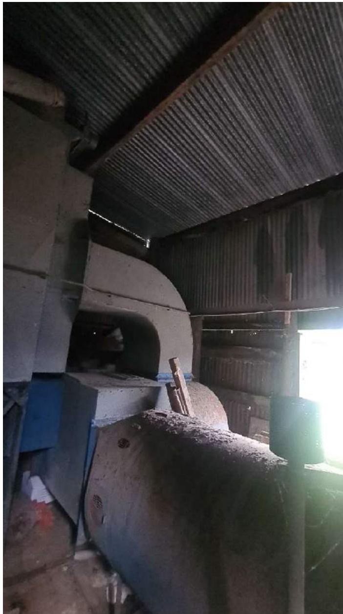
Photograph 36 – Barn C roof and wall structure
