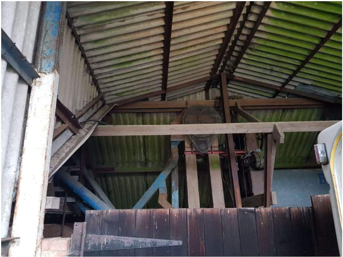
Photograph 26 – Barn Roof Structure with central post
