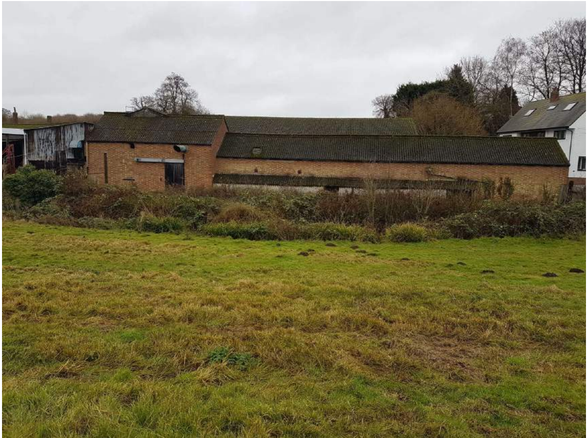
Photograph 1 – Western Elevation of Barns A, B & C
