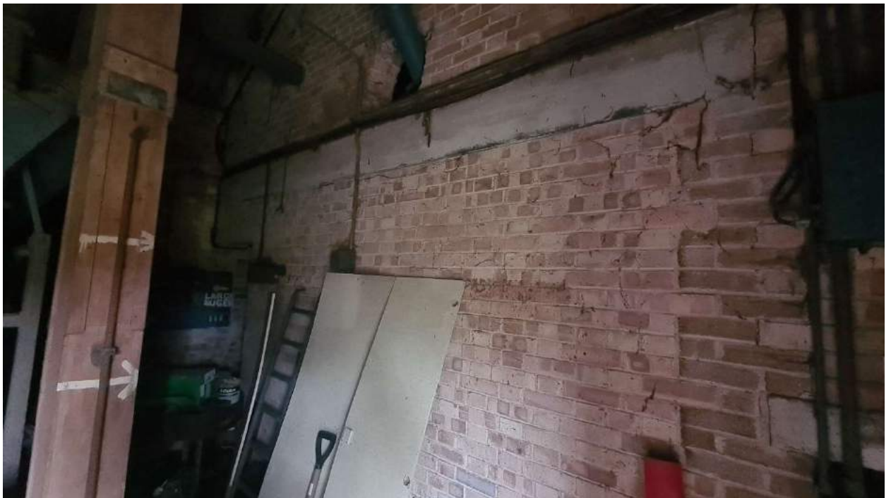
Photograph 25 – Infilled opening between Barns A & B
