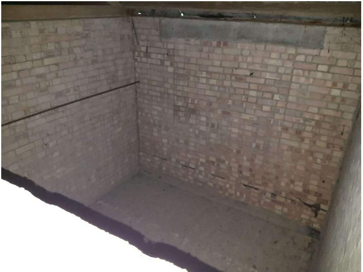
Photograph 13 – Installed Steel Tie in Barn A
