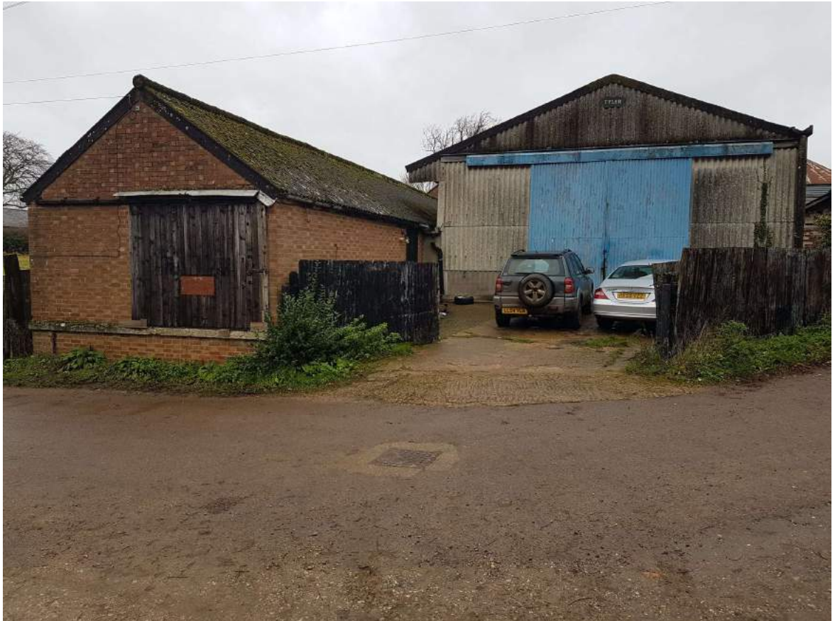
Photograph 3 – Barn A and adjacent portal frame shed on Eastern Elevation
