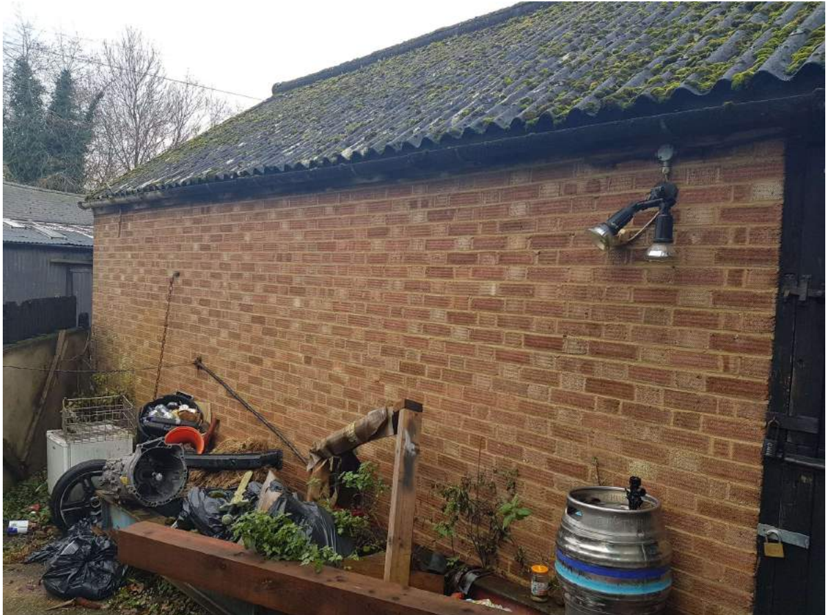
Photograph 8 – Cement Based Roof Sheeting to Barn A
