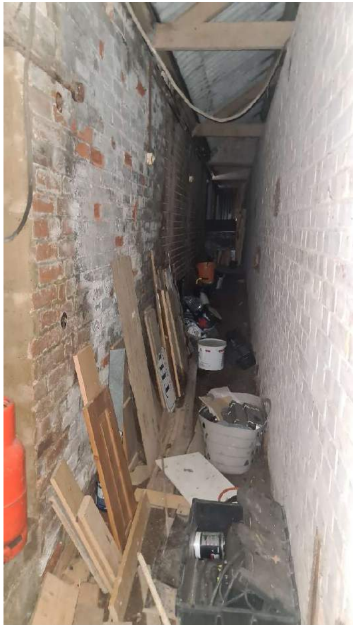
Photograph 19 – Internal corridor within Barn A
