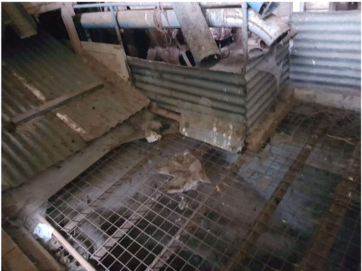
Photograph 30 – Floor Hopper Barn B
