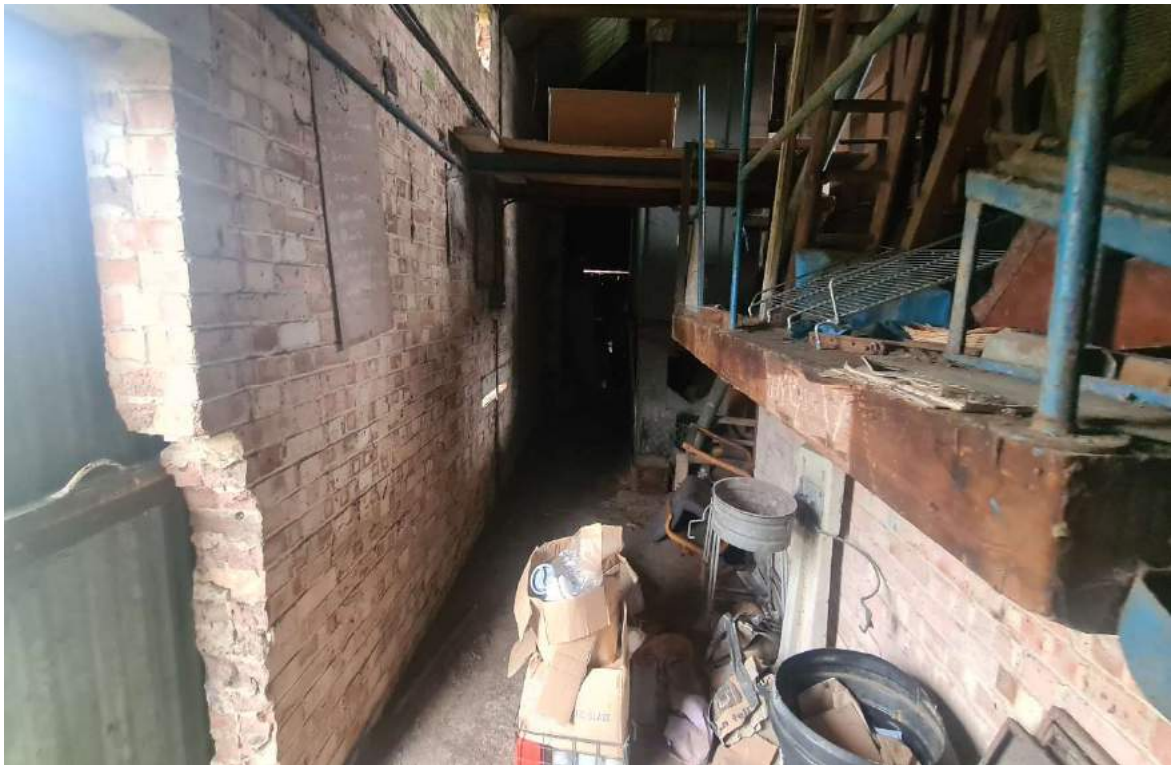
Photograph 24 – Removed brickwork at entrance door to Barn B
