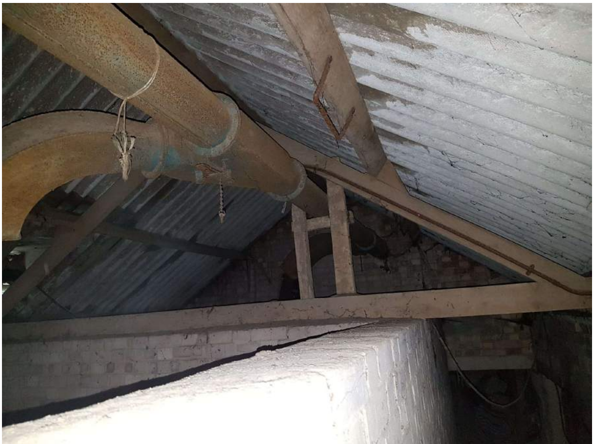
Photograph 14 – Timber Truss, Purlins and Roof Sheeting in Barn A
