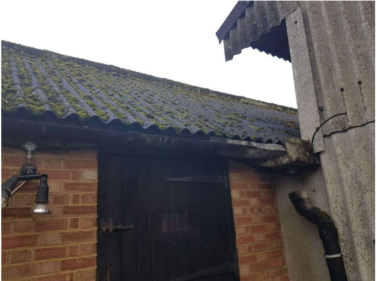
Photograph 9 – Junction between Barn A and concrete portal frame shed
