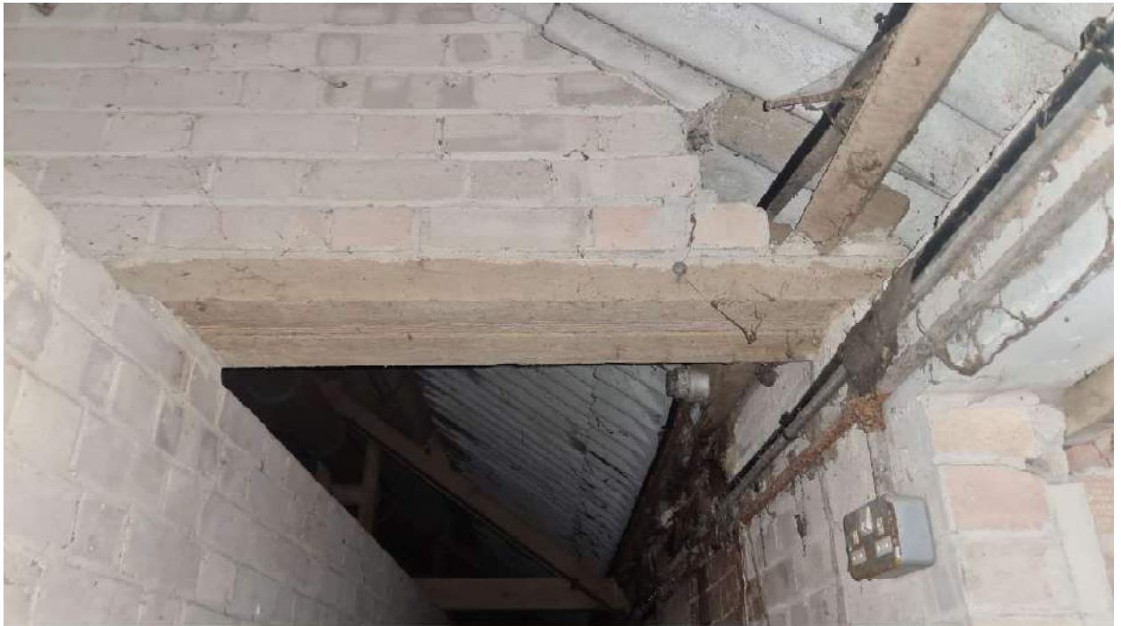
Photograph 17 – Timber lintel in Barn A
