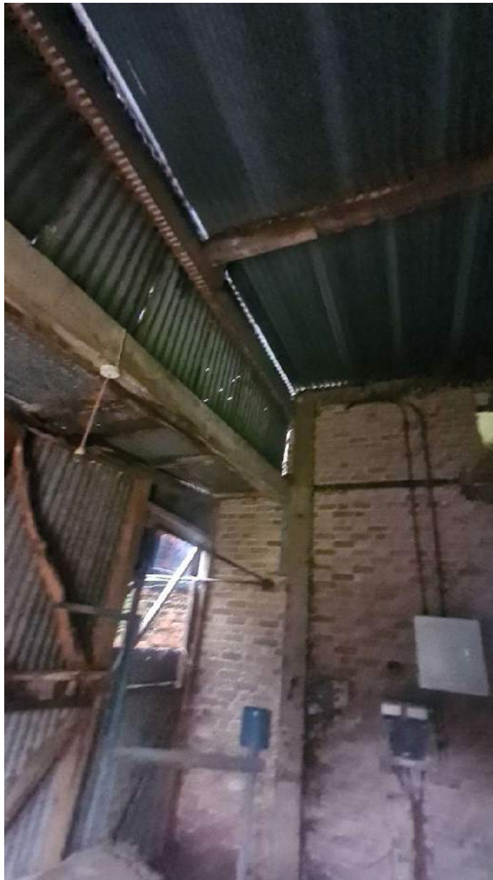
Photograph 35 – Barn C roof structure
