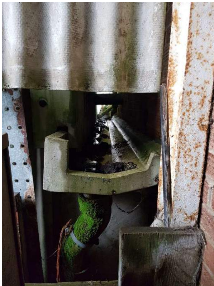
Photograph 10 – Gutter detail between Barn A and concrete portal frame shed
