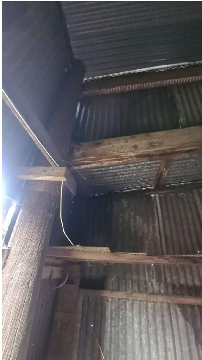
Photograph 38 – Barn C interior roof and wall structure
