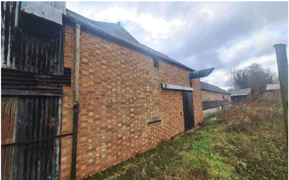
Photograph 23 – Western Elevation of Barn B
