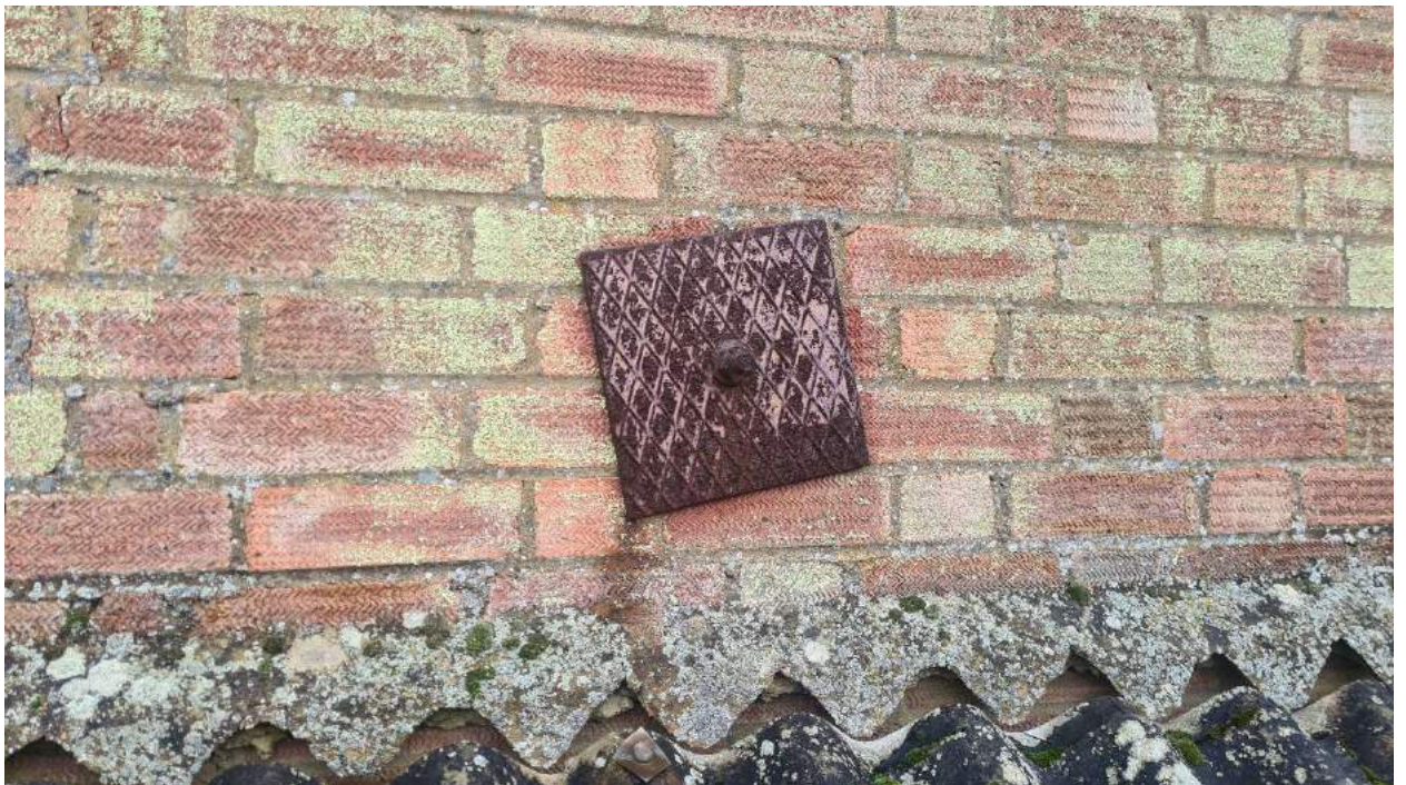
Photograph 6 – Wall Plate Anchor
