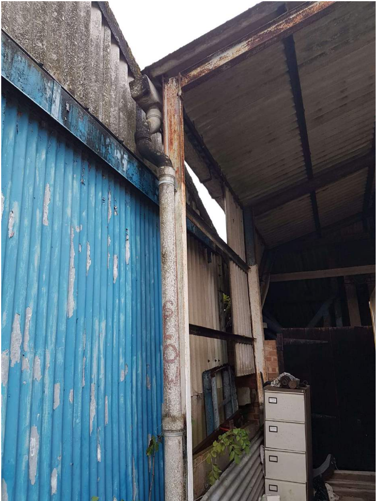
Photograph 32 – Open front lean-to steel frame structure with corrugated tin walls and roof
