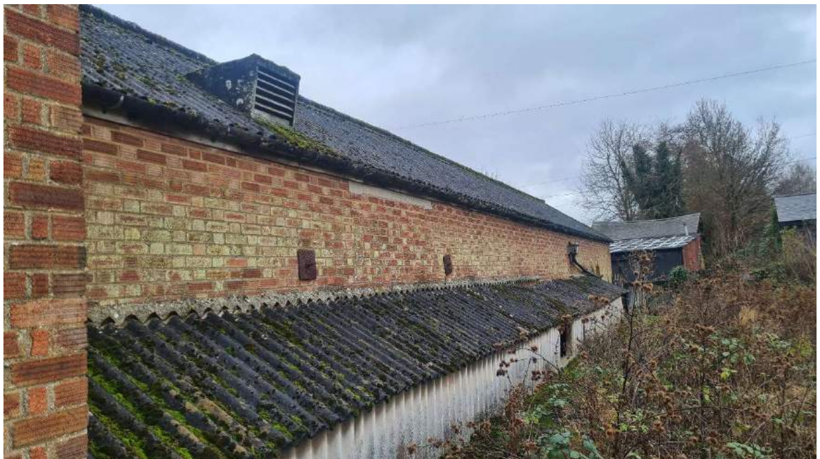
Photograph 4 – Barn A Service Trench lean to on Western Elevation
