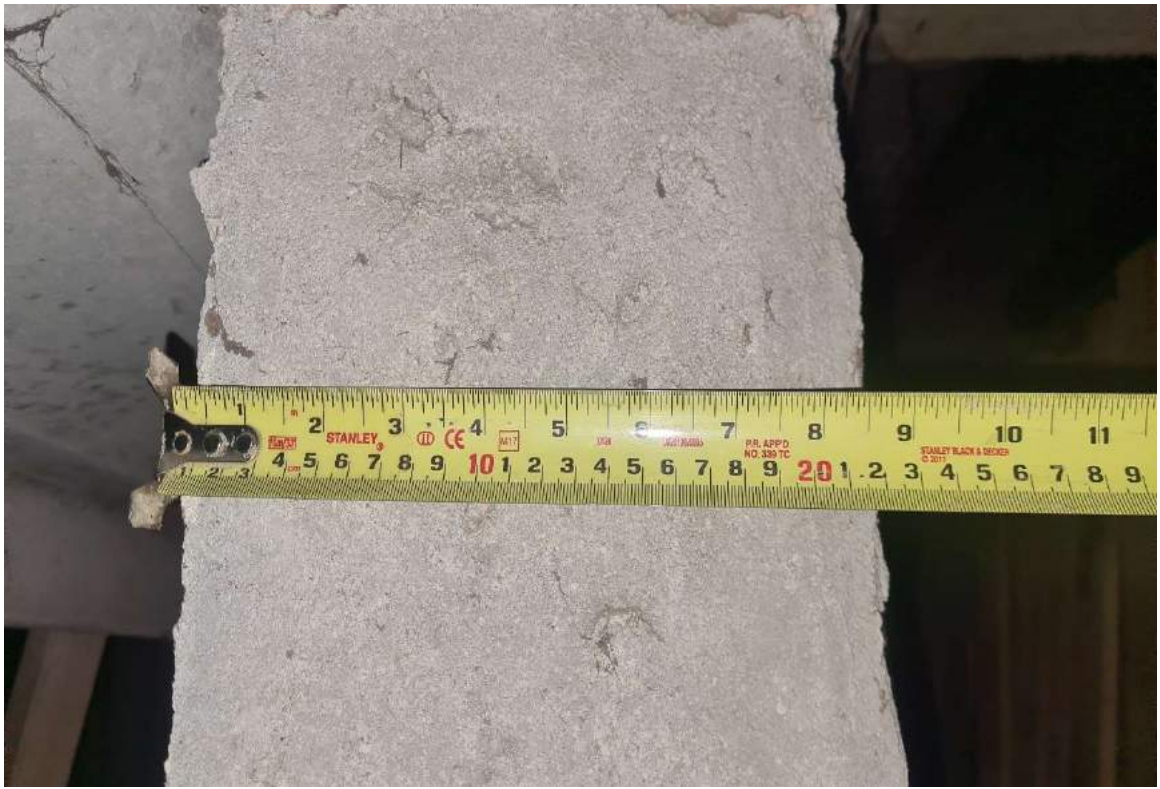
Photograph 22 – Masonry Walls 220mm wide
