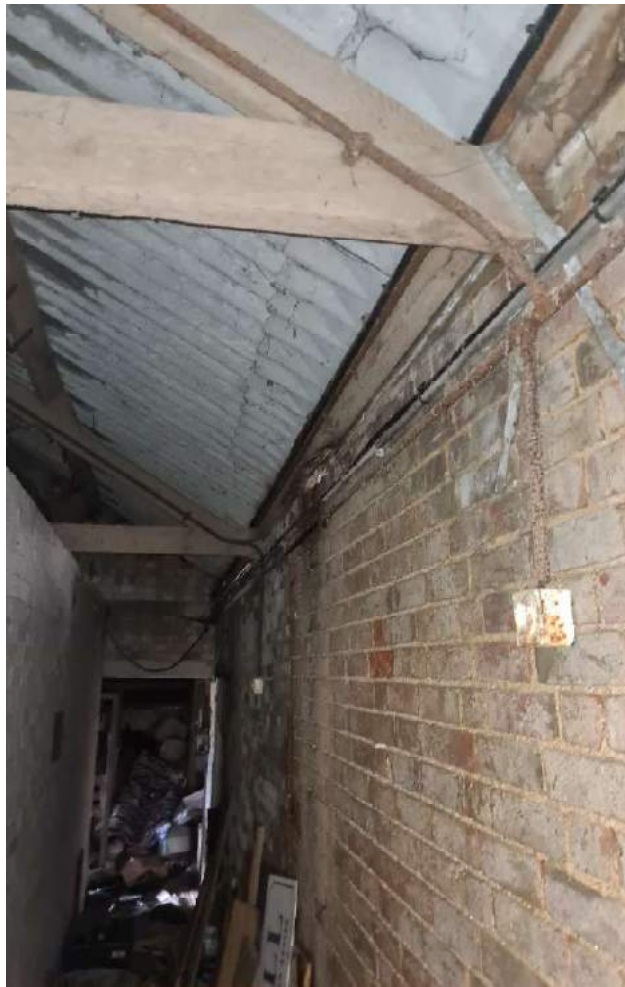
Photograph 20 – Timber Truss support in Barn A
