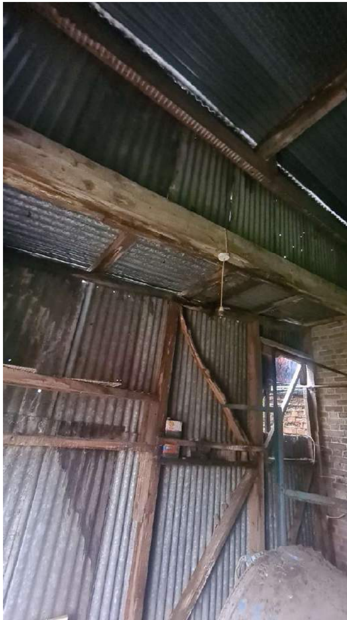
Photograph 37 – Barn C interior roof and wall structure
