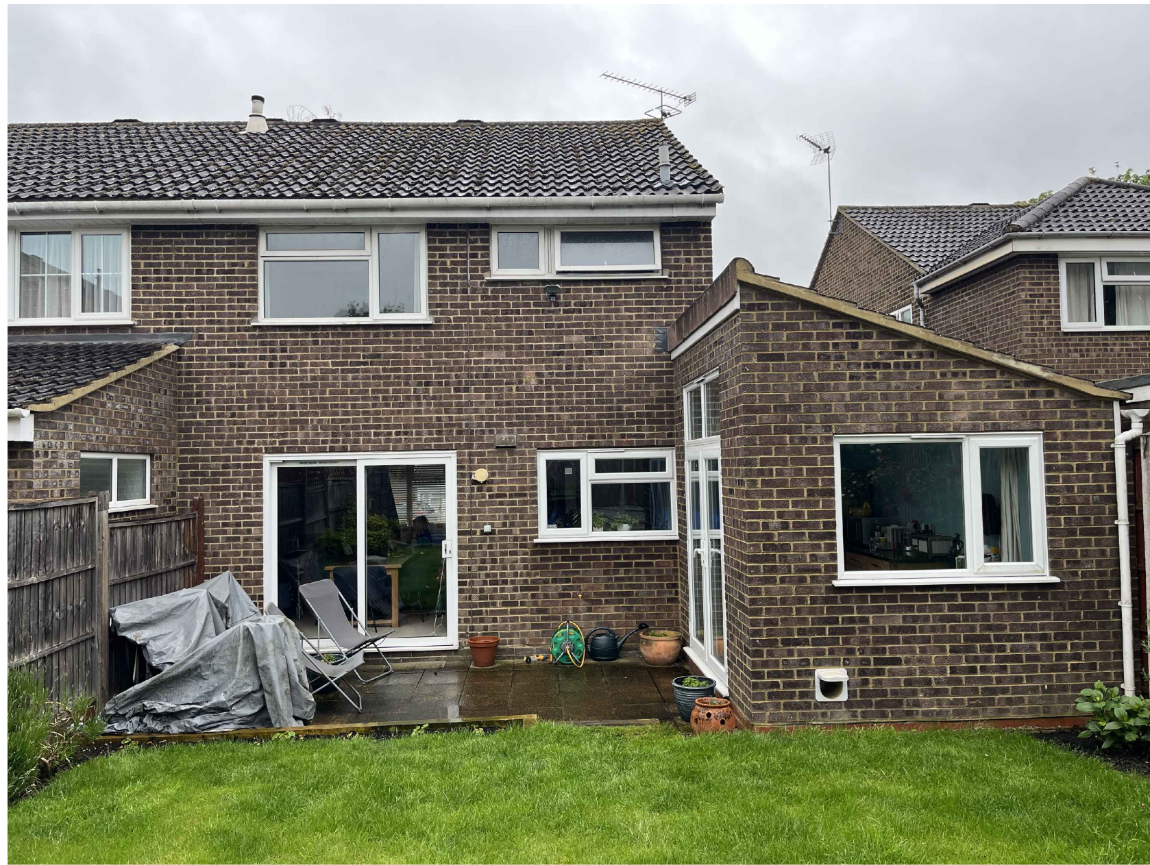
REAR VIEW OF EXISTING PROPERTY
