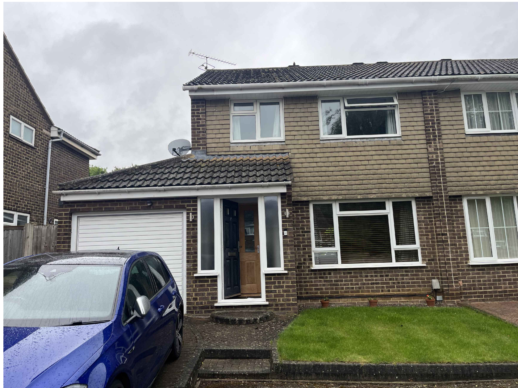
FRONT VIEW OF EXISTING PROPERTY
