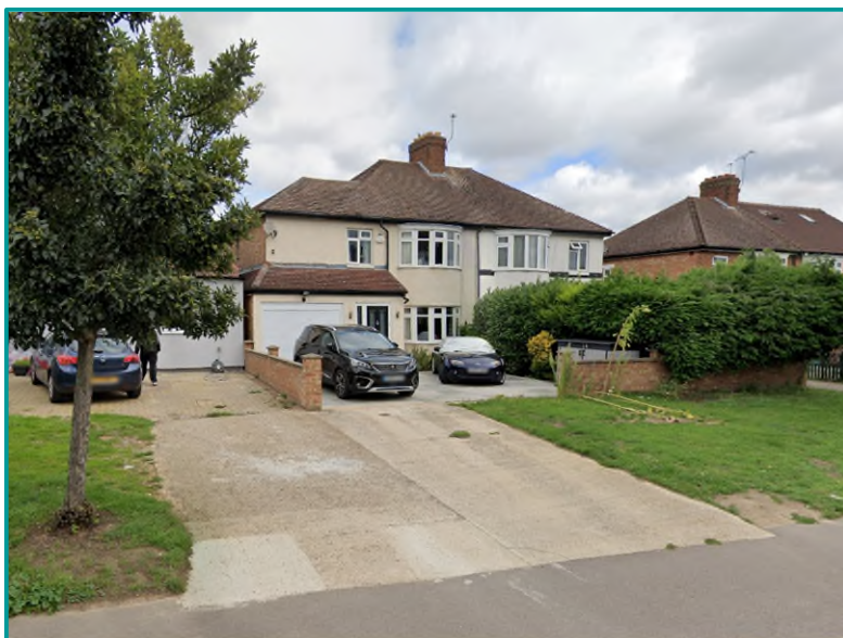
Figure 1 - Pre-existing vehicle crossover (Google Maps, Aug 2020)
