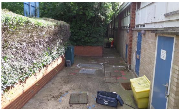
Photograph Three - Northern end of building (toward Glebe Rd).
