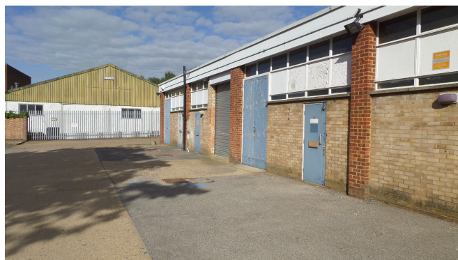
Photograph Four - Parking area to rear of site. Looking west toward neighbouring car repair workshop site.
