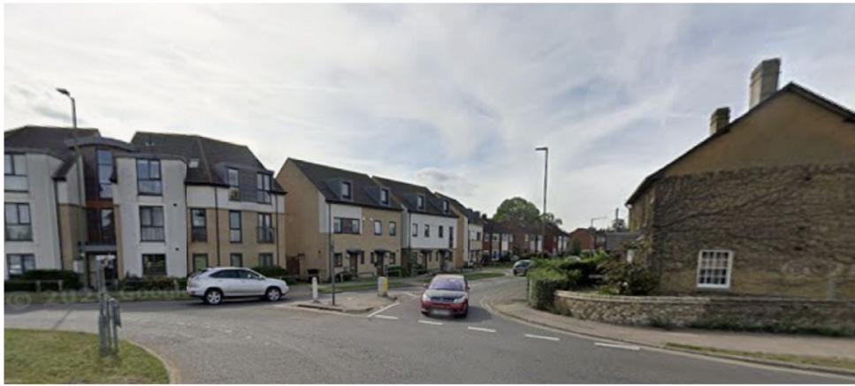
Clothall Road Roundabout Street View
