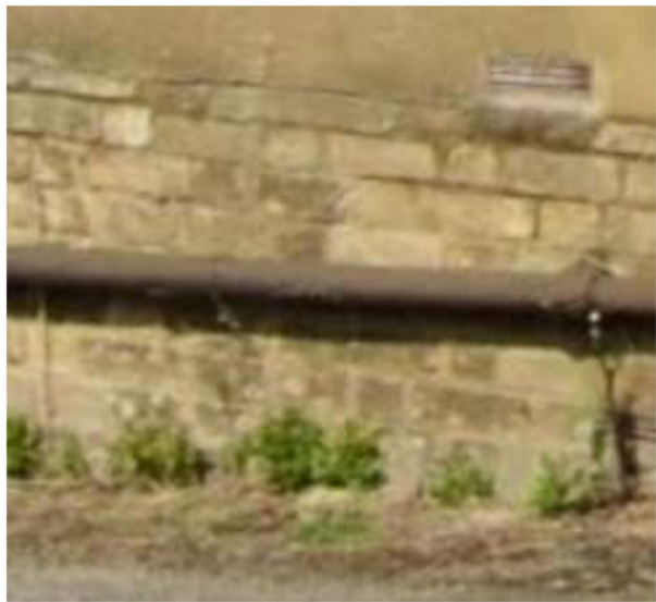
Facing Brickwork: (buff)
