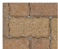
Permeable Block Paving Parking Bays Colour: Bracken
