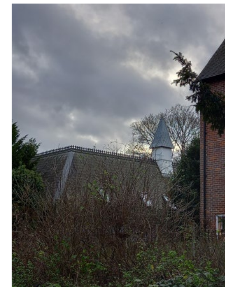
Former stables, rear of Lanterns
