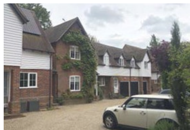
Hunter Mews - Situated North-West of the site
