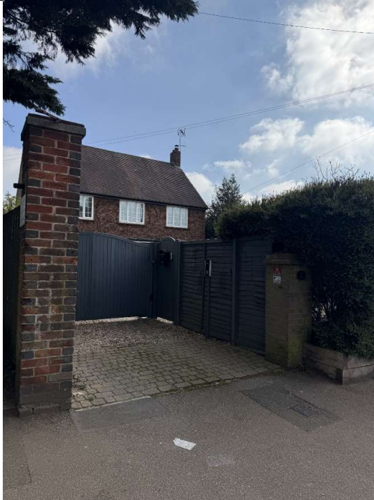
Photo 5: Boundary structure exceeding 1.0m in height adjacent to the footpath, incorporating brick piers and setback vehicular access gate.
