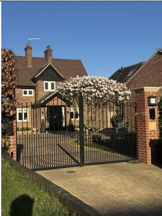
Photo 7: Brick piers exceeding 1.0m in height, together with setback black metal vehicular access gate.
