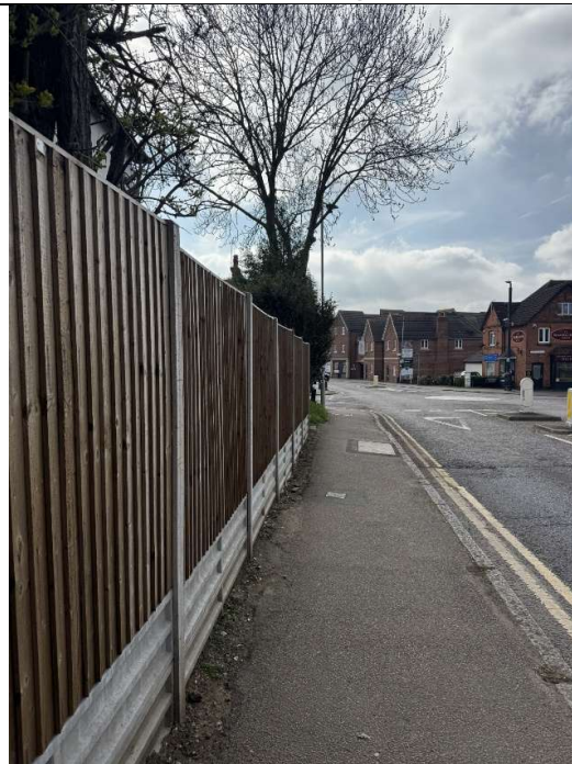
Photo 4: Boundary structure exceeding 1.0m in height positioned directly adjacent to footpath.
