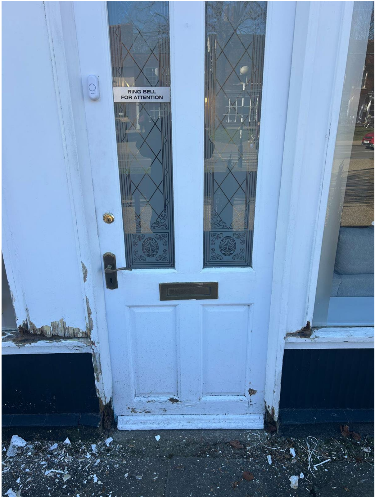
Existing Door Condition.
