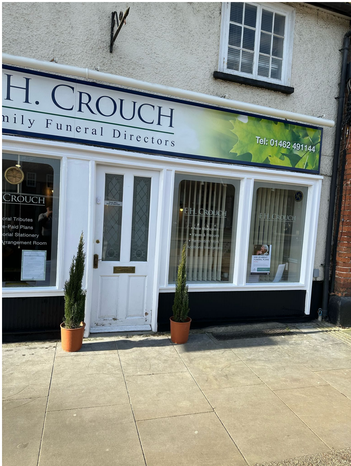
View Front Street – prior not timber rot inspection
