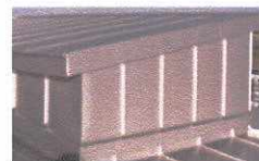
Terne Coat Stainless Steel Standing Seam Roofing & Vertical Cladding
