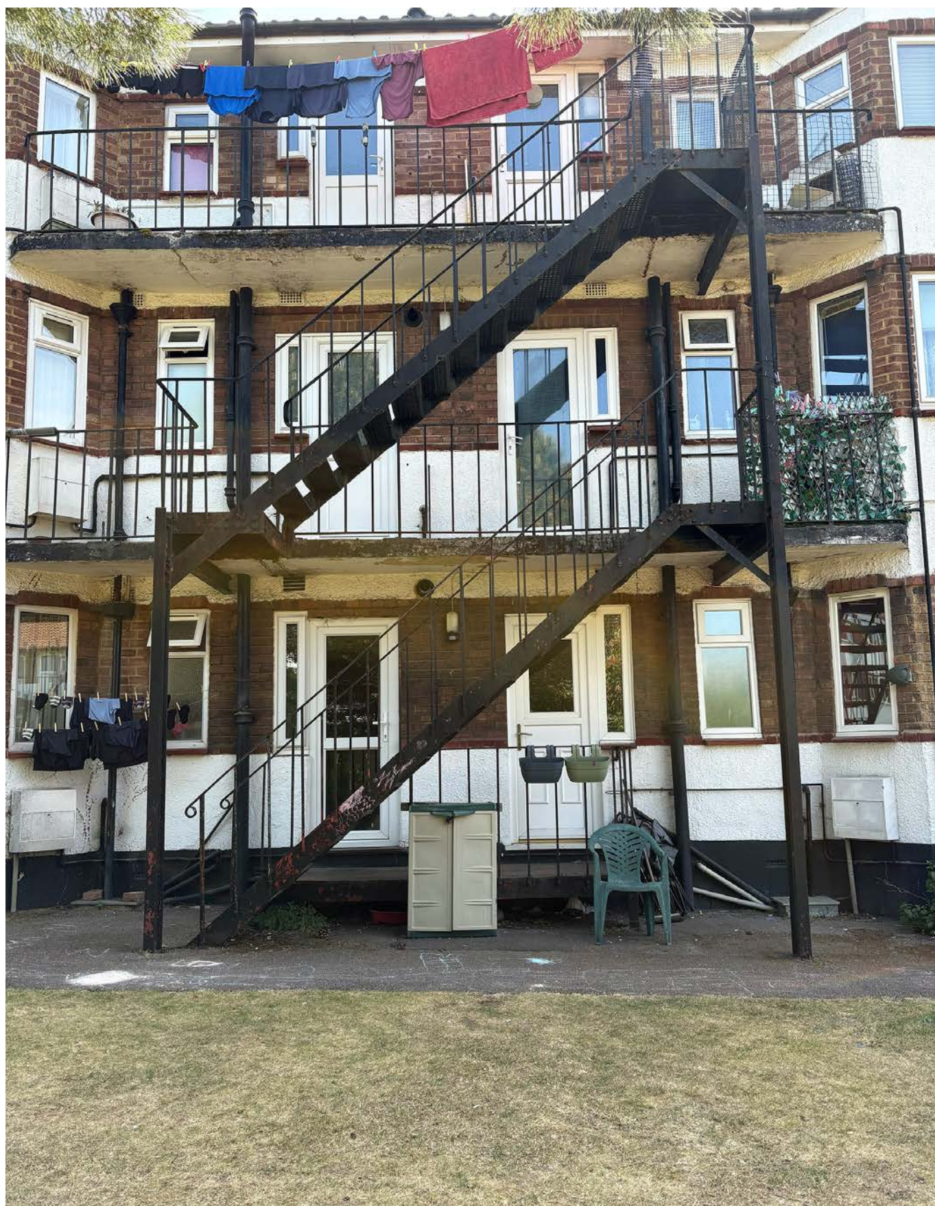
(008 – Staircase 4 and balconies existing condition)
