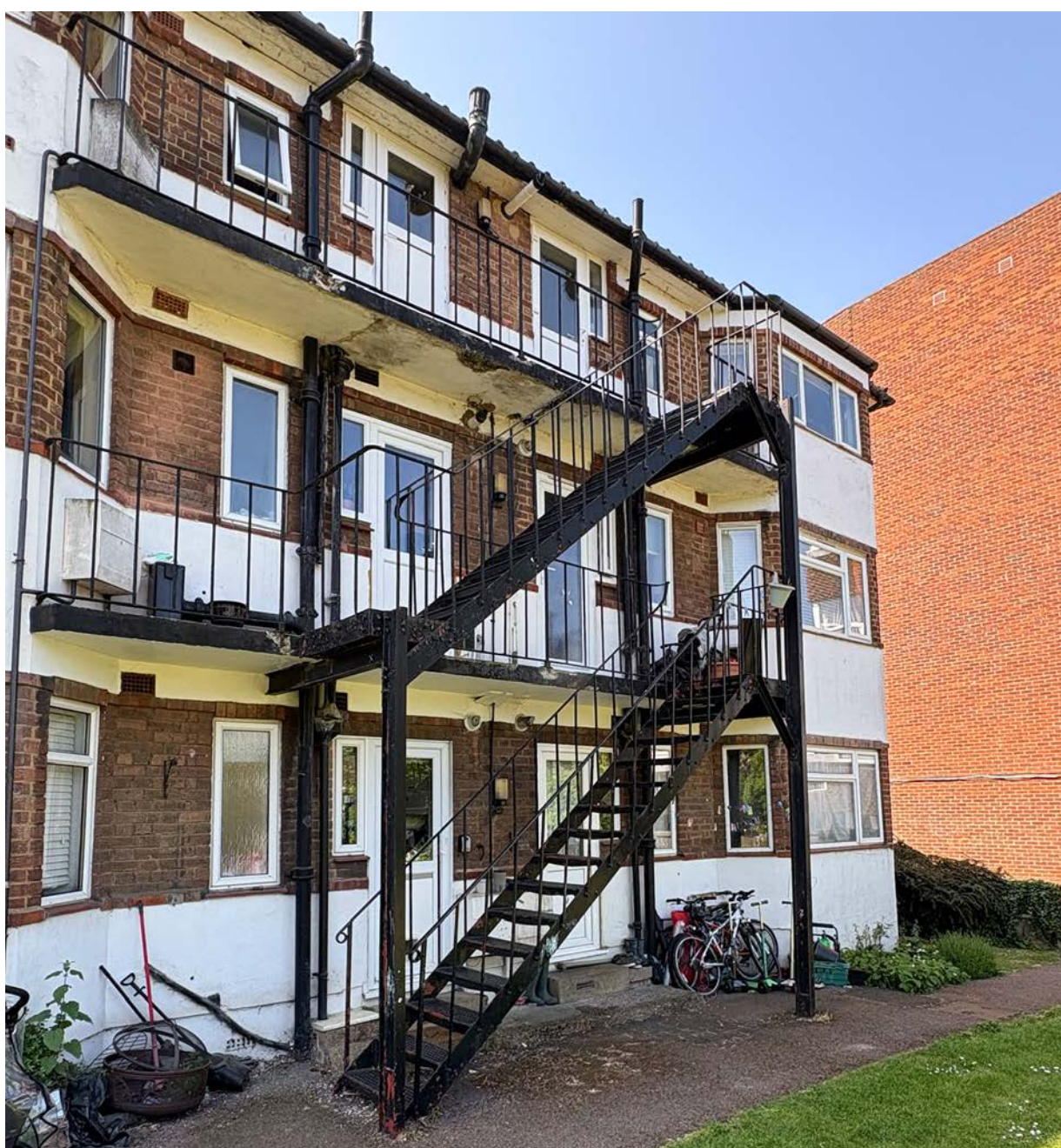
(005 – Staircase 1 and balustrading – existing condition)
