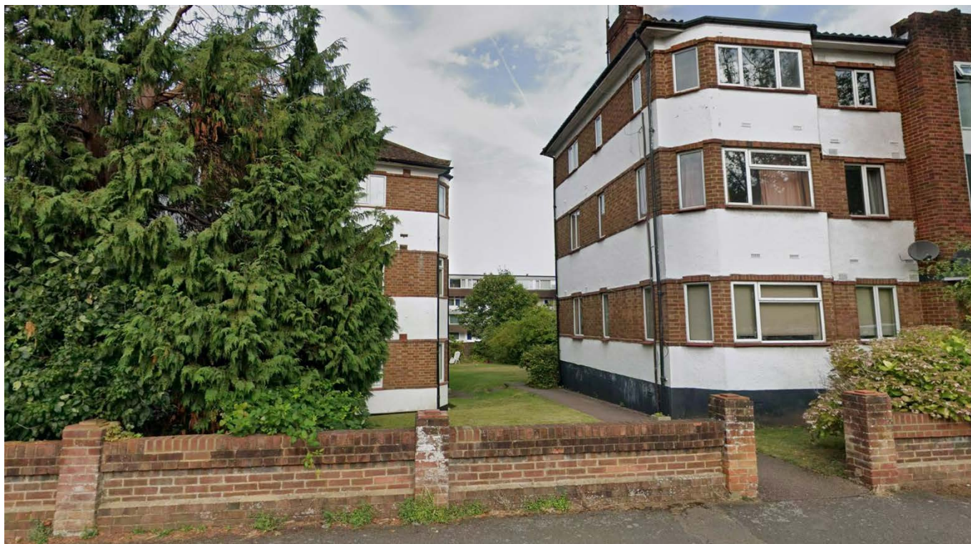
(002 – Street view - gap between blocks near corner junction)
