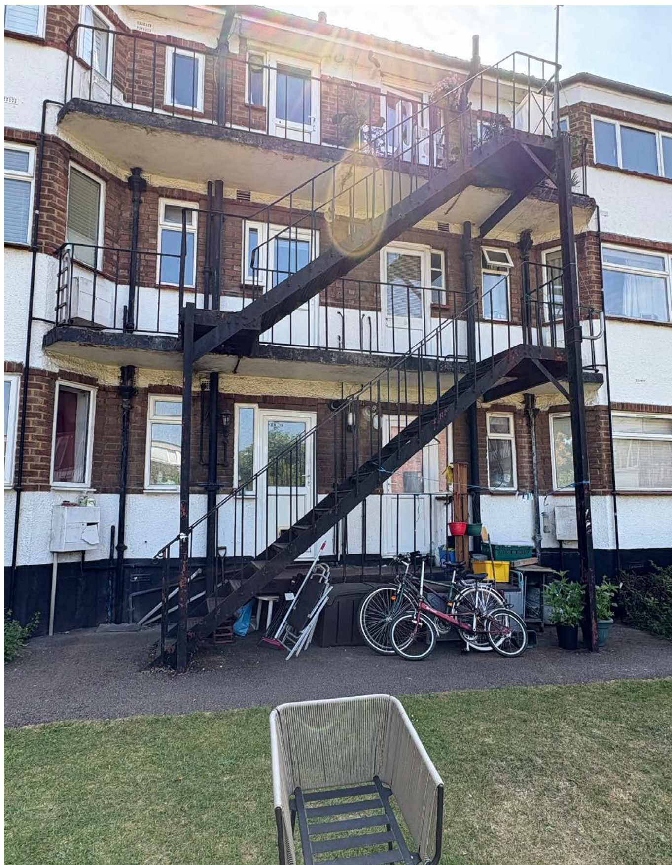
(007 – Staircase 3 and balconies existing condition)
