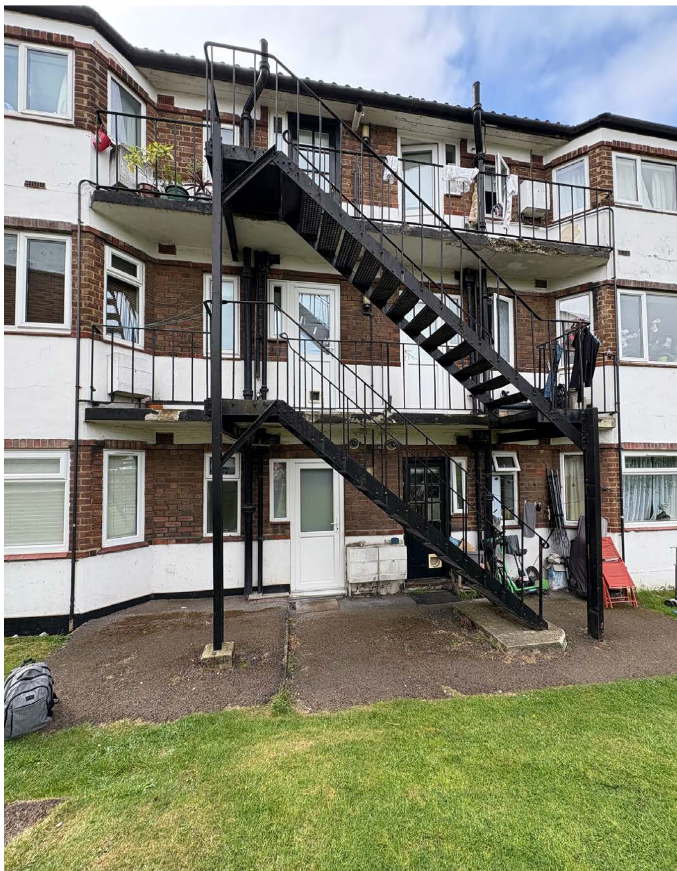
(006 – Staircase 2 and balustrading existing condition)
