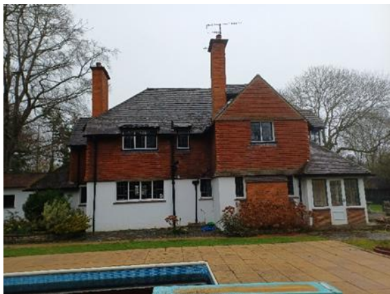
Rear house elevation
