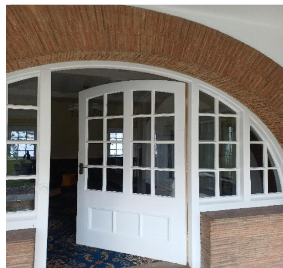
Aluminium patio sliding doors removed to expose existing Verandah door & brick sweeping arch
