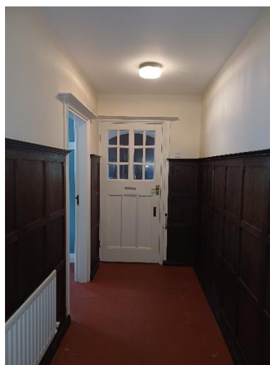
Original front entrance door
