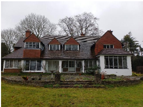
Full height glazing to Dining and aluminium sliding doors to verandah removed.
