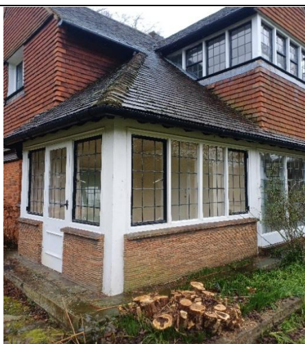
2. Door/windows/tiled wall removed to expose open canopy
