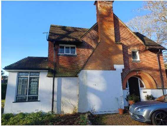
GF Lounge extension removed
