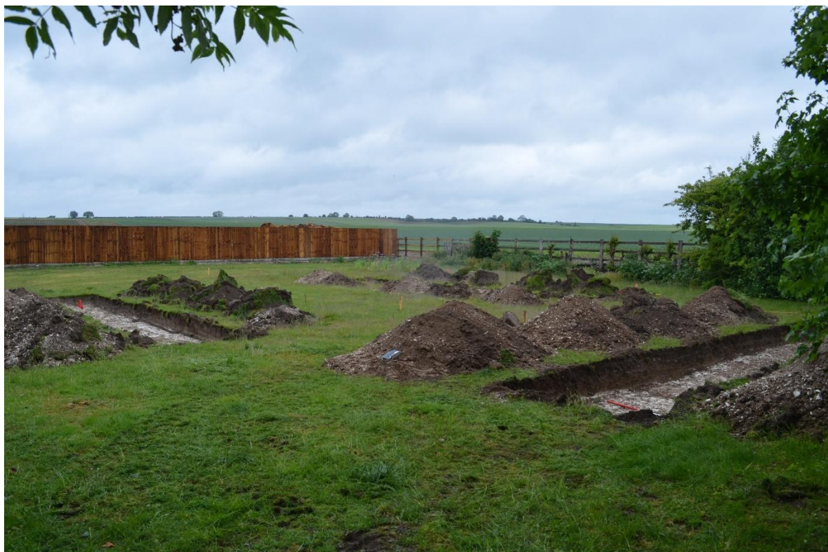
Plate 1: Trenches 1-3, view north.
