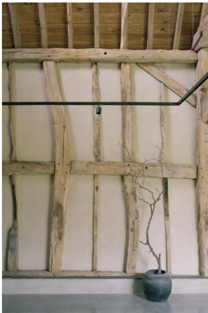
Exposing and insulating existing structure. Hunts Green Barn by McLaren Excell
