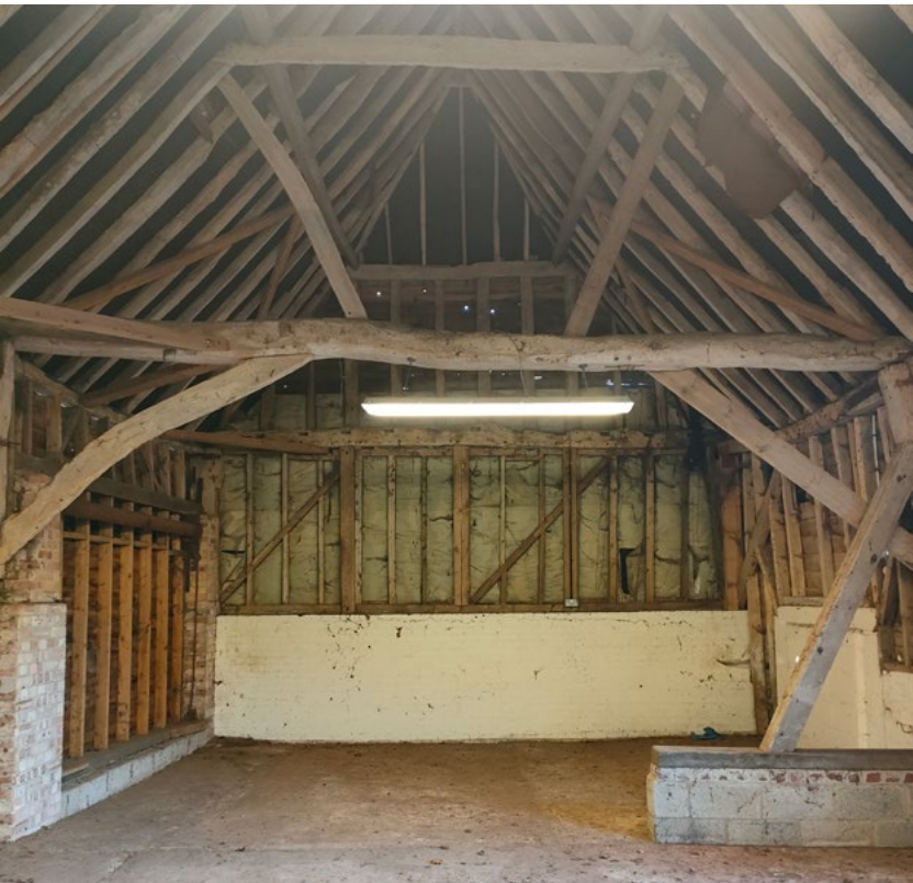
Existing view of bay 7
