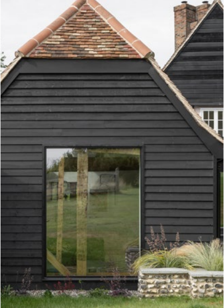
Exposed historic structure within window openings at Holborn Farmhouse. By Will Gamble Architects
