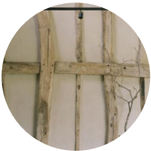
Sandblasted and treated Timber
