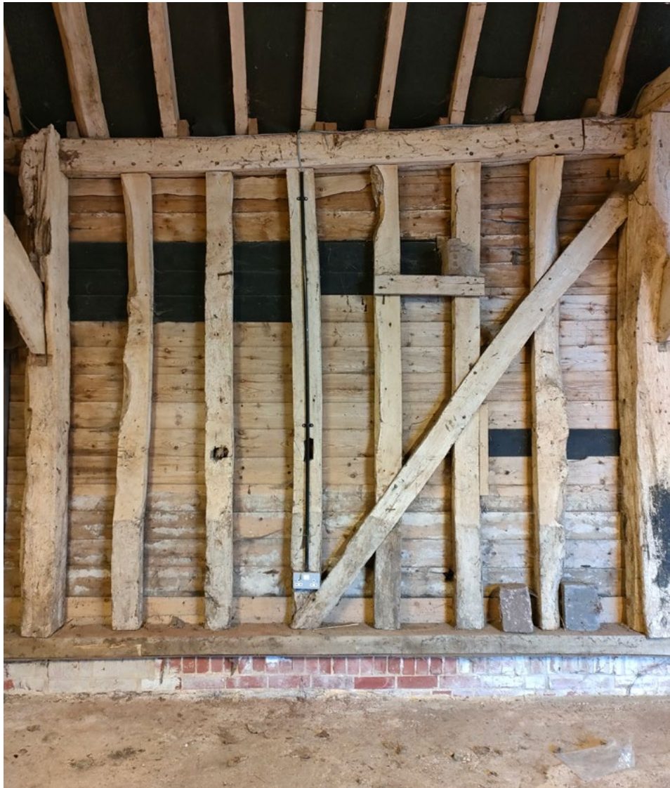
Internal view of bay 2 (south elevation), Holborn Barn
