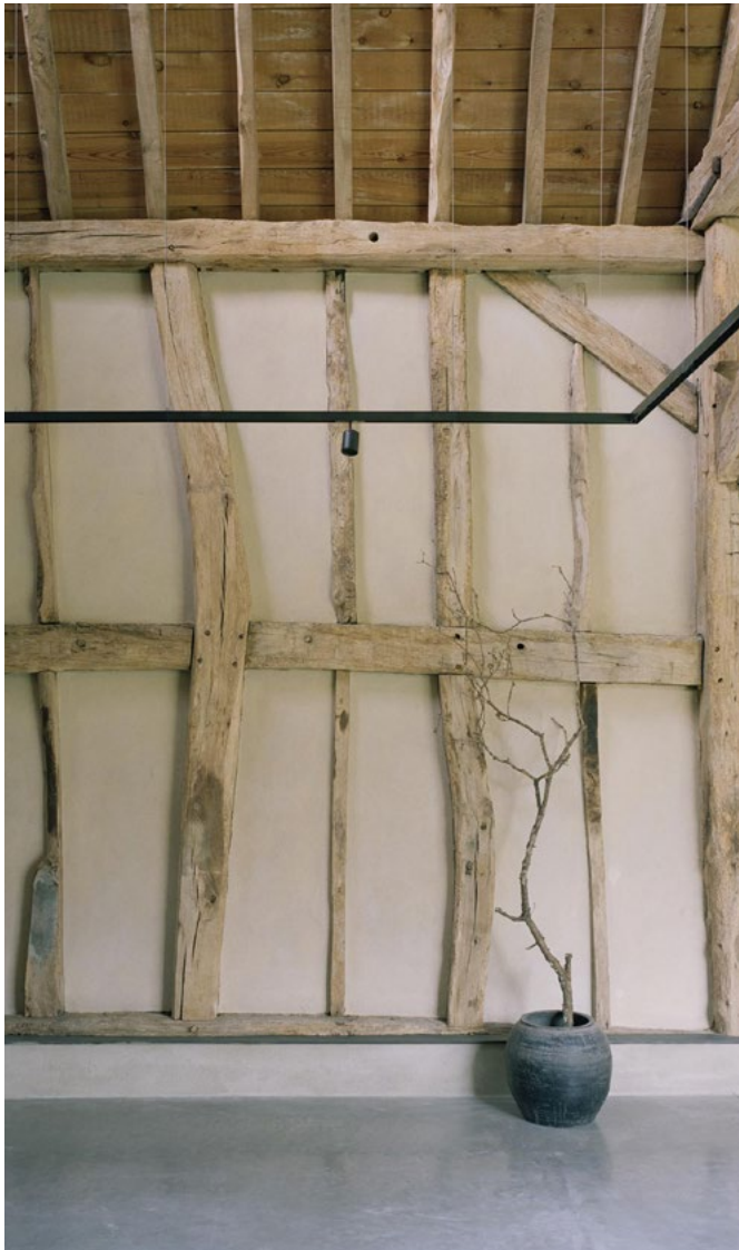
Exposing and insulating existing structure. Hunts Green Barn by McLaren Excell
