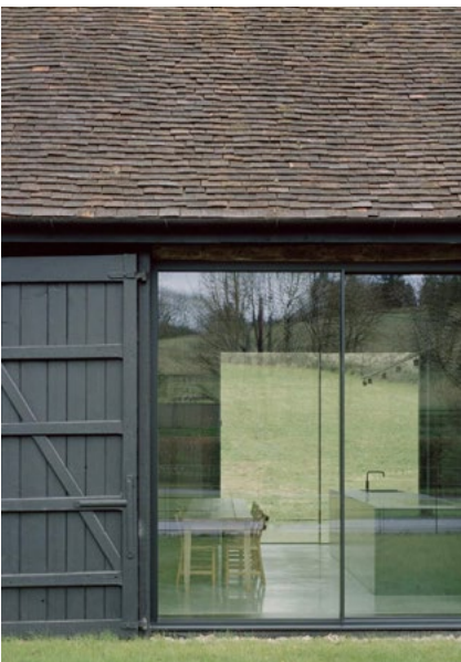
Large openings concealed by shutter style barn doors. Hunts Green Barn by McLaren Excell
