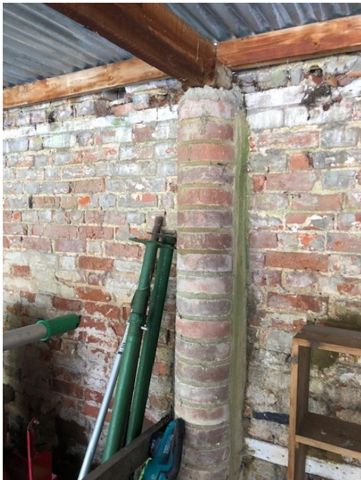
Photo – 2: Rear Wall Internally with Small Pier
