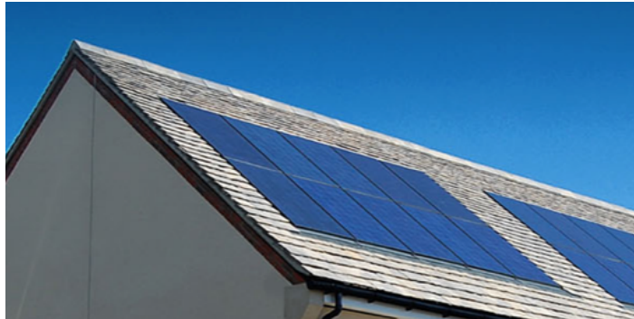
Figure 9: Typical PV installation to pitched roof
