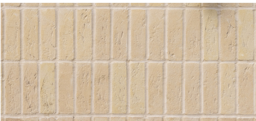
Stack bonded brick detail
